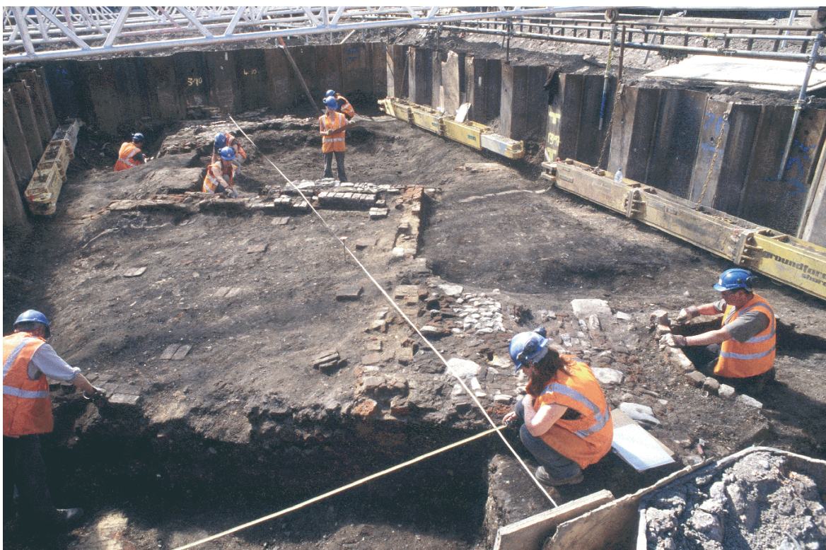
Fig. 10: in the foreground is an outbuilding of the Earls of Rutland’s mansion (facing west)
