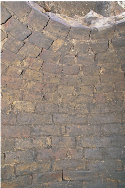
Fig. 3: inside view of the wall and domed top
