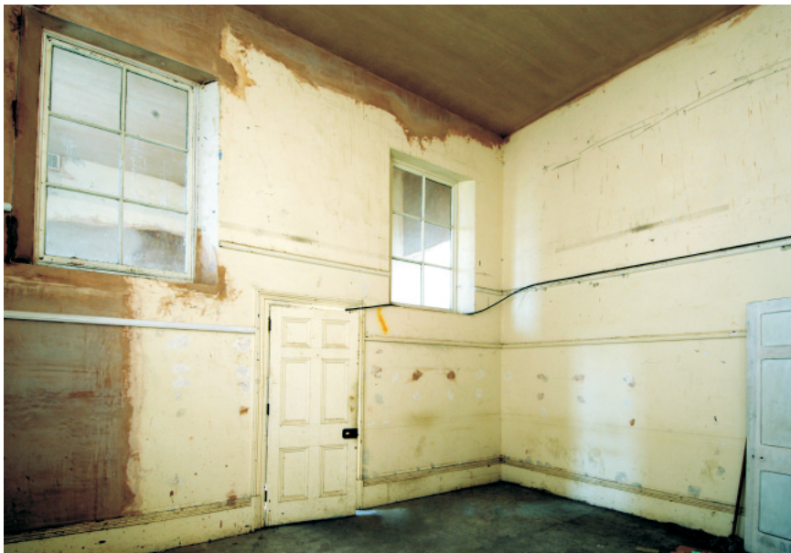
Fig. 13: the south wall of the 1st-class ladies waiting room, showing the thicker wall with revealed windows, possibly a former external wall to the original 1854 station
