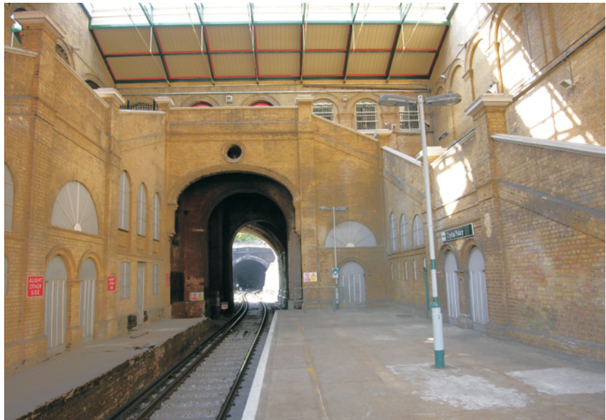
Fig. 5: the northernmost platform in the train shed, looking west; the tunnel passes below the entrance building and areas below the stairs provided gentlemen's lavatories and storage space
