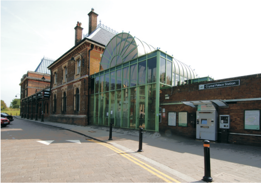
Fig. 3: the station entrance building, with the 1980s 'birdcage', looking north
