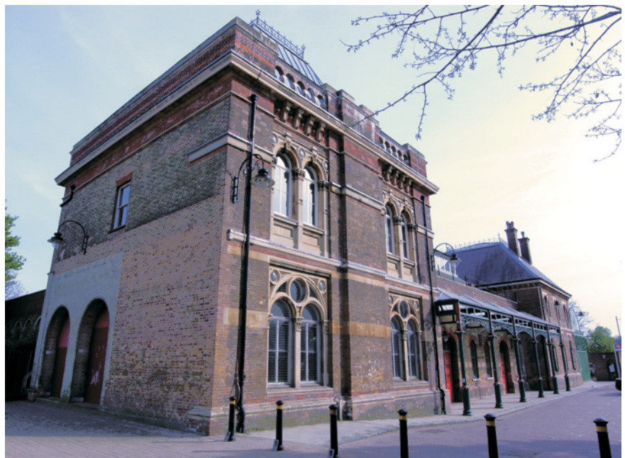
Fig. 9: the station entrance building, looking south east, with the north pavilion in the foreground
