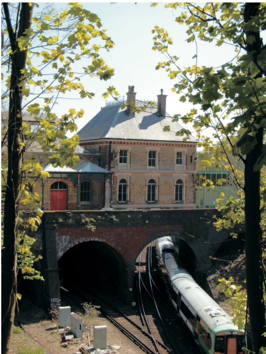
Fig. 6: the station from the west, showing the tunnel beneath and the line to Wandsworth
