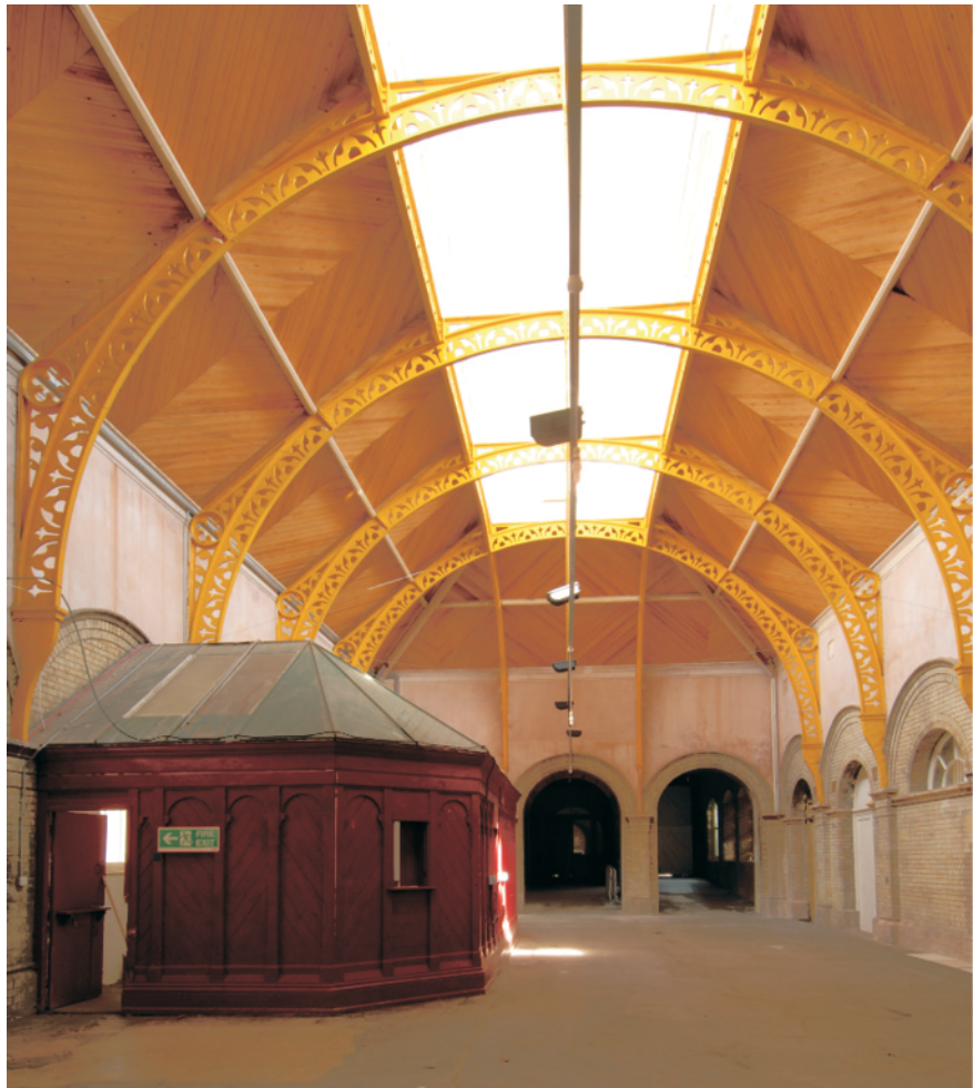
Fig. 12: the ticket booth and hall with ornate arched roof beams, looking north
