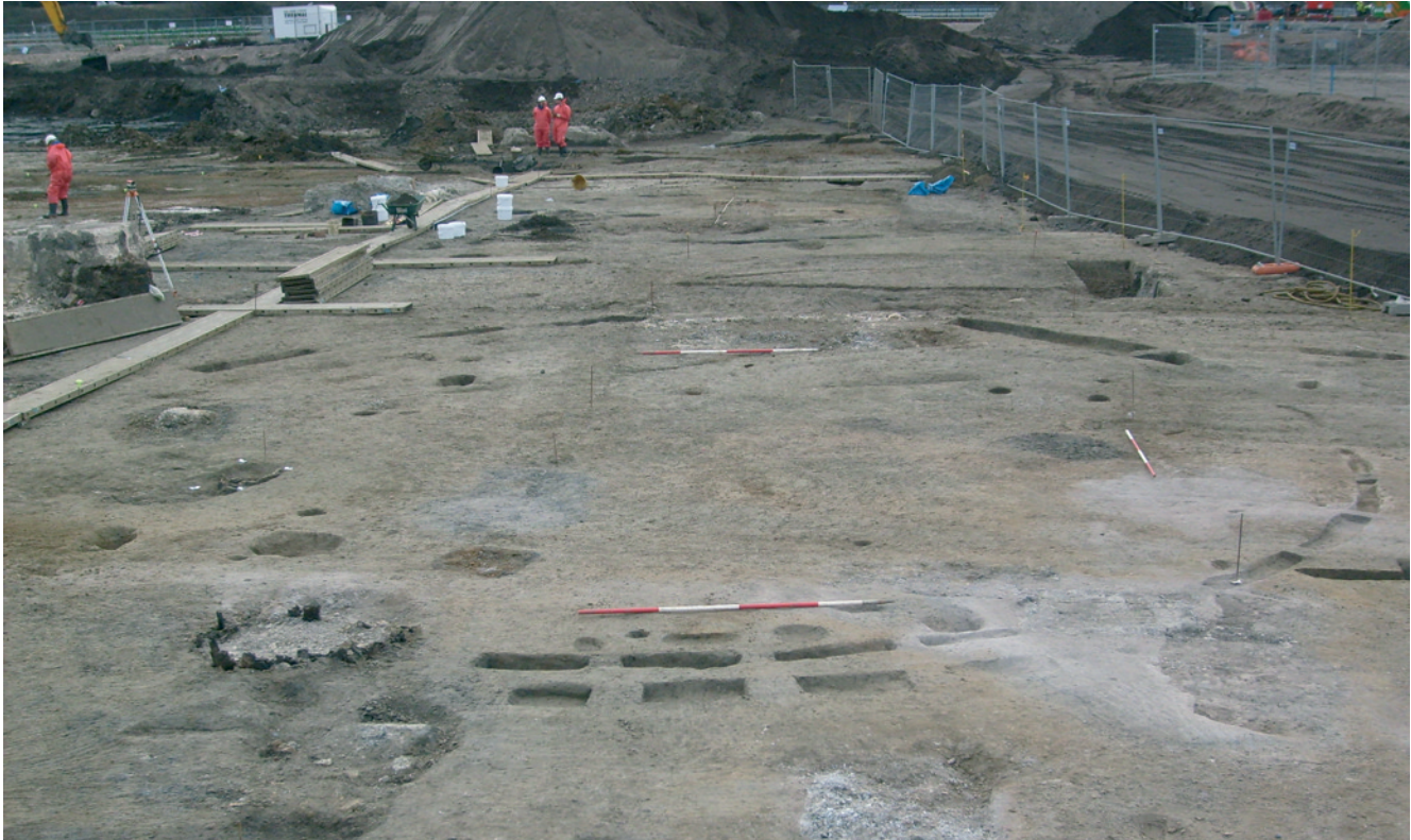
Fig. 5: general view of site, showing Middle Iron Age ring gully and re-cut (© MoLAS-PCA)
