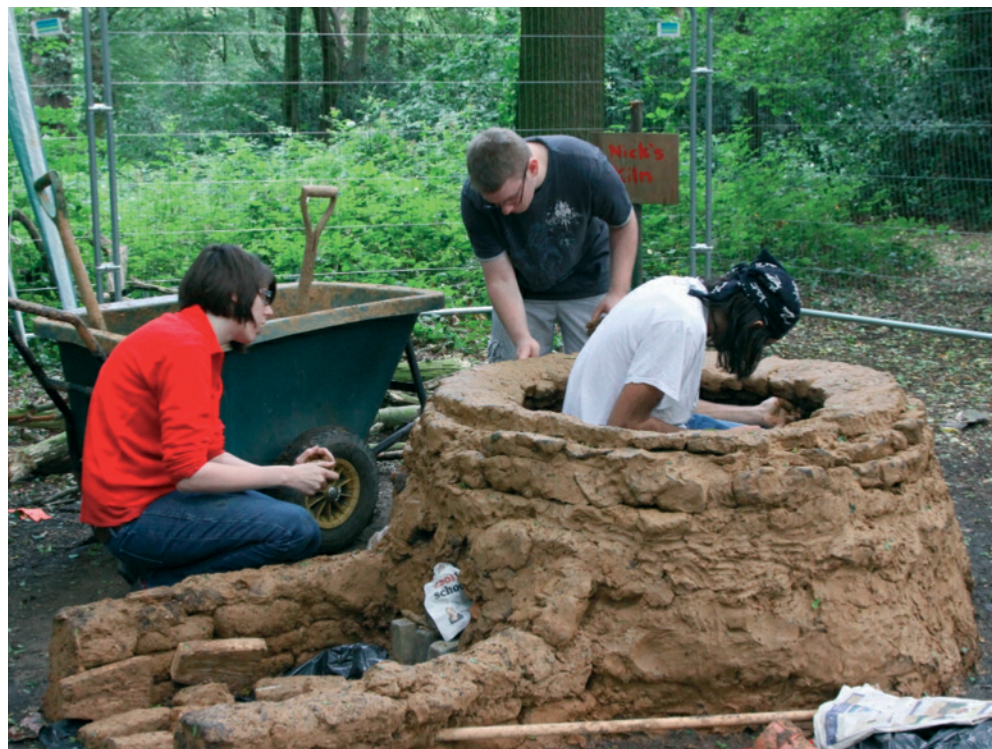
Fig. 3: Jennifer, Tom and Mathew building the kiln. This is the first attempt and the kiln was soon to suffer a partial collapse due to excess water in the clay. (Photograph: Bruce Castle Museum, Haringey Cultures, Libraries and Learning)
