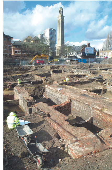
Fig. 5: late-18th-century barrel vaulted cellar, with 19th-century malthouse and engine house to rear. Kew pumping station tower in background. View from south-east.
