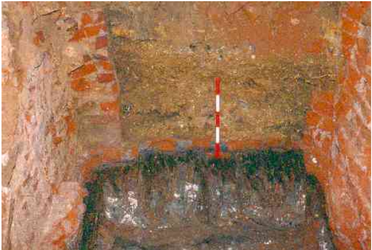
Fig 55 Exposed oak plank foundation [48] below the eastern end of the wheel housing [47]. Immediately behind the 0.5m scale and below the present Mill wall is the infilled millrace
