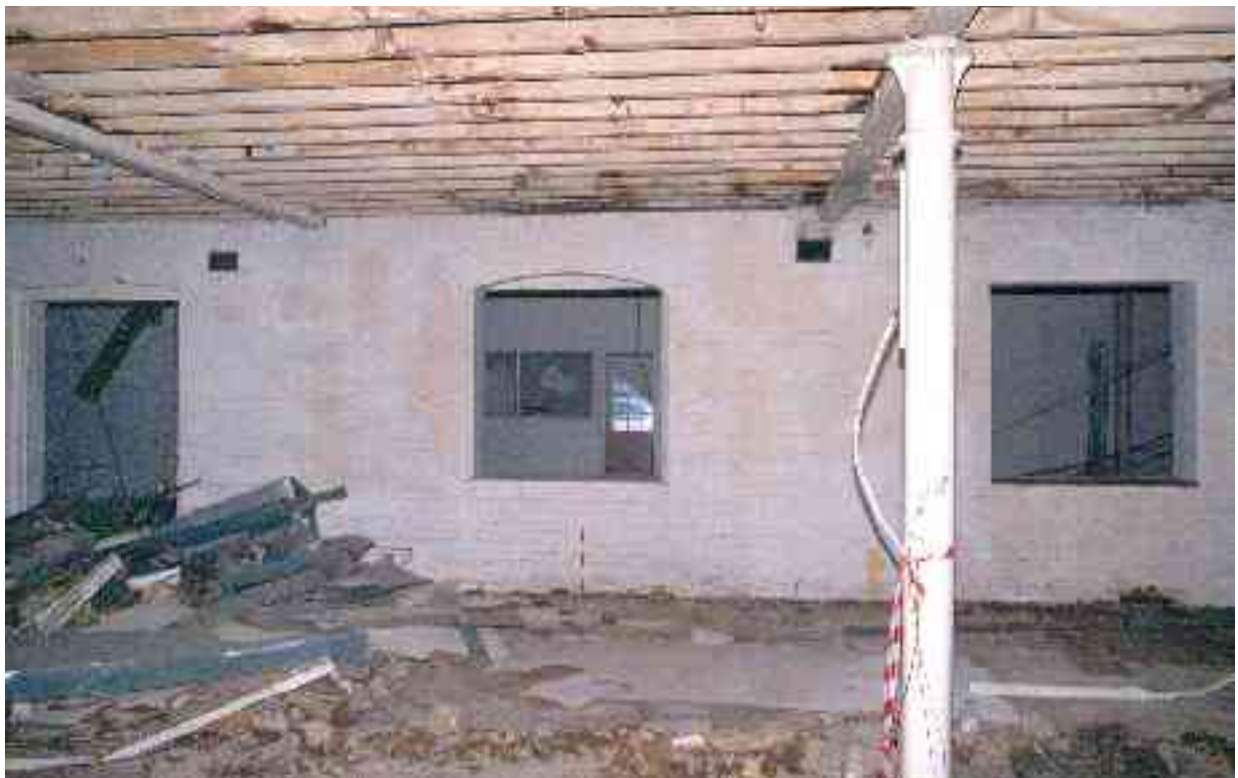
Fig 12 The internal face of the 1860s west front of Grove Mill (the same area as in Fig 7 but viewed from the inside). Note the variation in window/door head design (l-r) from shallow to fuller arch to flat, reflecting the original layout as door, window and blind window
