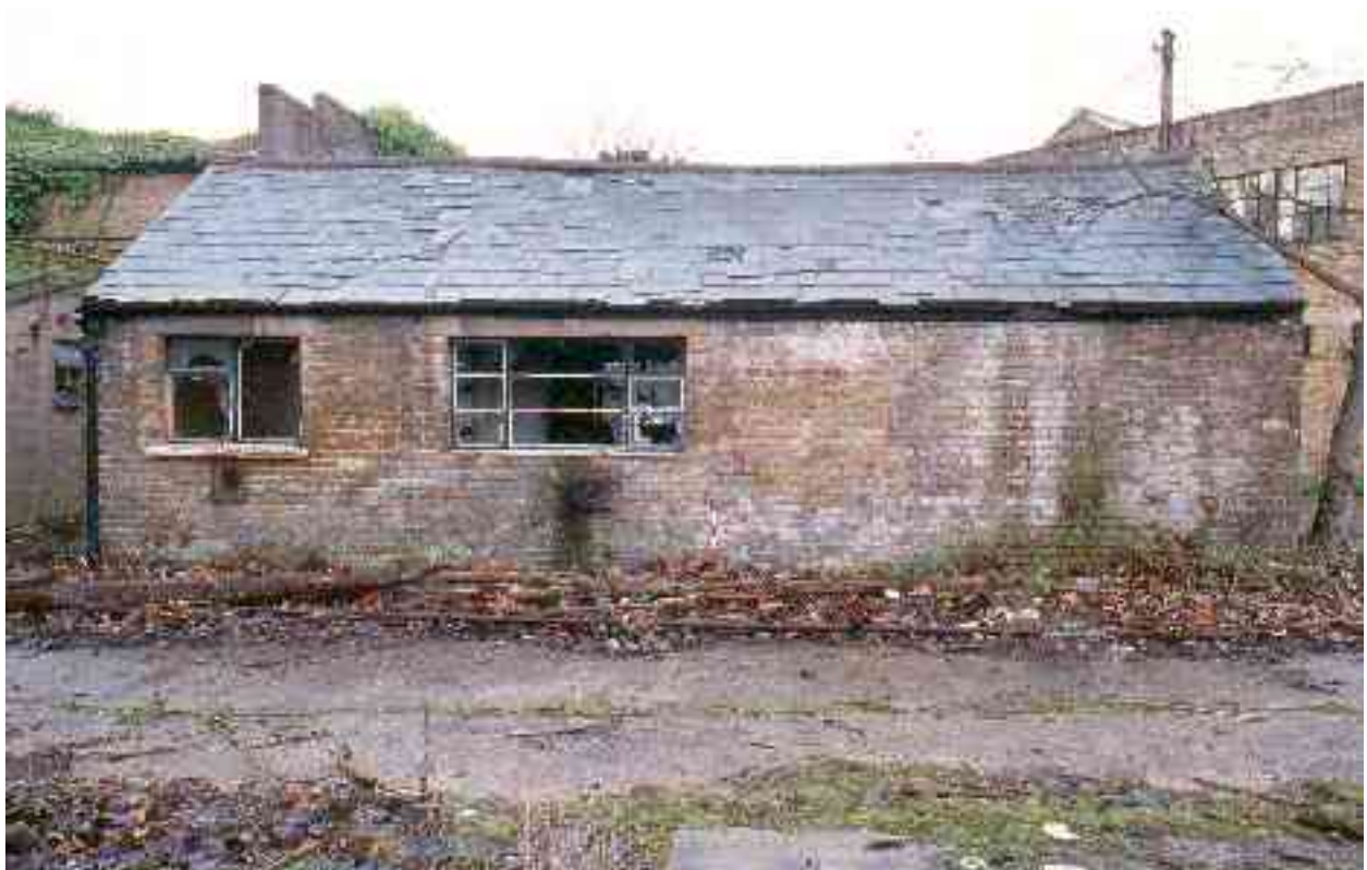
Fig 28 The eastern side of Building C, again showing later window insertions with concrete lintels and a blocked arched opening immediately to the right of the 0.5m scale. This wall previously fronted onto an open north-south channel
