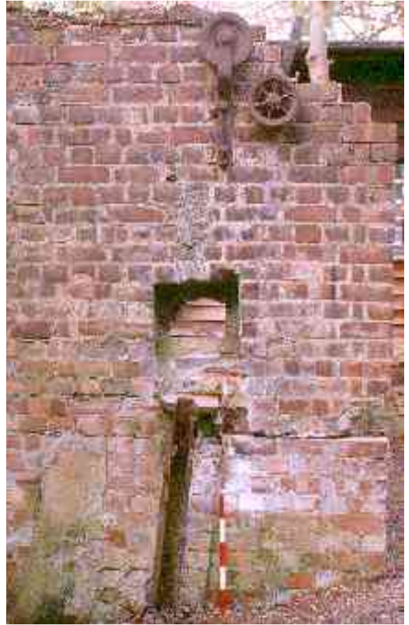
Fig 22 Remains of the sluice, including a cast iron channel for the gate
