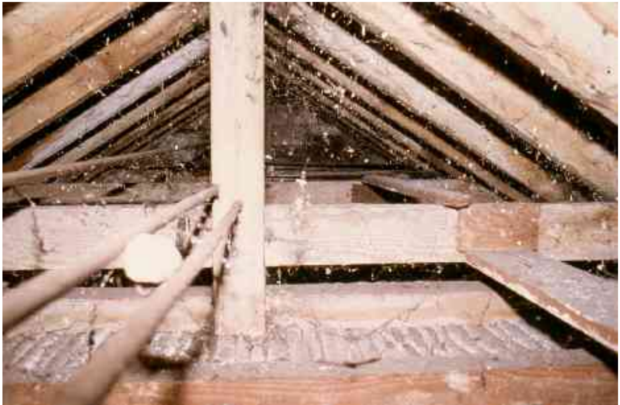
Fig 29 The roof construction of Building C, looking north. White paintwork is visible on several of the timbers, with a later lathe-and-plaster ceiling in the foreground
