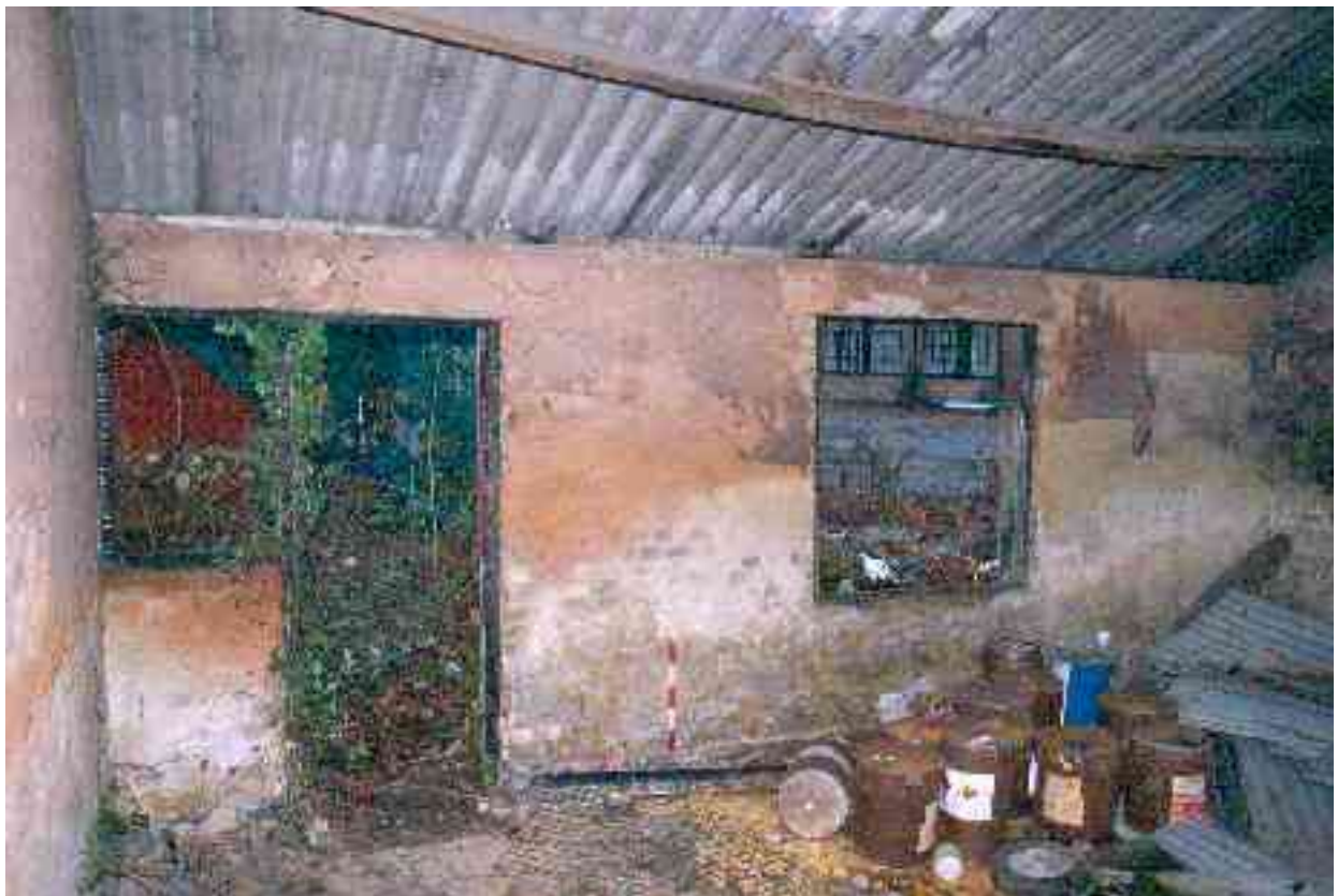
Fig 26 Interior of Building B, looking towards the west face and showing the minimal structure of the replacement roof
