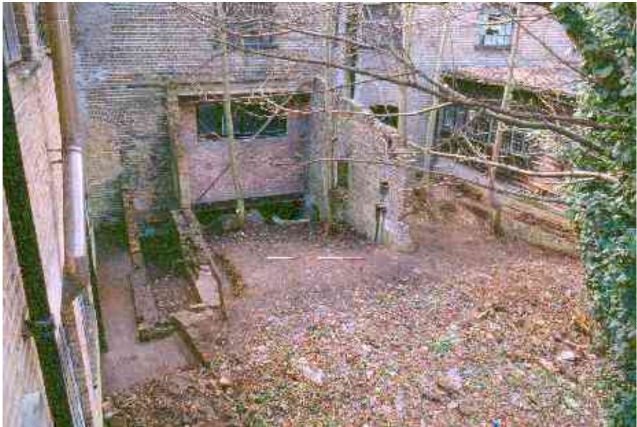
Fig 16 The remains of the wheelhouse and machine pit, looking west towards the earlier part of Grove Mill (2m scale). The central red brick blocking wall and window are also of 20 th century date
