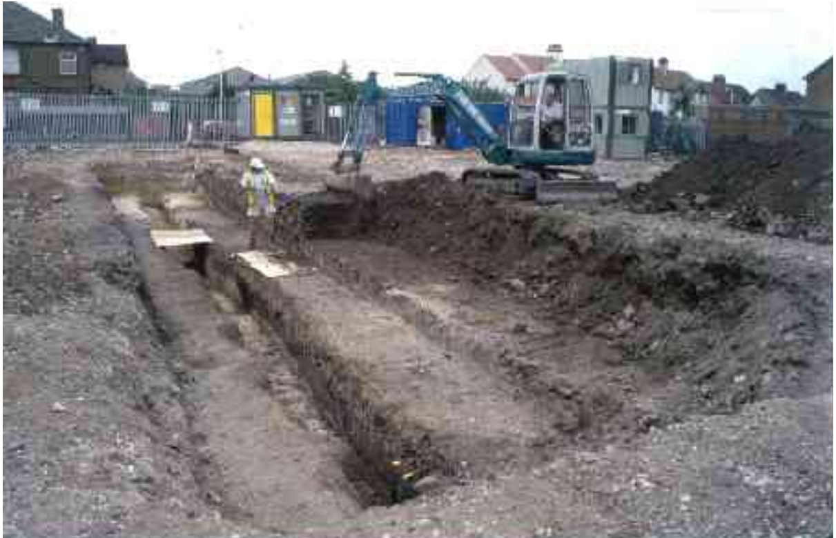
Fig 16 View showing an earthmoving machine extending the north-east side of the evaluation trench. This was done for safety reasons so as to reduce the height of the ground surface in the area of the archaeological excavation
