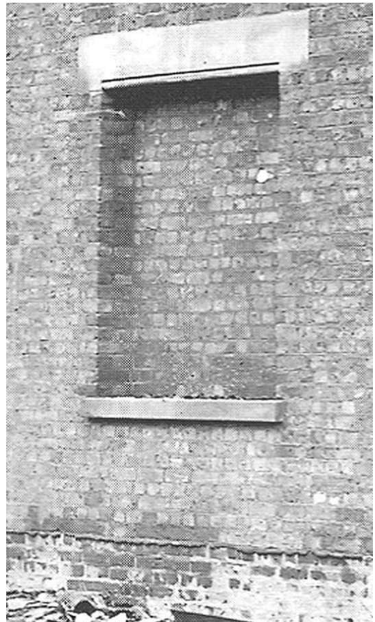
Fig 11 Ground floor opening within the west face of the 1860s Grove Mill, prior to redevelopment (left) and as a blind window immediately after the 1907 fire ( see also Figs 7 & 8 )
