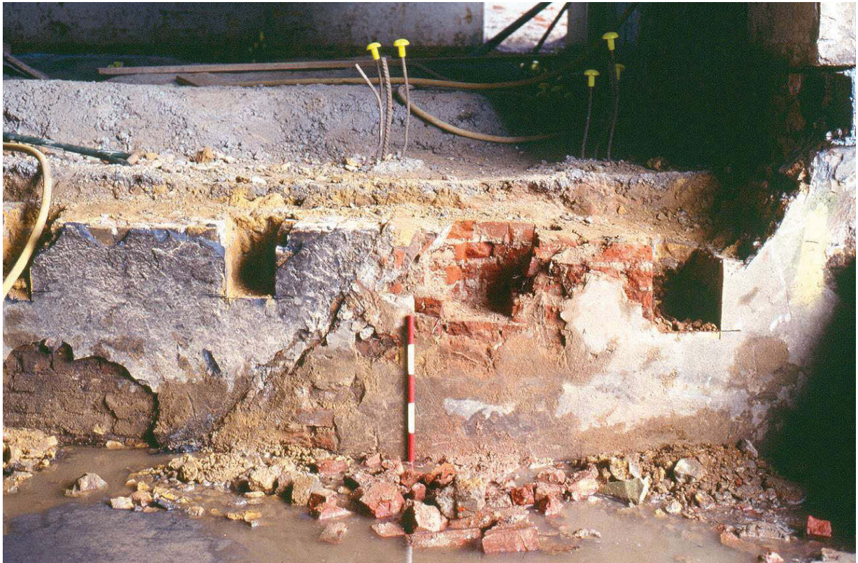
Fig 54 The truncated southern side of the red brick structure [47], incorporated into the 1860s yellow stock wall [33]. The line of the earlier waterwheel is visible just to the left of the 0.5m scale
