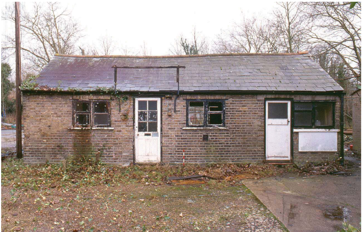
Fig 27 The western side of the 19 th century Building C (0.5m scale). The two door openings are original but the central window has been widened and those at either end are later insertions. The frame over the left-hand door previously held the sign Mitcham Hair & Fibre Mills
