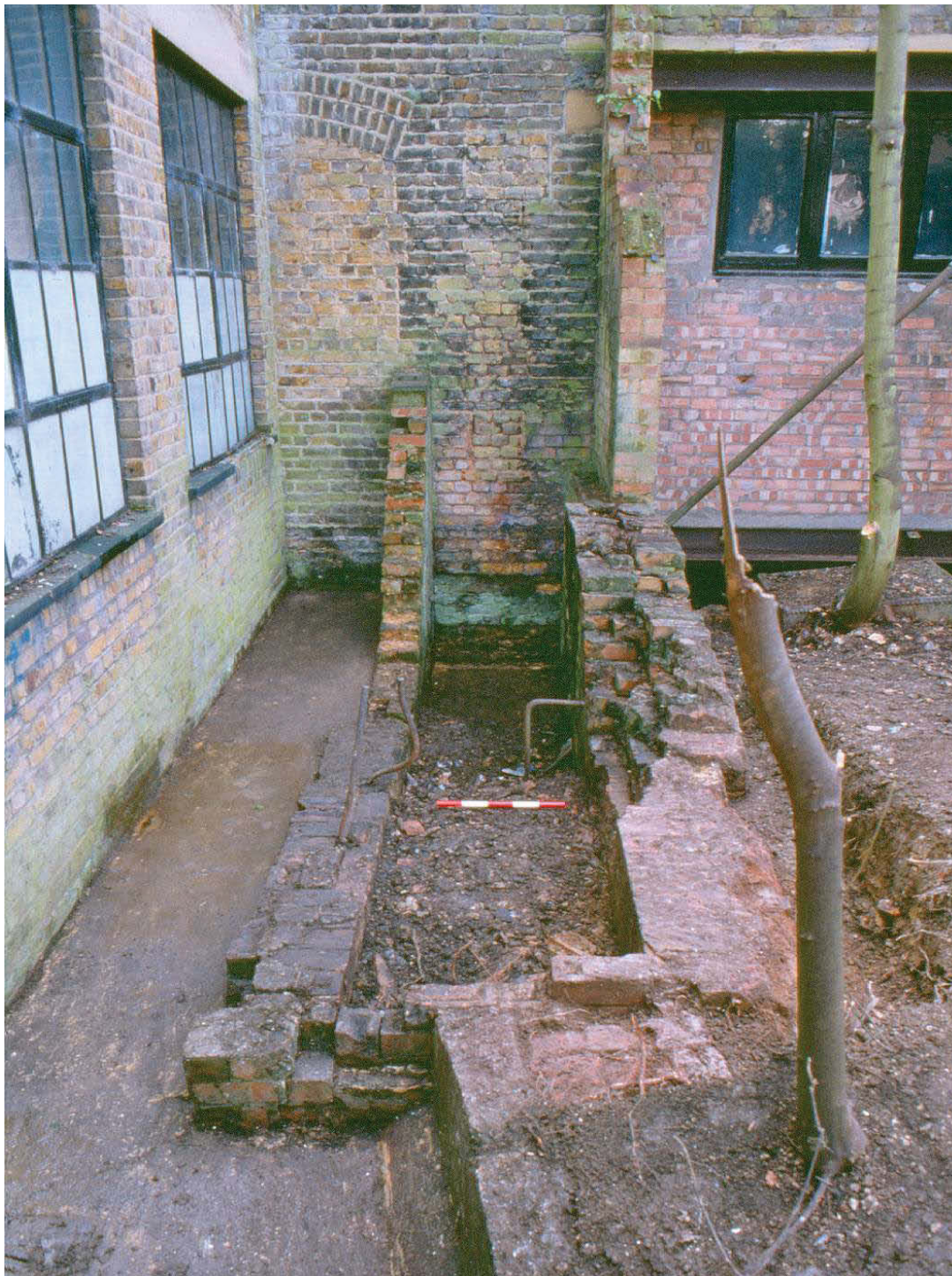
Fig 24 Machine pit on the southern side of the waterwheel ( 0.5m scale; see Figs 14 & 17 ). The 19 th century mill wall in the background has a blocked window to the left and smaller areas of blocking above the pit that would have taken the drive shaft from waterwheel
