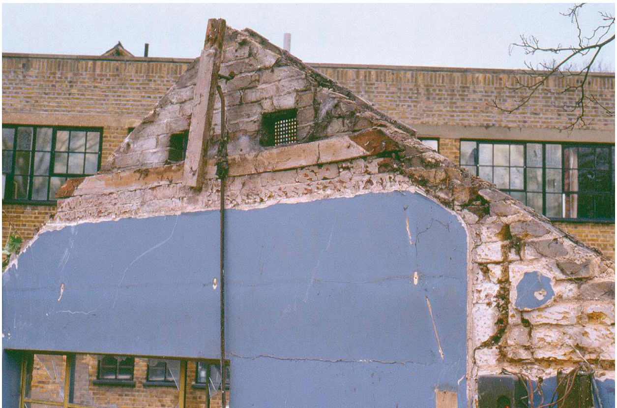
Fig 30 The northern gable end of Building C during demolition. This internal view shows the original full-height limewashed brick face, subsequently obscured by plasterwork and ceilings
