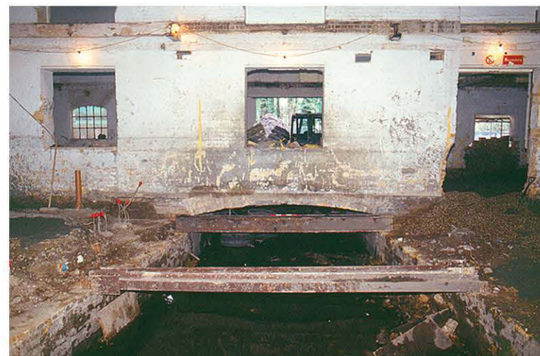
Fig 7 Elevation and views of the west face of the 1860s Grove Mill, now forming the central wall within the extended building. The photo at lower left shows the exposed millrace after removal of the floor slab
