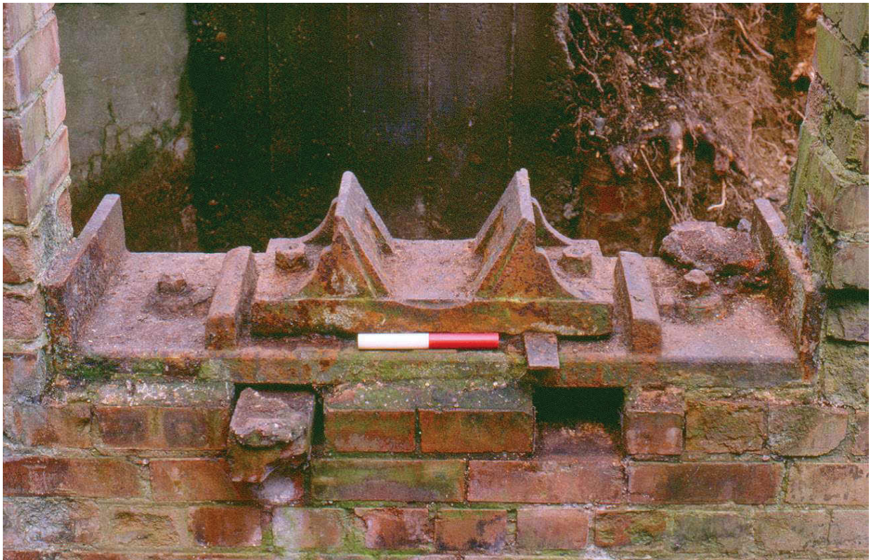
Fig 23 Cast iron bracket or plummer-block for the northern end of the waterwheel axle. A levelling bar for fine adjustment projects just to the right of the 0.2m scale
