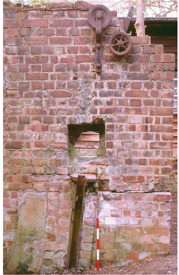
Fig 22 Remains of the sluice, including a cast iron channel for the gate
