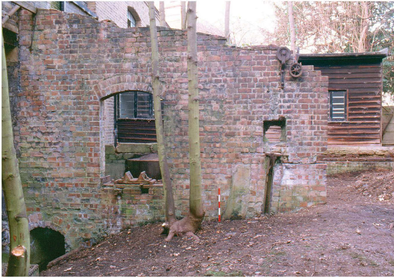
Fig 19 The northern side of the wheelhouse, partially infilled in the 1960s (0.5m scale)
