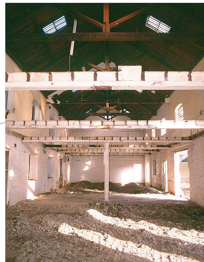
Fig 10 Section across the 19 th and early 20 th century parts of Grove Mill ( elements 1 & 2, Fig 4; located on Fig 5 ) and views during redevelopment works. The lower right hand view shows the main body of the 1860s Mill after removal of the ground slab and first floor. Both sections of roof are contemporary (c 1907/8), using the form of king-post construction known as renaissance truss
