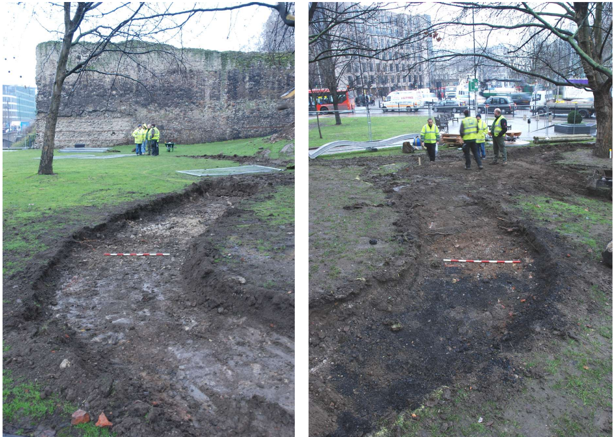
Figure 17 View of path groundworks (No. 5) on the eastern side of the new play area, in both cases approximately 200-250mm deep ( 1m scale ).
