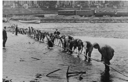
The laying of a cable in the River Esk © Sutcliffe Gallery ( www.sutcliffe-gallery.co.uk )
