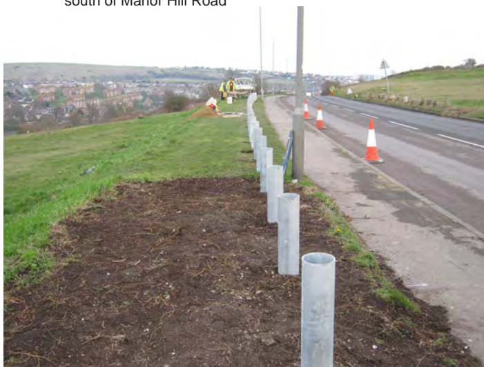
Fig. 4.3: Installation of new bollards, facing west
