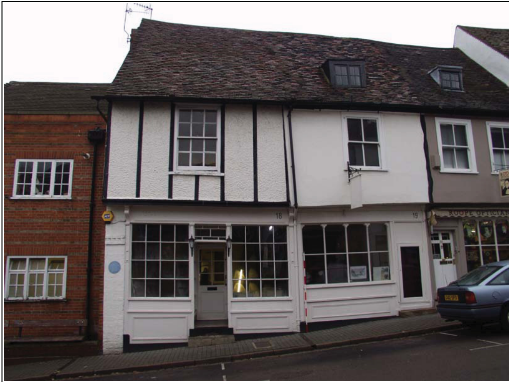
Plate 1 Front/south elevation taken from the S (DP 2)
