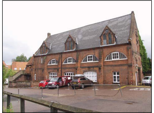
DP 2 South-west elevation of the assessment building, taken from the south-west
