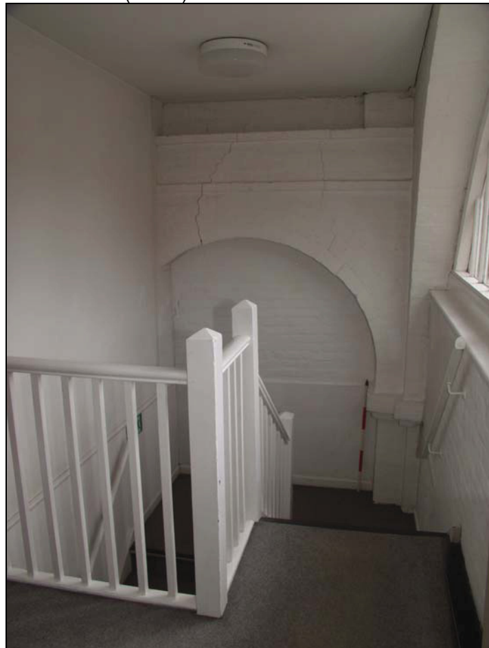
Plate 6 Staircase at upper level (south-east end), taken from the north (DP 28)
