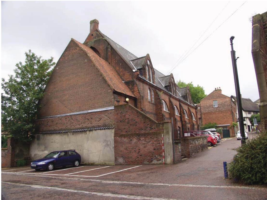
Plate 3 North-west end of the assessment building, taken from the north-west (DP 04)
