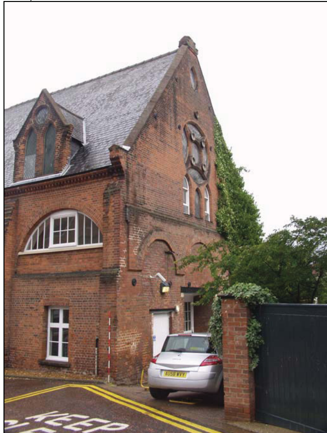
Plate 2 South-east elevation of the assessment building, taken from south (DP 01)
