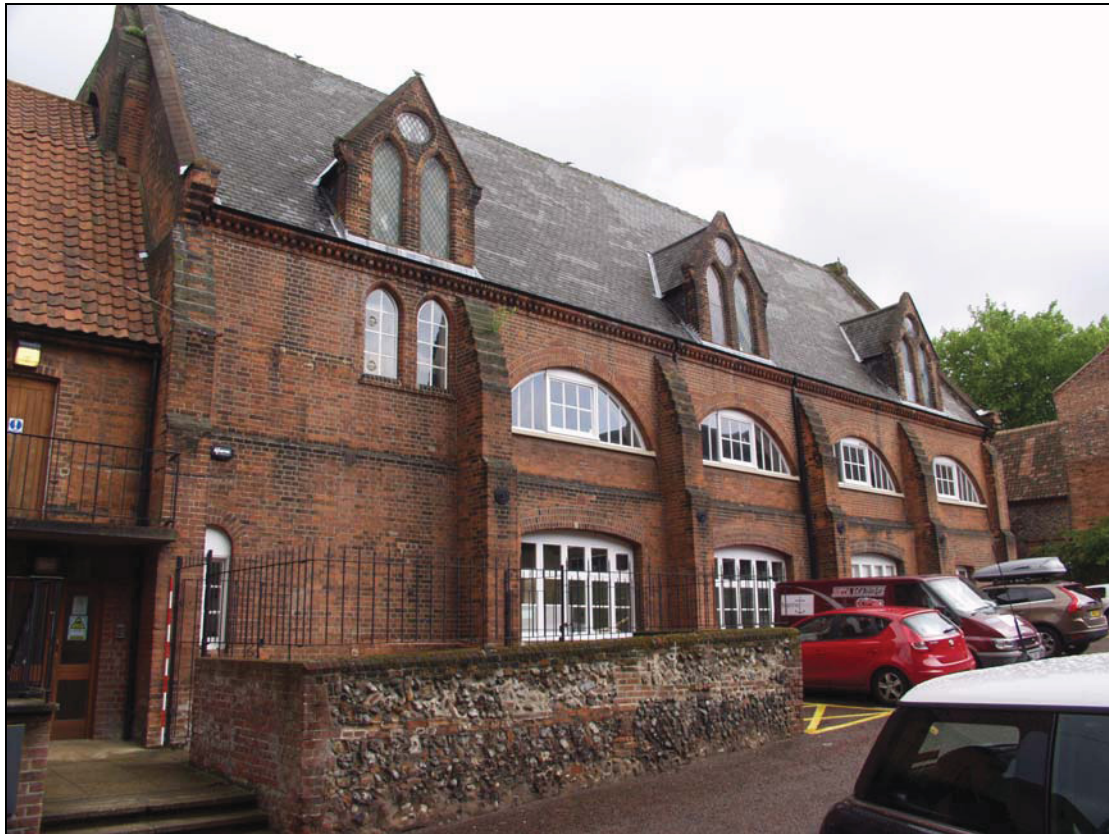
Plate 1 South-west elevation of the assessment building, taken from the west (DP 03)
