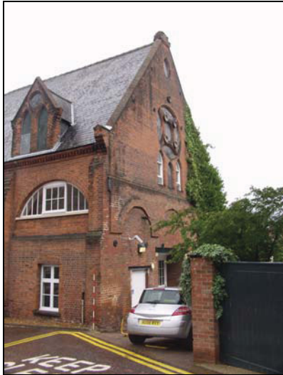
DP 1 South-east elevation of the assessment building, taken from south
