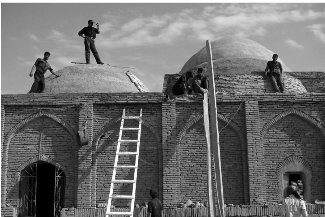
17. Masons insert dry packing in the interstices
