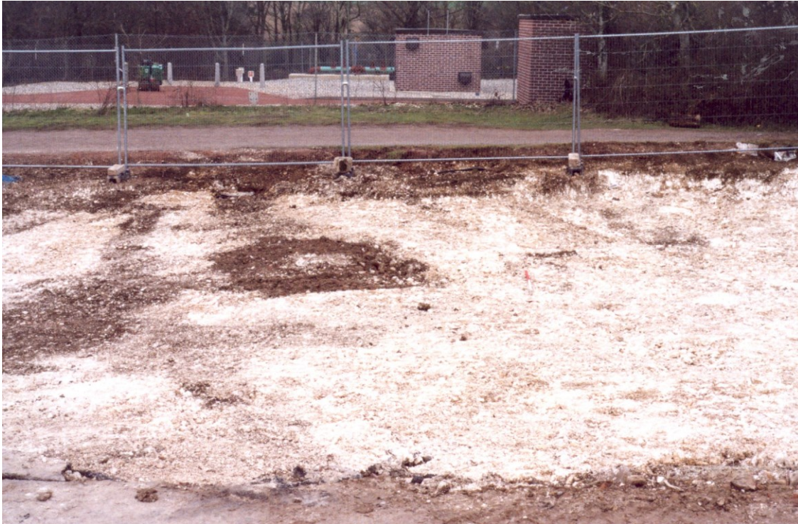
Plate 2: Area B following backfilling of drainage sump pit (looking N)
