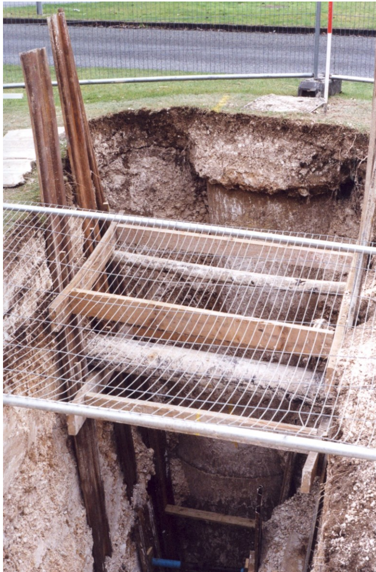
Plate 6: Concrete inspection chamber and pit (facing S)
