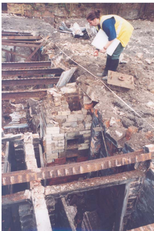
Plate 13 Possible brick ventilation structure in the air raid shelter (Structure P)
