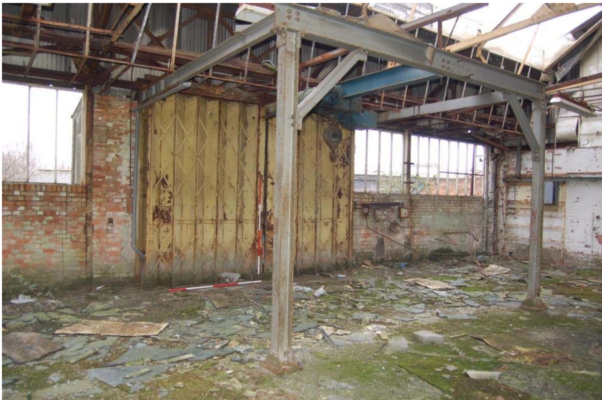
Plate 41: Building G, first floor (E); hoist mechanism
