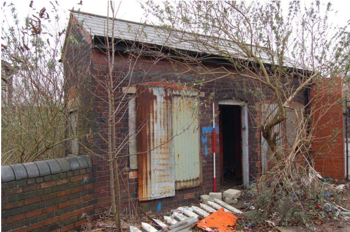
Plate 62: Building S from the west.
