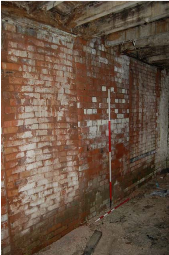
Plate 29: Bldg D, 1 st floor; early fabric in side bay.
