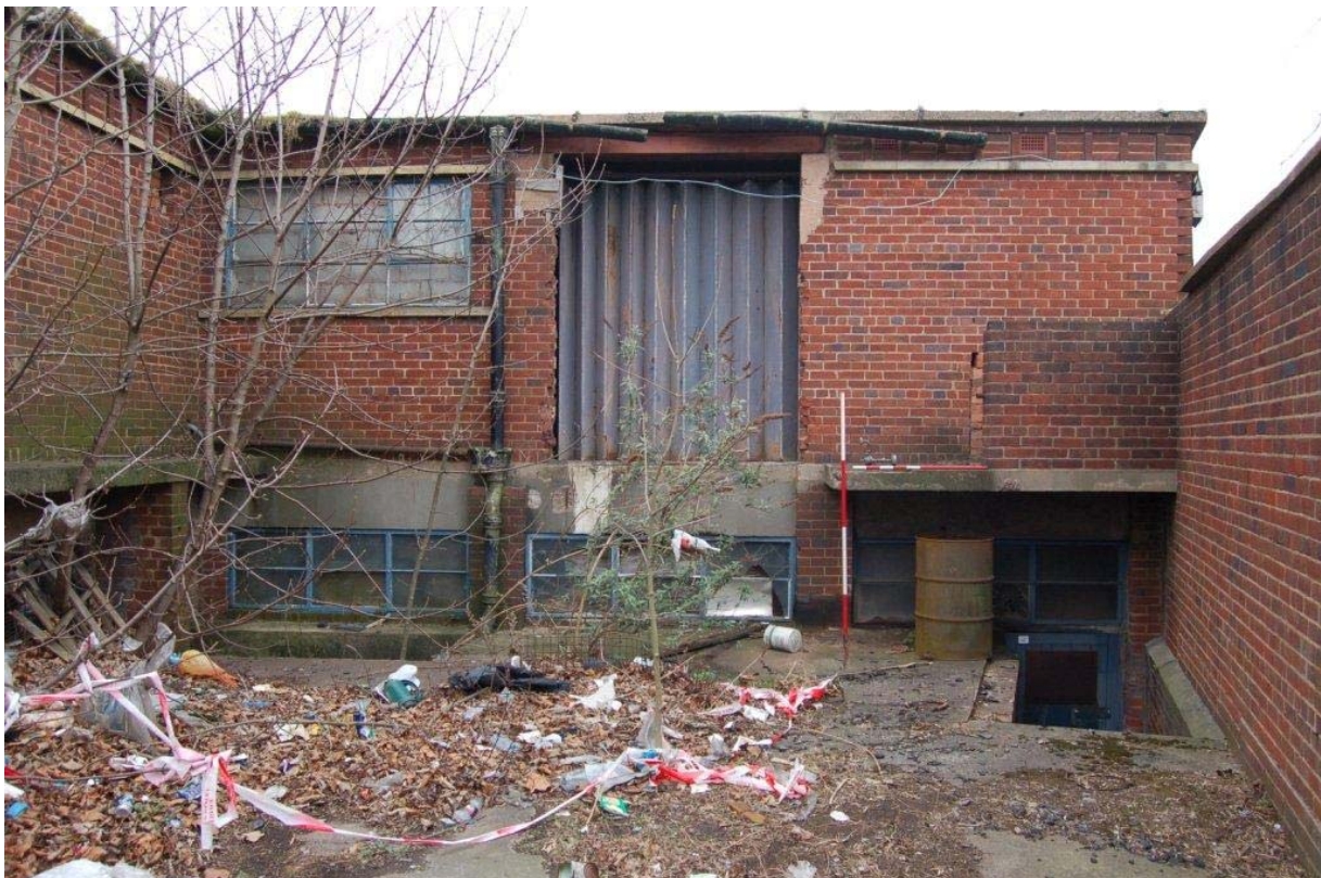
Plate 61: Building R, south elevation viewed from loading platform.
