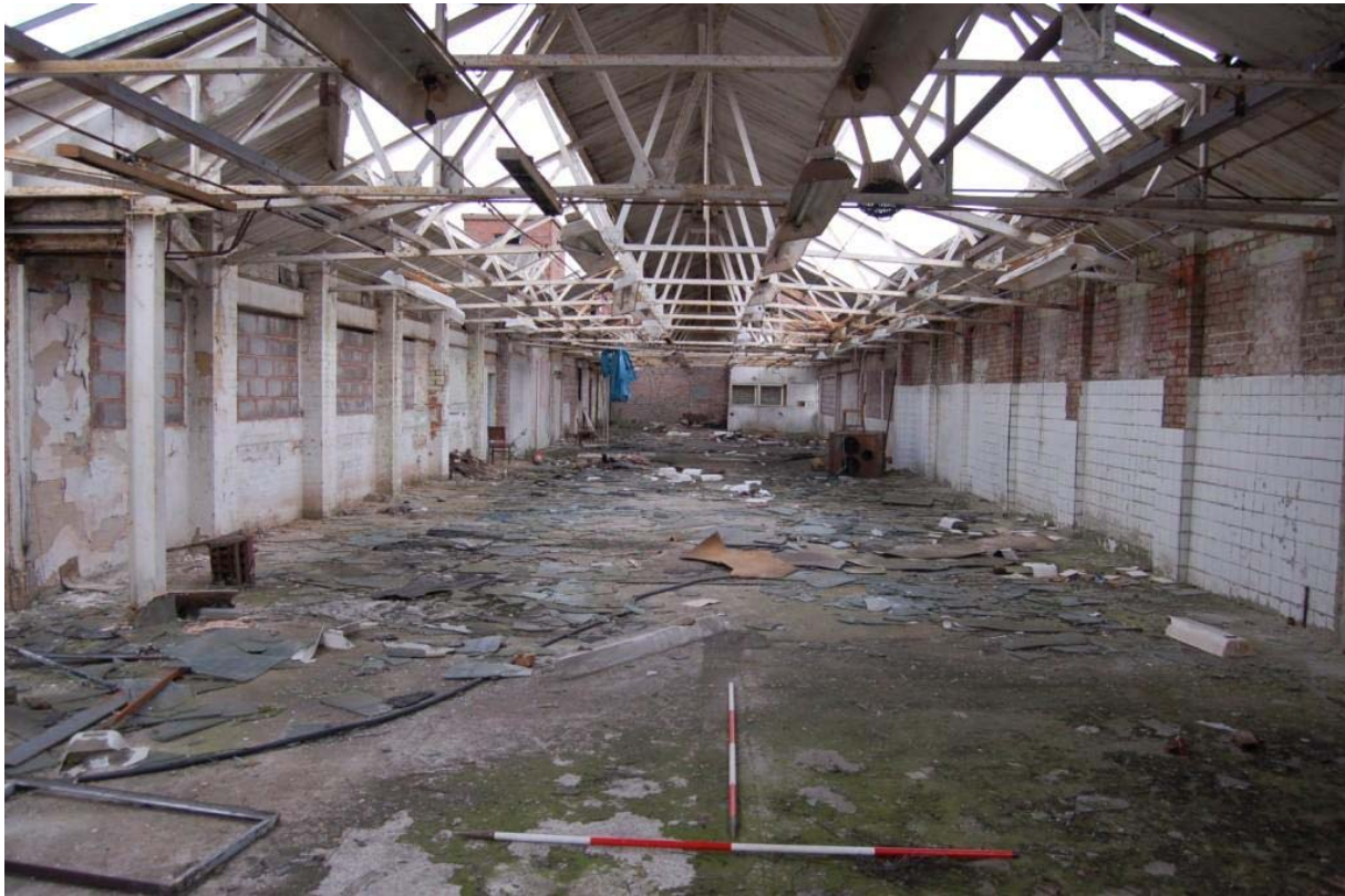
Plate 25: Building D, first floor looking north.
