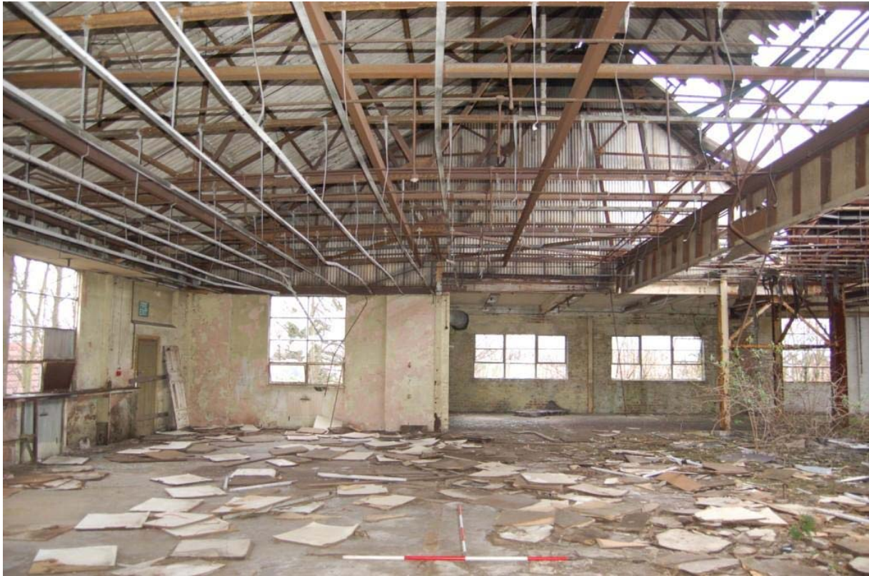
Plate 40: Building G, first floor (W) looking north. Note asymmetrical roof profile.
