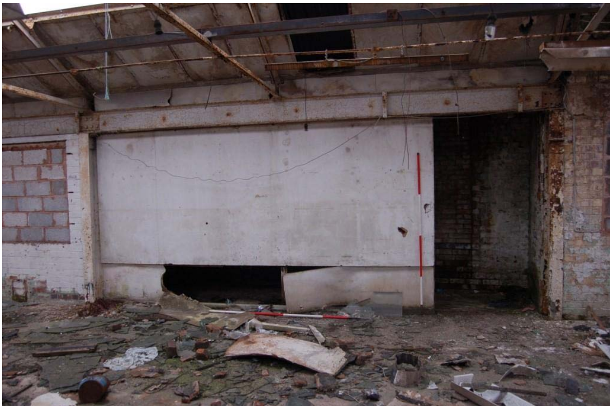
Plate 28: Building D, first floor, east; side bay retaining early fabric.
