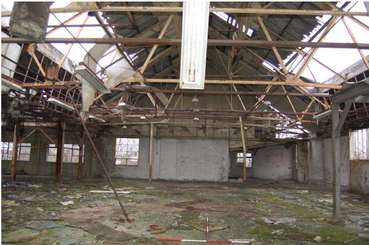
Plate 39: Building G, first floor (E) looking north.
