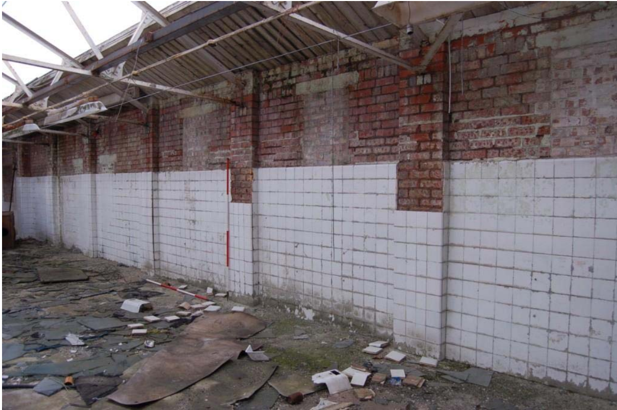
Plate 27: Building D, first floor central section.
