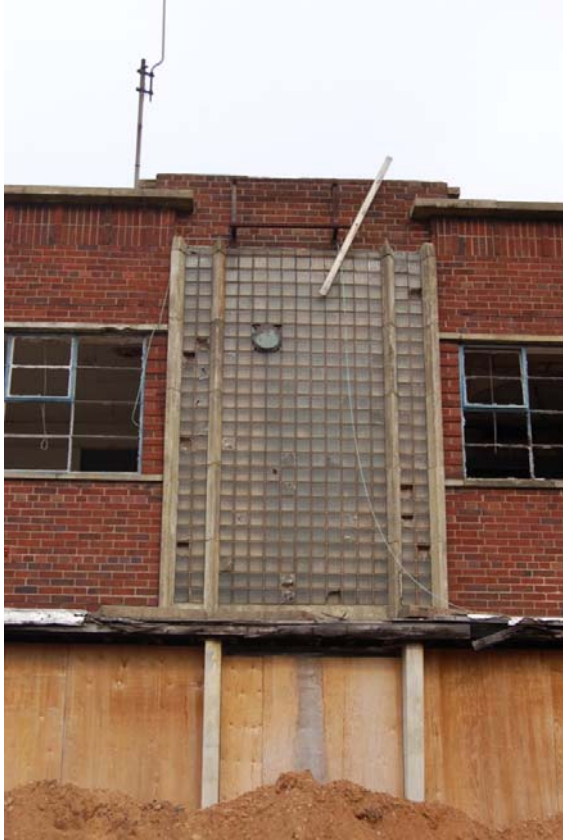
Plate 5: Bldg. B1, glass block window . above central entrance
