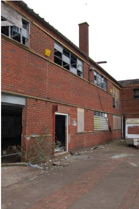
Plate 15: Bldg C, oblique view from southwest. lighting stairwell.
