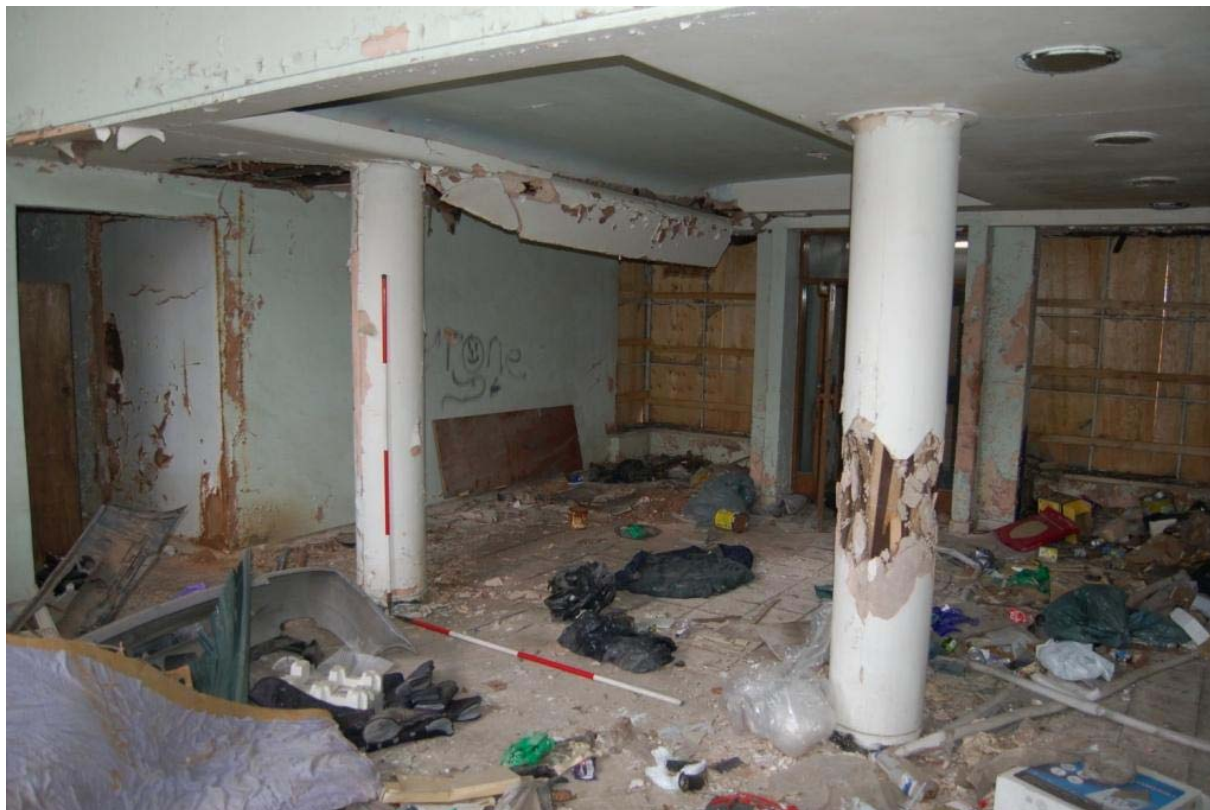
Plate 8: Building B1, pier supports to balcony of principal stair.
