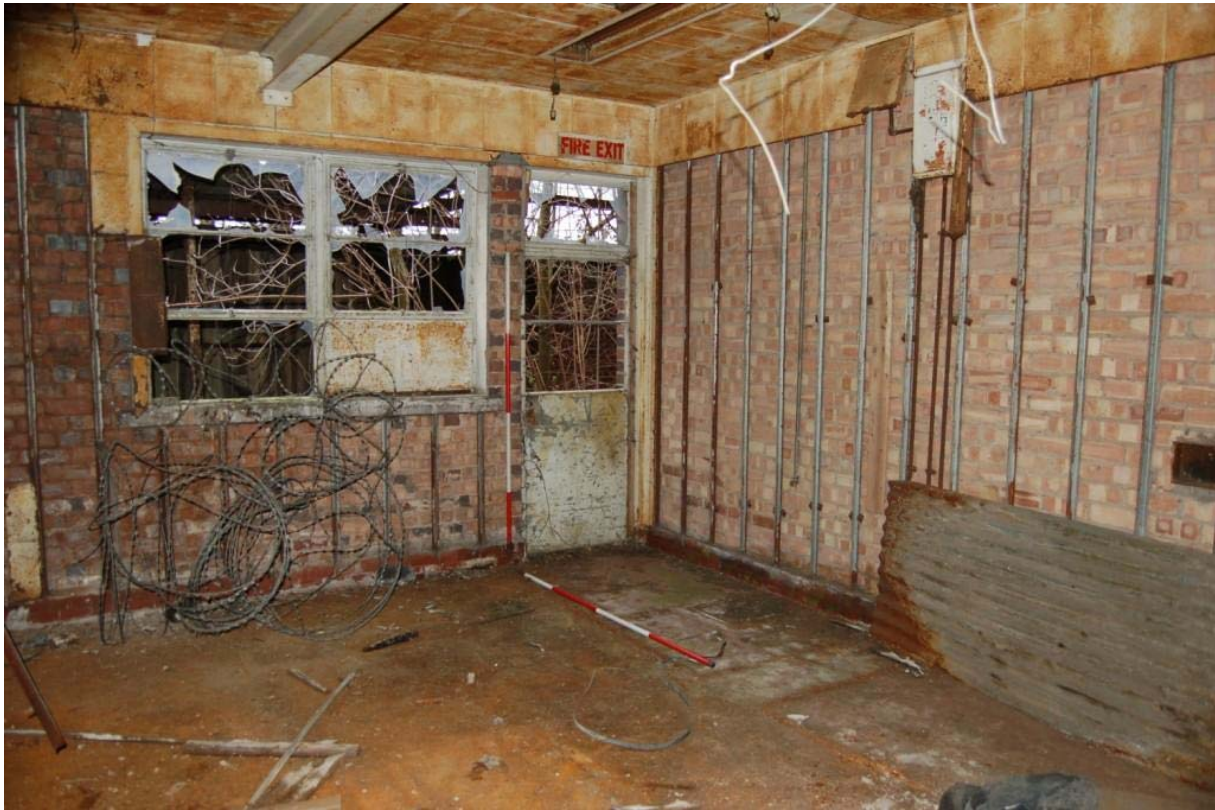
Plate 38: Building G, ground floor, enclosed room to north side.
