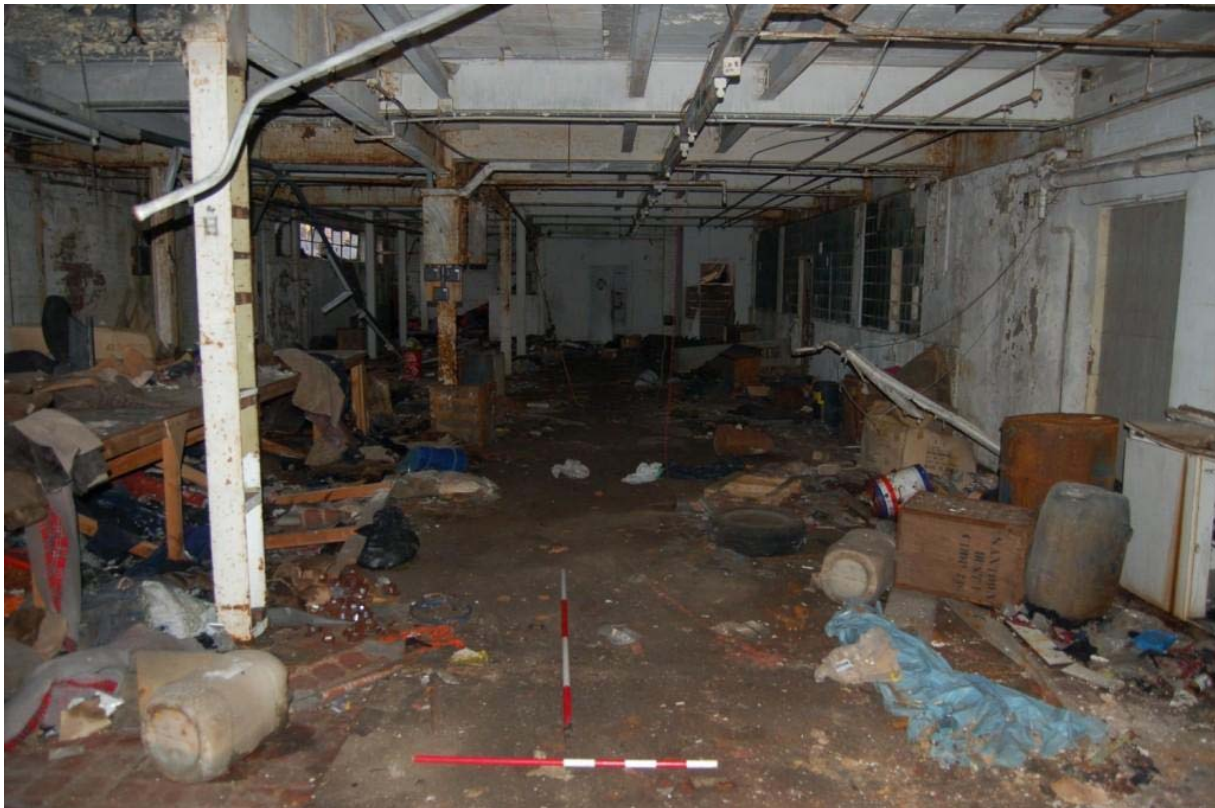
Plate 21: Building D, ground floor looking south.
