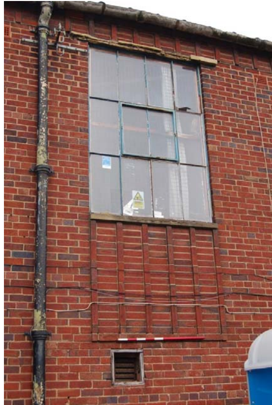
Plate 16: Bldg C, window with decorative panel
