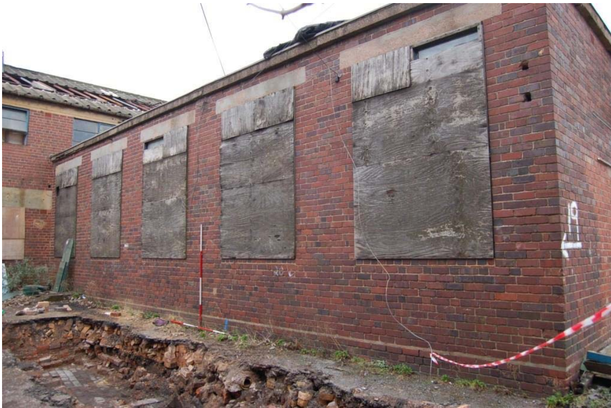
Plate 32: Building E, east elevation oblique view.
