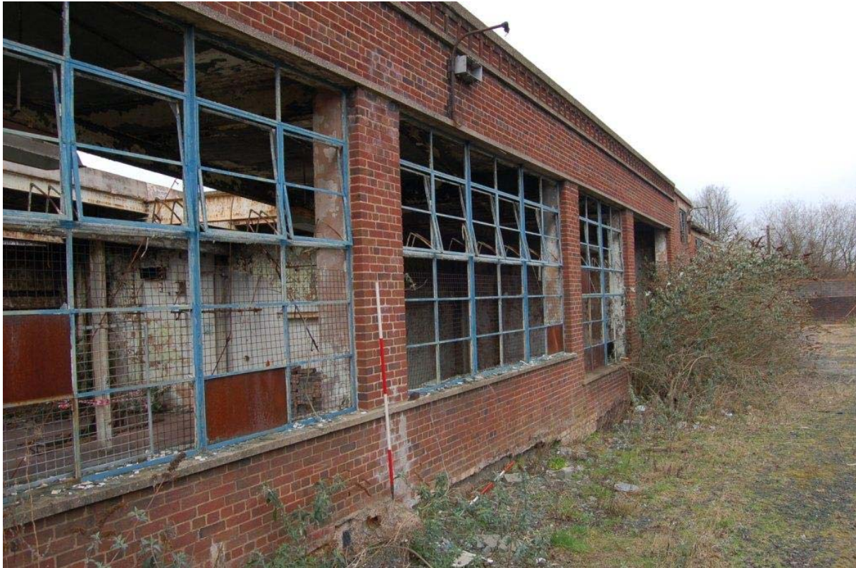
Plate 42: Building H, east elevation; oblique view from south.
