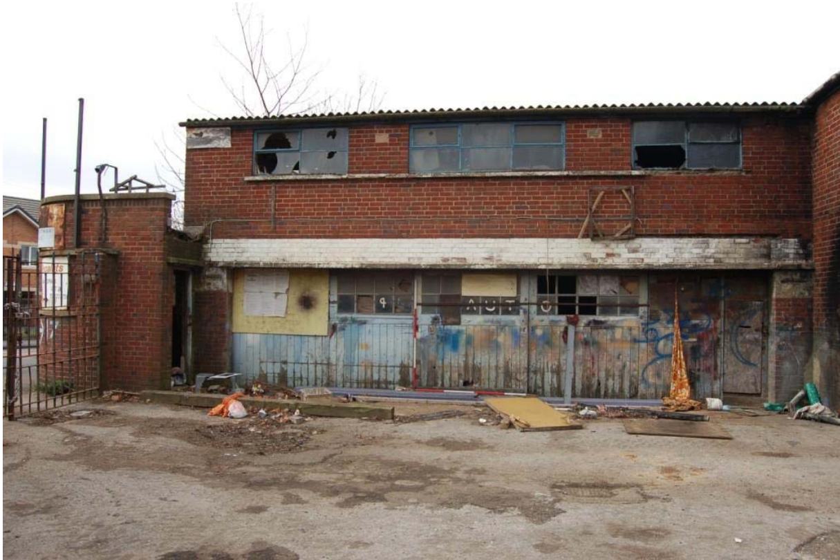
Plate 3: Building A, east elevation to yard.
