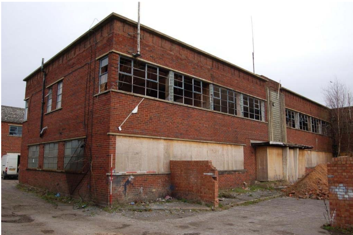
Plate 4: Building B1, oblique view from the southwest.
