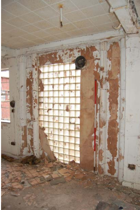
Plate 11: Bldg B1, 1 st Floor; central window, South elevation.
