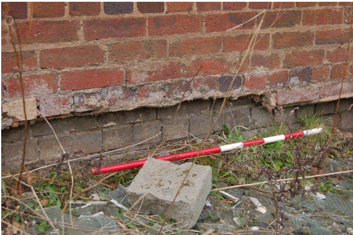
Plate 43: Building H, east elevation; (early ? C19 th ) English bond brickwork exposed at base of wall.
