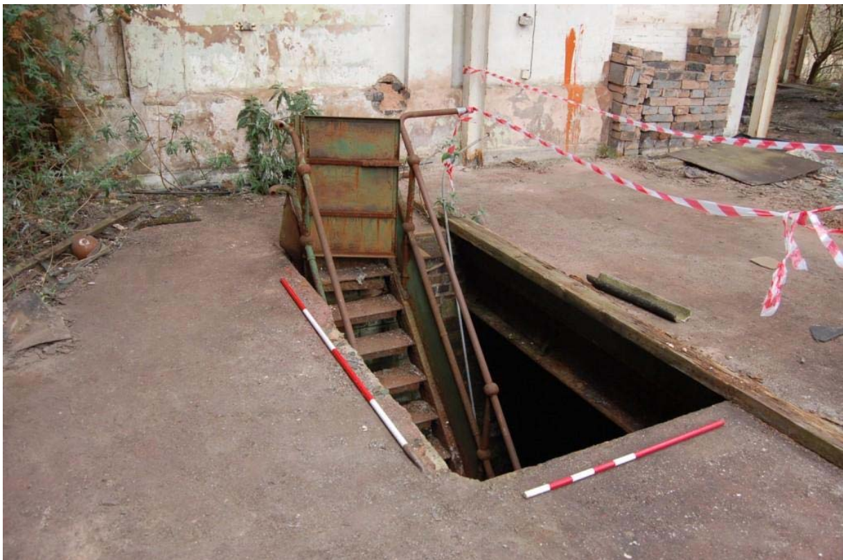
Plate 45: Building H; stairwell descending to basement area.
