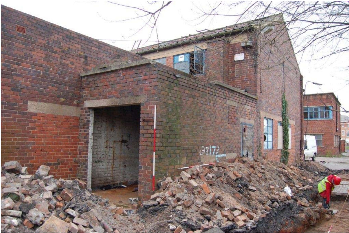
Plate 34: Building F, oblique view from northwest.
