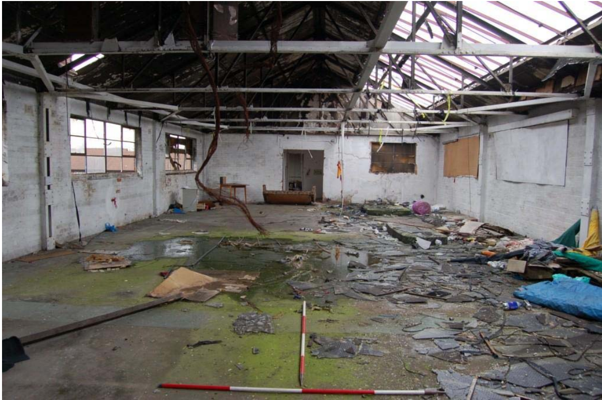
Plate 18: Building C, first floor looking west.
