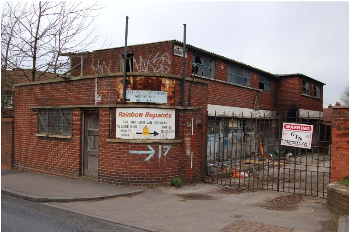
Plate 2: Building A, oblique view from southeast.
