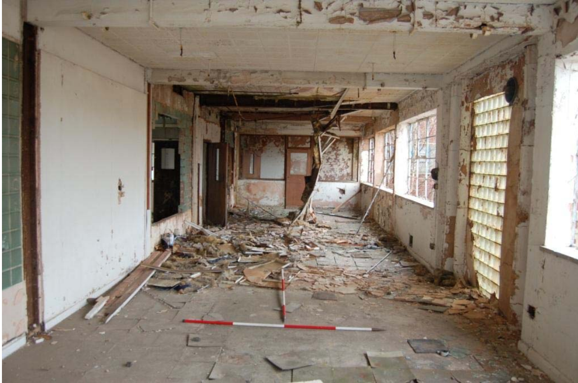
Plate 10: Building B1, first floor. (Note continuous glass-block walling to left).
