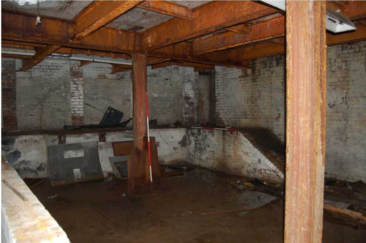
Plate 66: Tunnel complex beneath building H, Area H1, looking south
