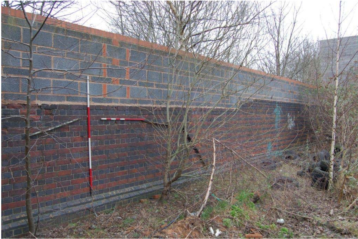
Plate 64: Northeast boundary wall of site.
