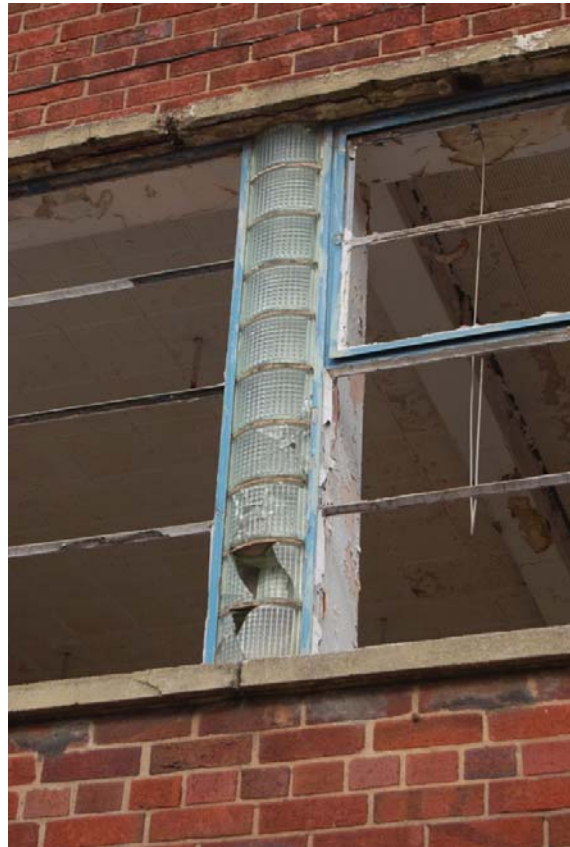
Plate 6: Bldg B1; Detail of glass brick window pier.
