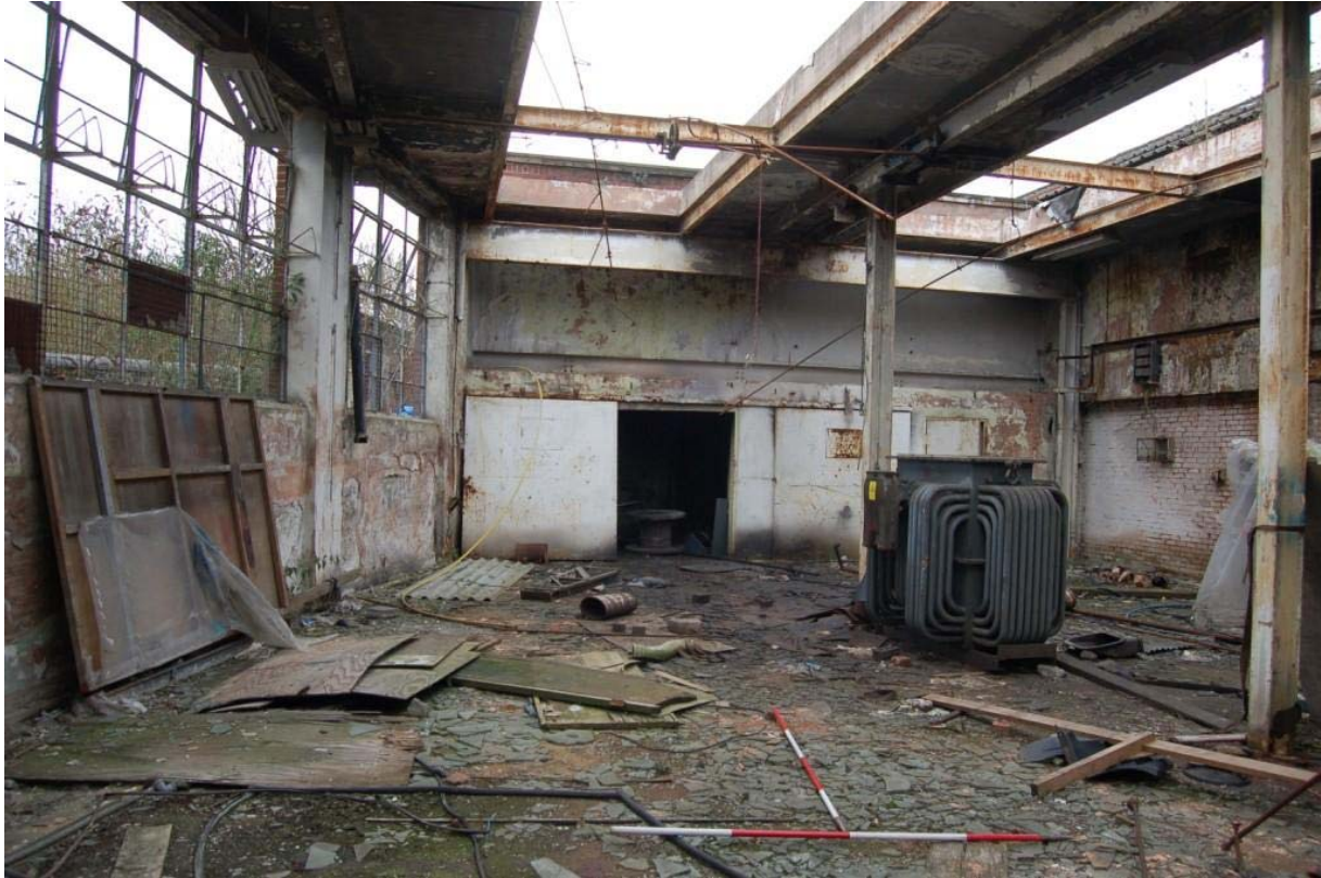
Plate 44: Building H, interior looking south.
