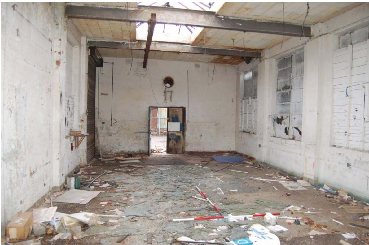
Plate 33: Building E, interior looking north.
