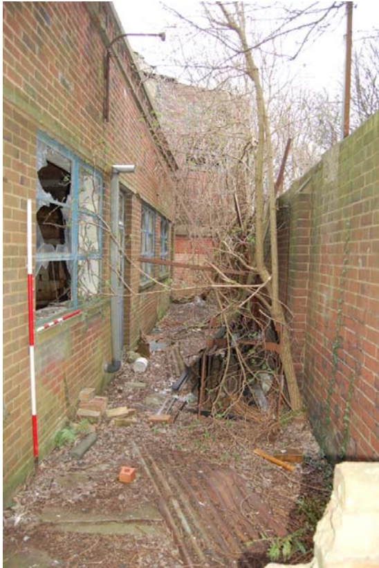
Plate 55: Building M, north elevation, oblique view.
