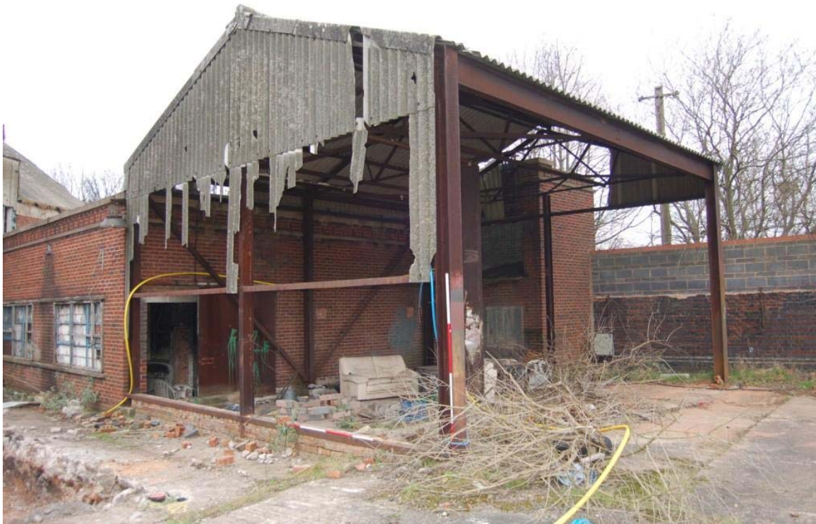
Plate 54: Hoist at east end of Building M
