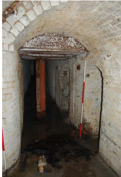
Plate 69: Tunnel complex beneath building H, Corridor H4, looking southeast
