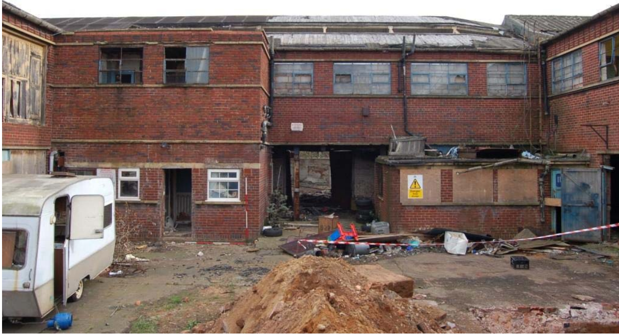
Plate 20: Building D and angle structures, west elevation.
