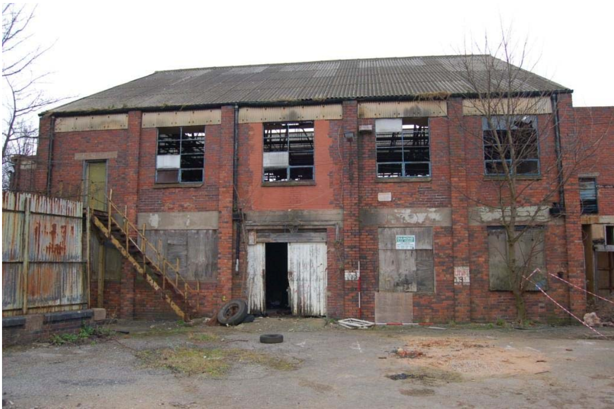
Plate 35: Building G, west elevation.
