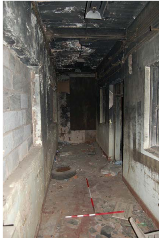
Plate 56: Building M, lateral corridor.
