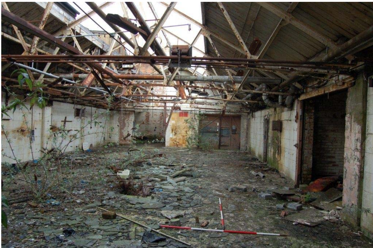
Plate 47: Building K interior looking north.
