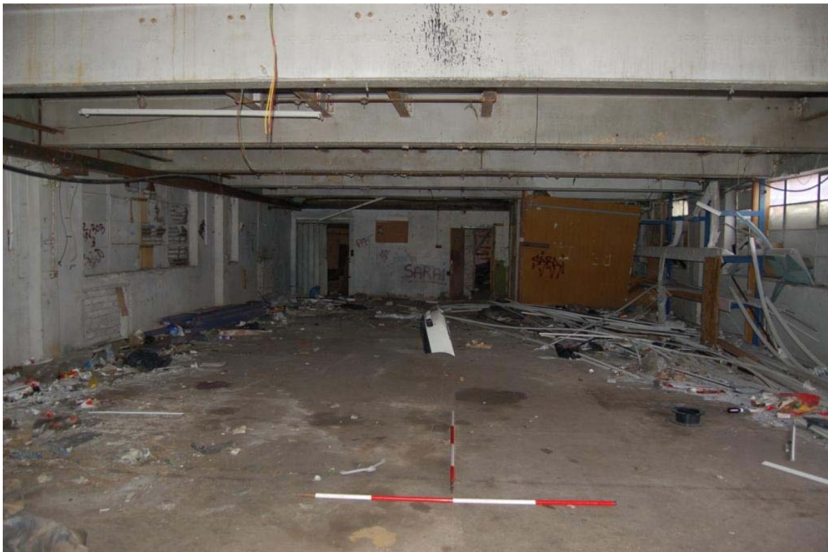
Plate 17: Building C, ground floor looking east.
