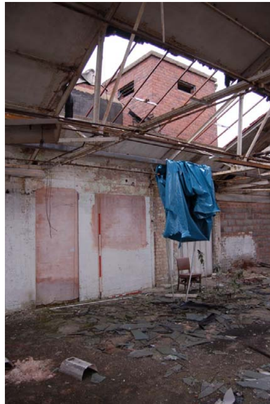
Plate 30: Bldg D, 1 st floor, west. Blocked doors to Bldg C.
