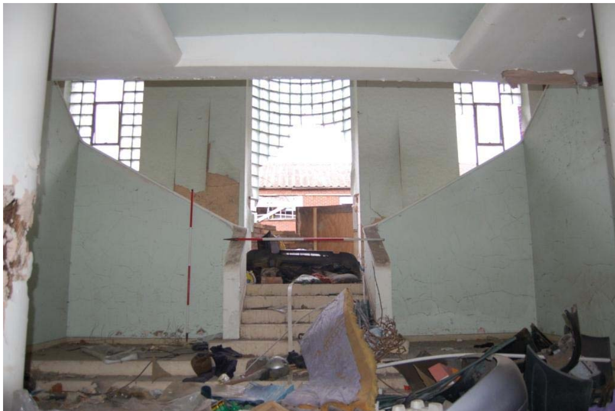
Plate 9: Building B1, principal stair.
