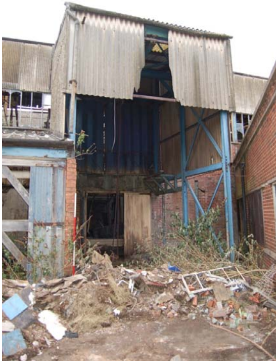
Plate 52: Hoist serving 1 st floor of Building G.
