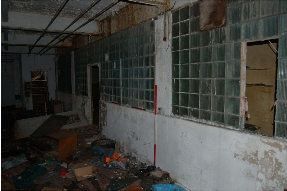
Plate 22: Building D, ground floor; detail of glass-block division wall with Building B2.
