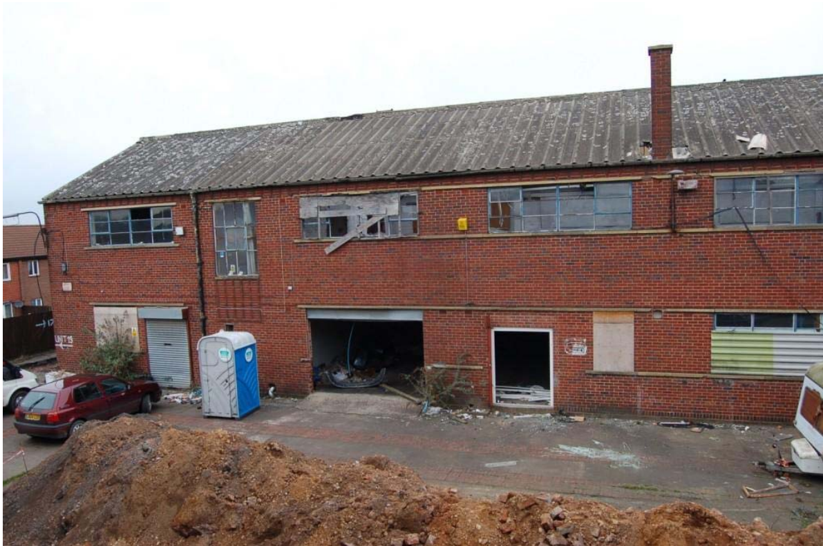
Plate 14: Building C, general view of south elevation, seen from first floor of Building B1.
