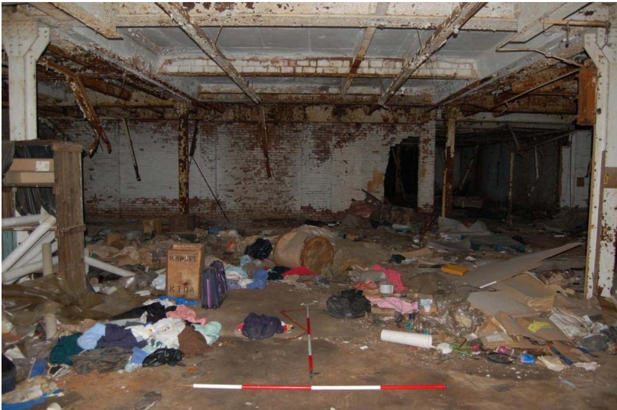
Plate 37: Building G, ground floor (west), looking east.
