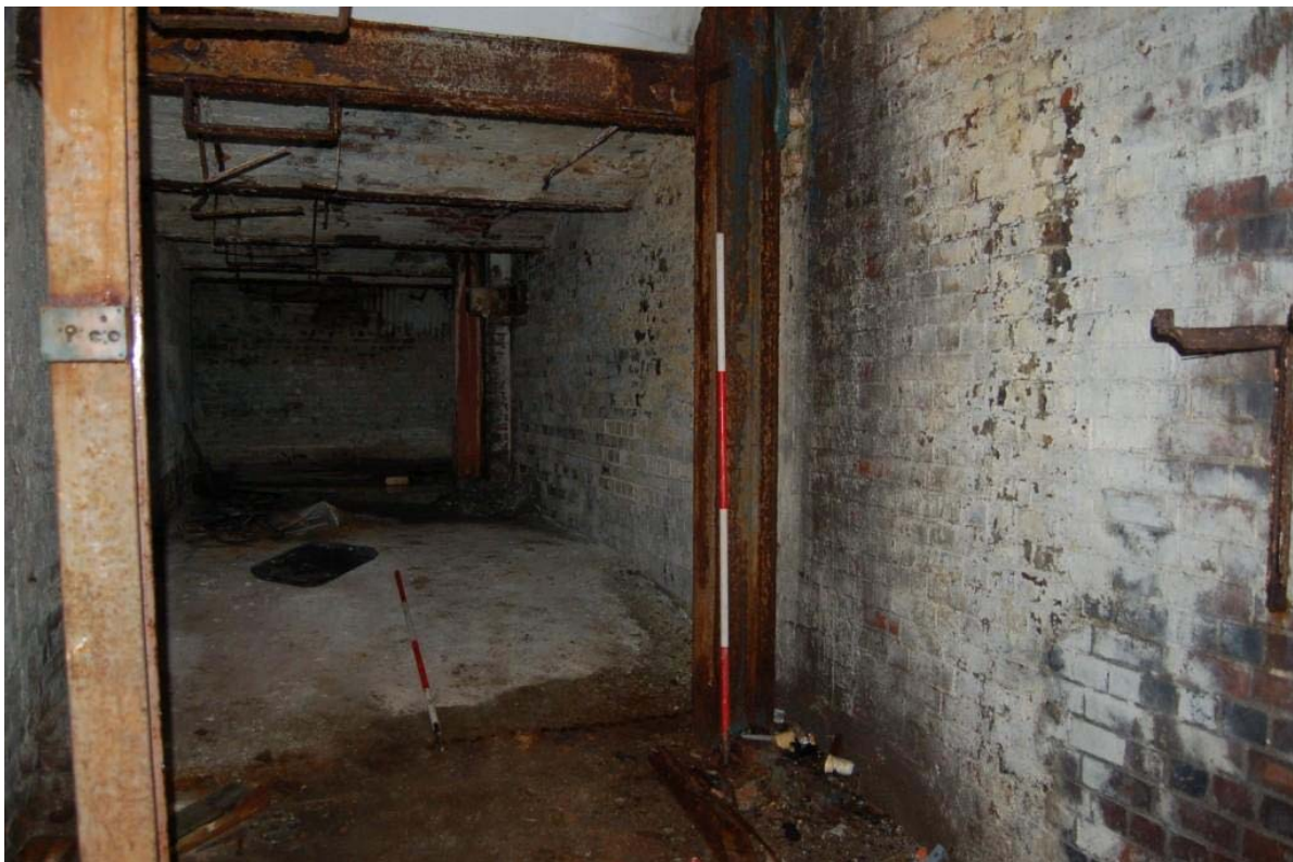
Plate 67: Tunnel complex beneath building H, Area H2, looking northwest
