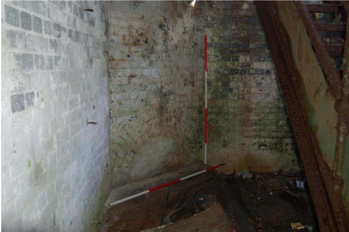
Plate 65: Tunnel complex beneath building H, Area H1- Blocked Arch, looking north
