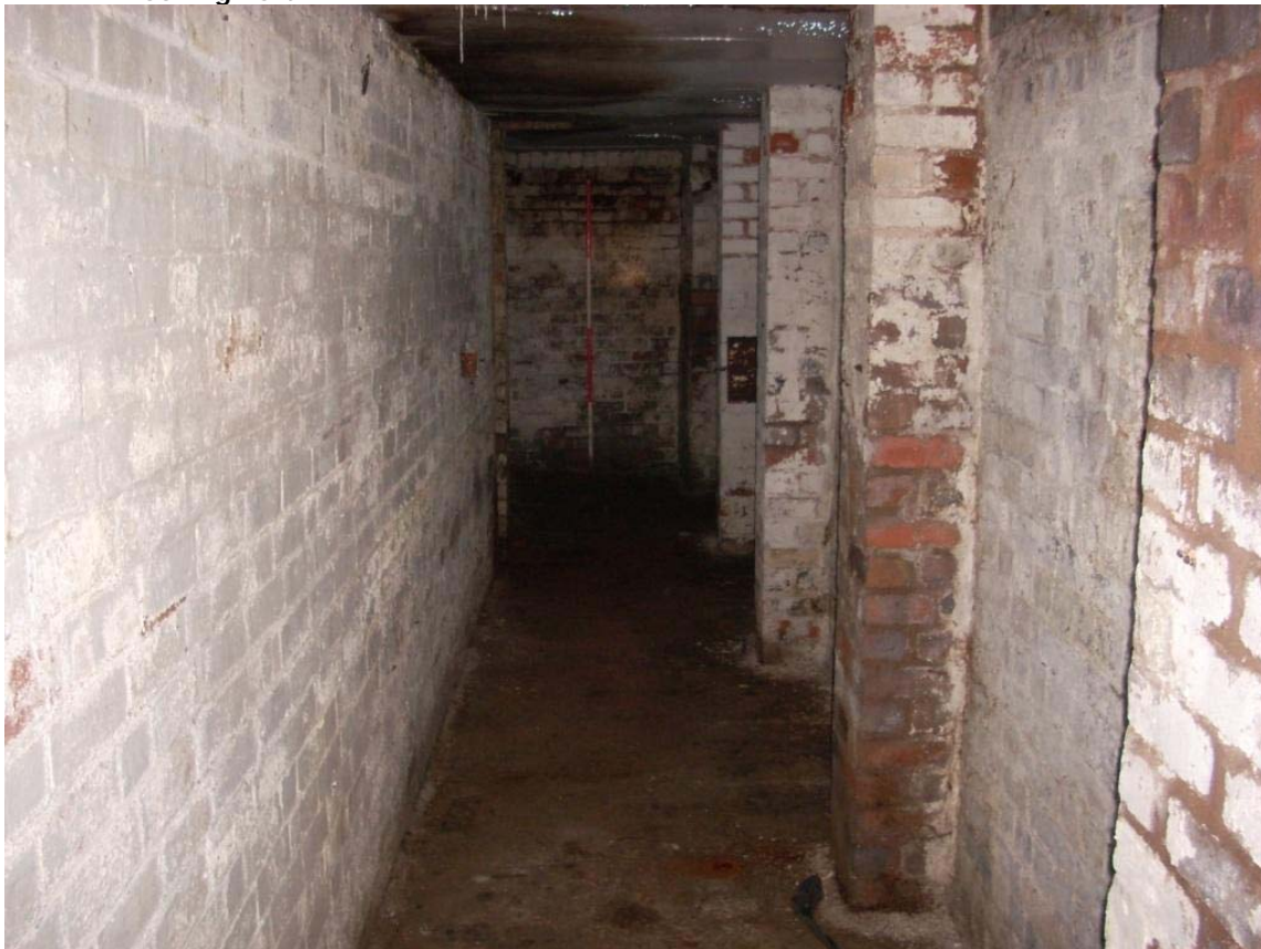
Plate 70: Tunnel complex beneath building H, Corridor H5, looking northeast
