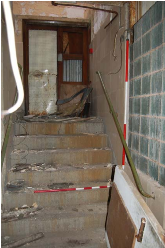
Plate 23: Bldg D, stair and mezzanine door to exterior.
