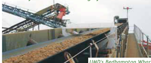
UMD's Bedhampton Wharf
