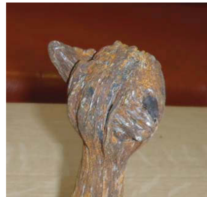
Close up of central upright
