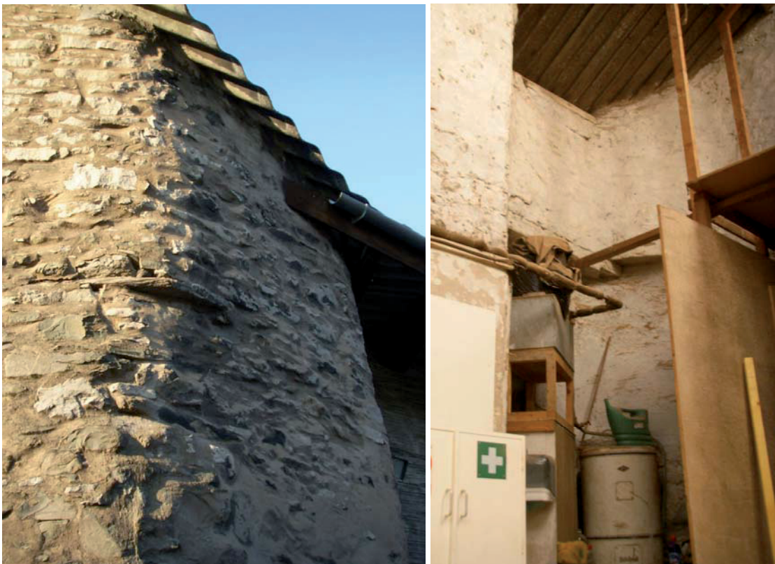
Plates 25-26: The exterior of the unusual building corner (with a timber board protruding), and the interior of the same part of the building
