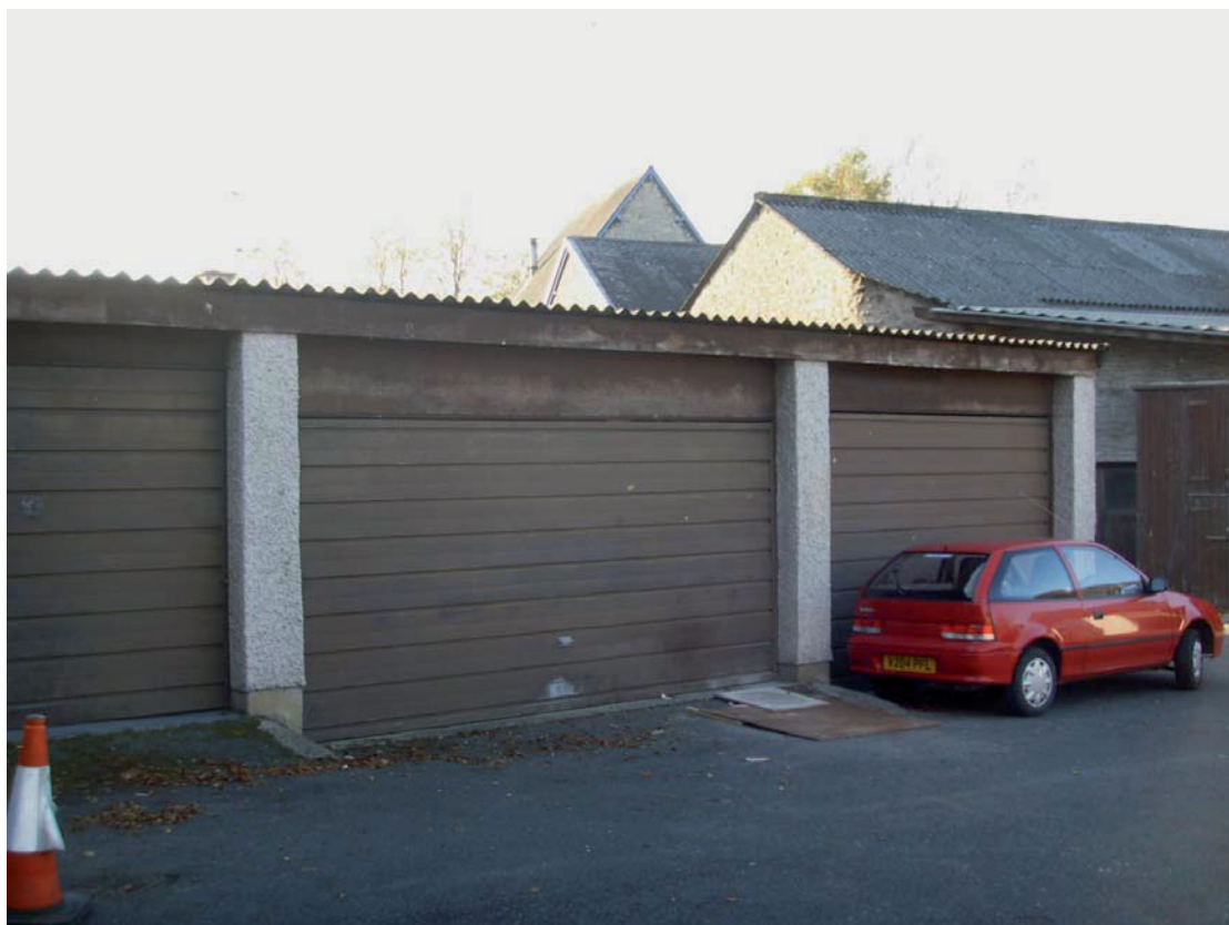
Plate 19: Front view of the garages to be demolished, facing west
