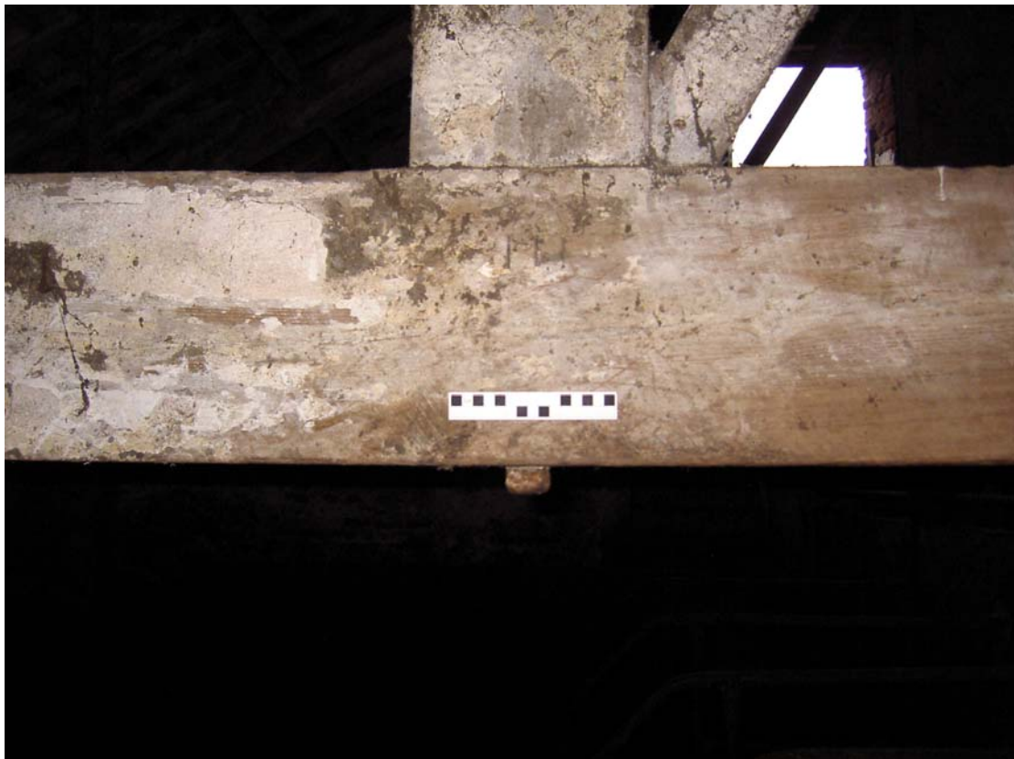
Plate 42: Carpenter's mark on the south face of Truss III
