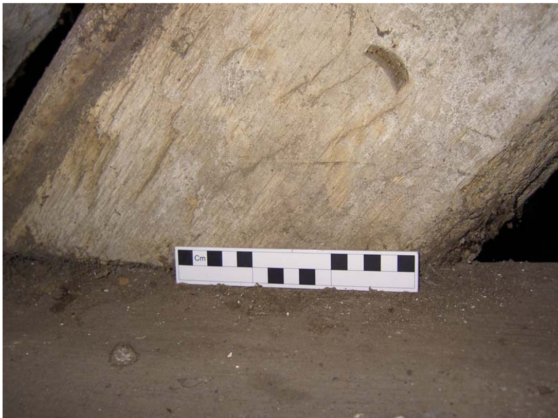
Plate 46: Punched carpenter's mark 'I' on the west side of Truss 1 within the barn
