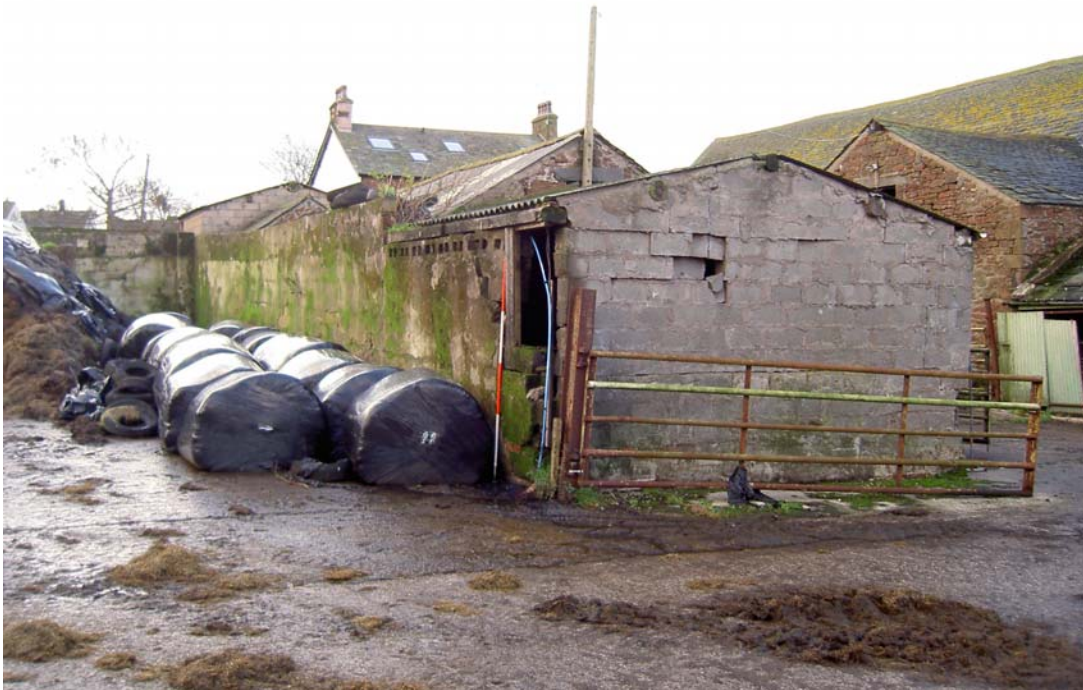
Plate 11: The north external elevation and the north end of the east external elevation of the dairy
