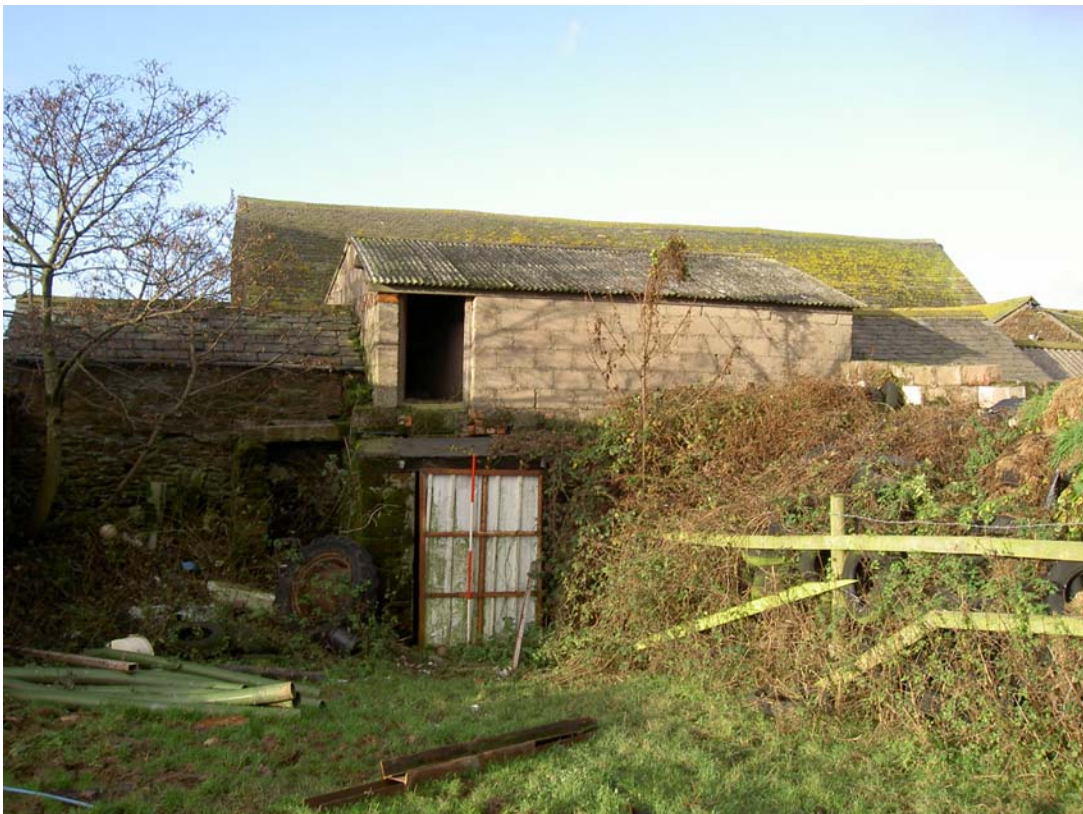
Plate 12: The south end of the east external elevation of the dairy
