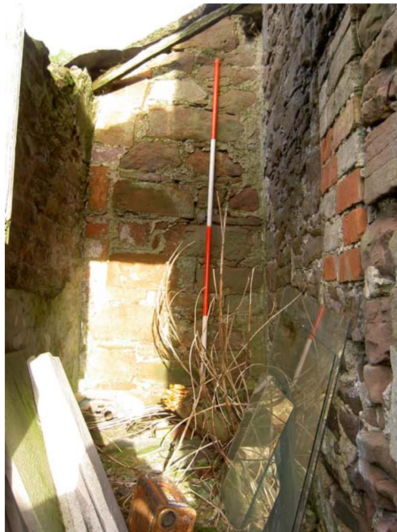
Plate 52: Buttress incorporated into the north wall of the south-west outshut attached to the barn
