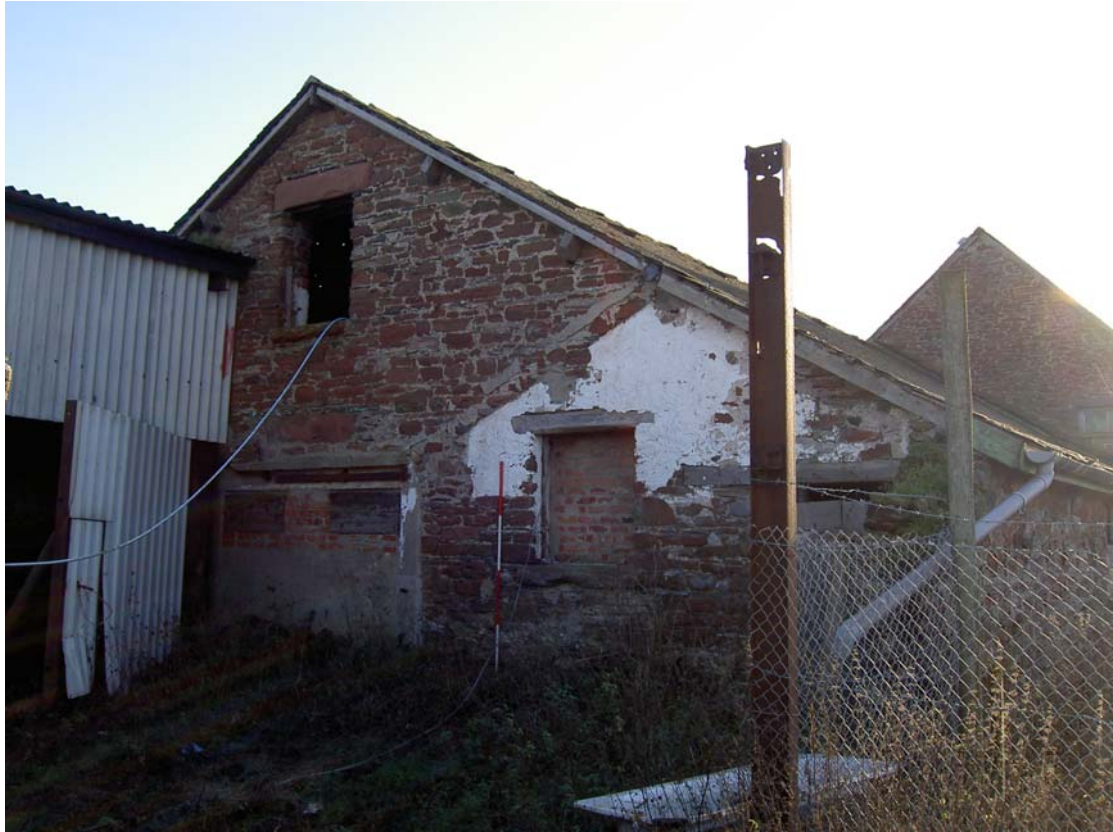
Plate 17: The west side of the north external elevation of the shippon
