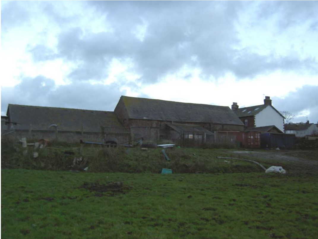
Plate 9: General view of the site from the west showing the barn and attached shippon and the farmhouse beyond
