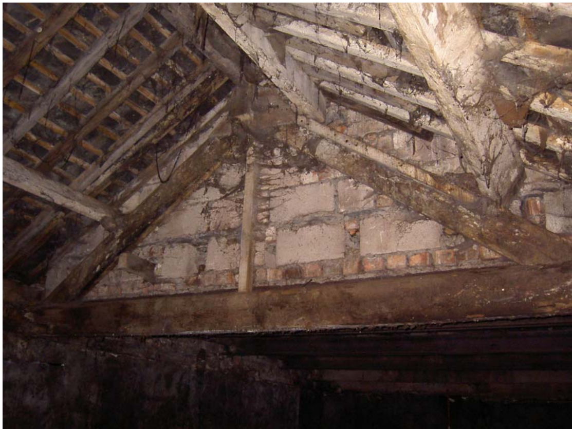
Plate 38: North side of truss within Room 4 of the dairy
