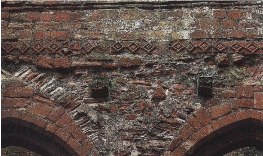
Plate 57: Decorative stone from the original 12 th century Savigniac church re-used in the 15 th century remodelling of the southern transept at Furness Abbey (after Harrison 1998, 8; compare with Plate 26)
