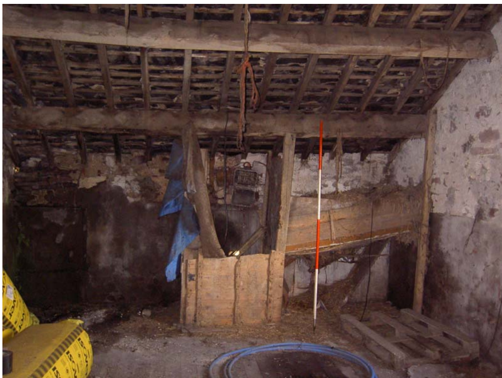
Plate 50: North side of the first floor of the north-east outshut attached to the barn showing the inserted walls associated with the grain crusher
