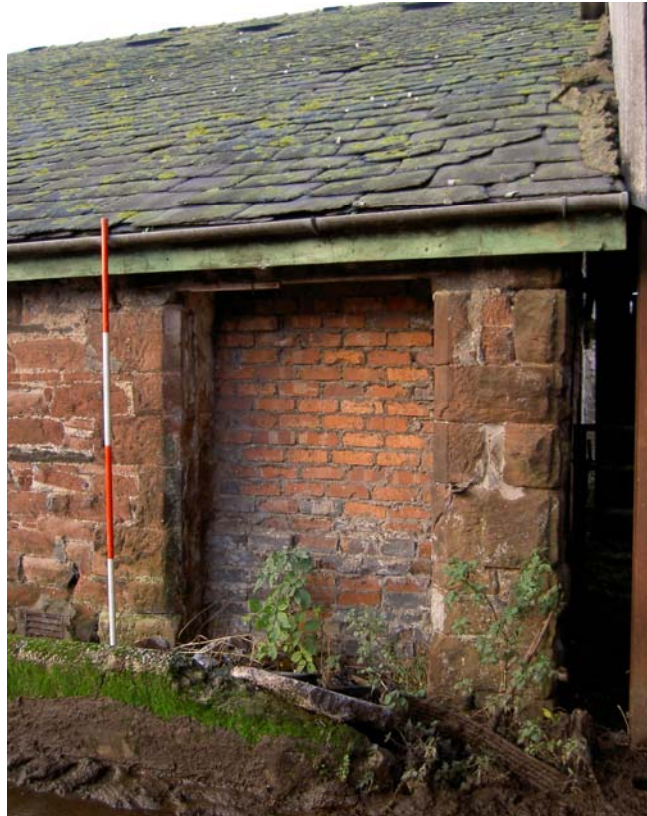
Plate 19: Doorway at the north end of the east external elevation showing the chamfered jambs
