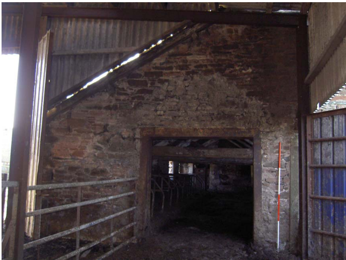
Plate 16: The east side of the north external elevation of the shippon
