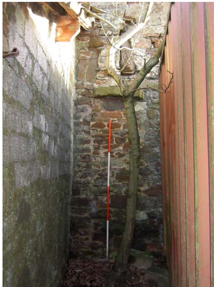
Plate 32: Blocked wagon doorway and projecting cruck base in the west external elevation of the barn
