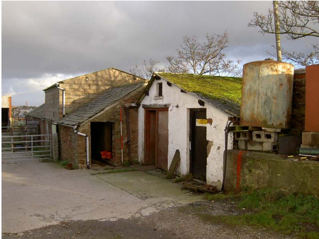
Plate 13: The south external elevation of the dairy
