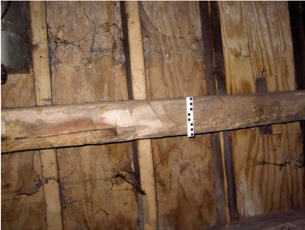
Plate 39: Baltic timber marks in the ceiling of Room 4 of the dairy
