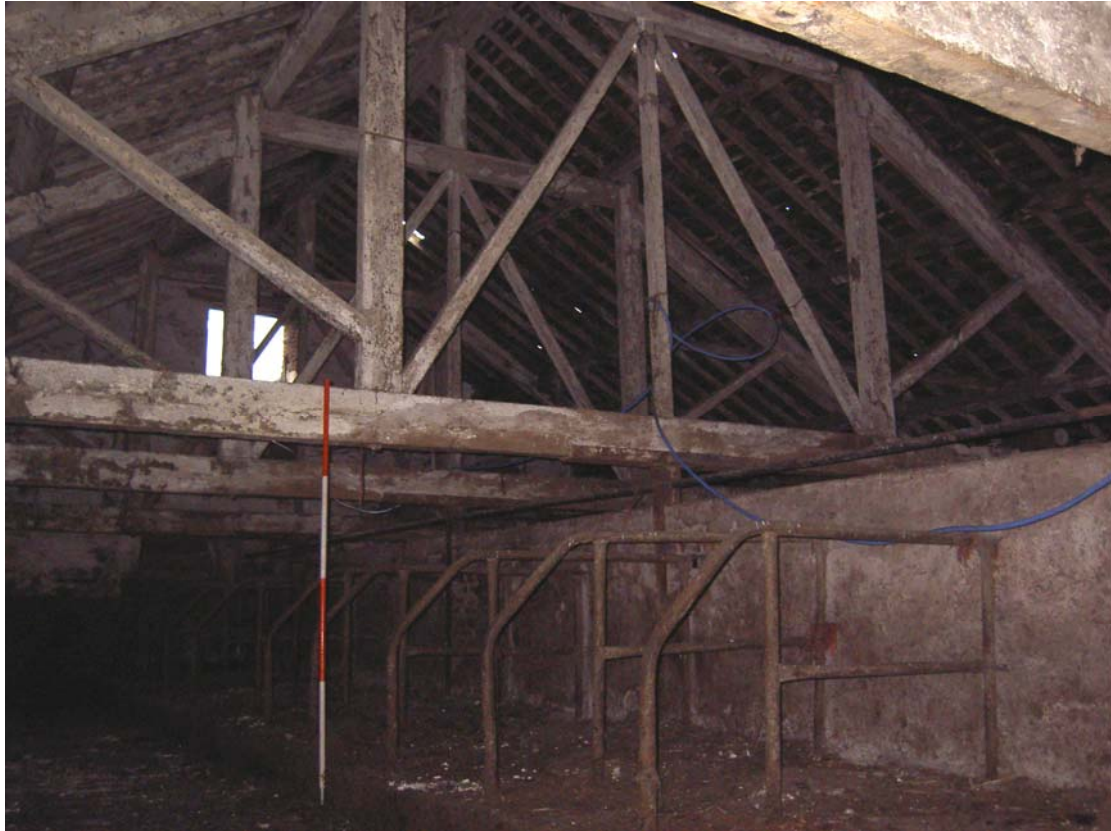
Plate 41: General view of the north side of the interior of the shippon
