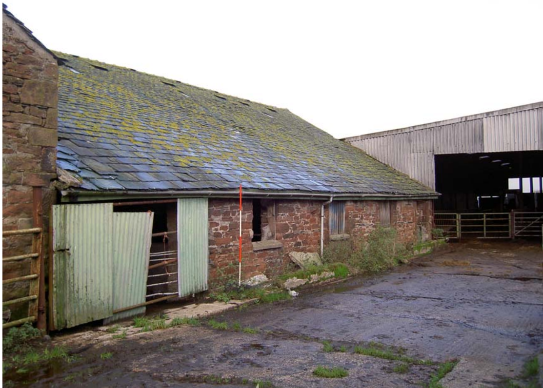
Plate 18: The east external elevation of the shippon
