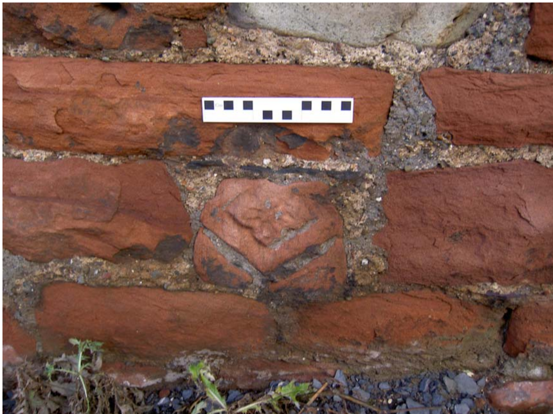
Plate 26: The re-used moulded stone decorated with petals enclosed by a rhombus in the south external elevation of the south-eastern outshut attached to the barn
