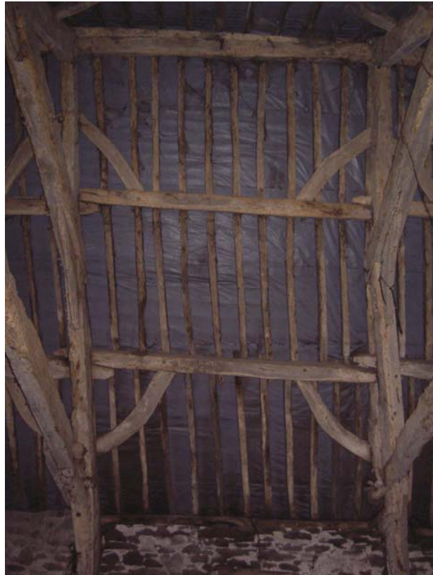
Plate 47: Typical arrangement of trusses and wind braces on the east side of the roof between Trusses 1 and 2
