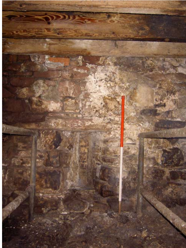
Plate 49: Blocked slot and re-used chamfered stone in the north wall of the ground floor of the north-east outshut attached to the barn
