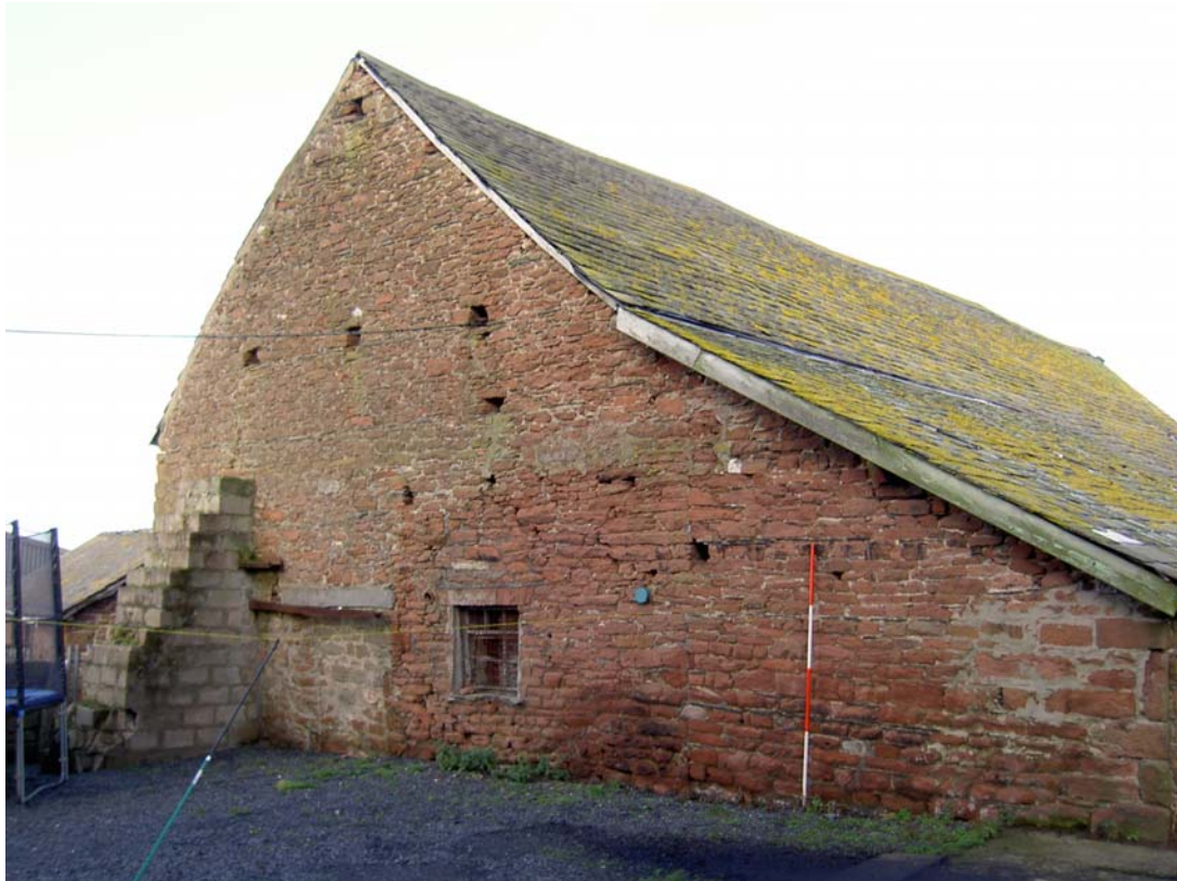
Plate 25: The south external elevation of the barn
