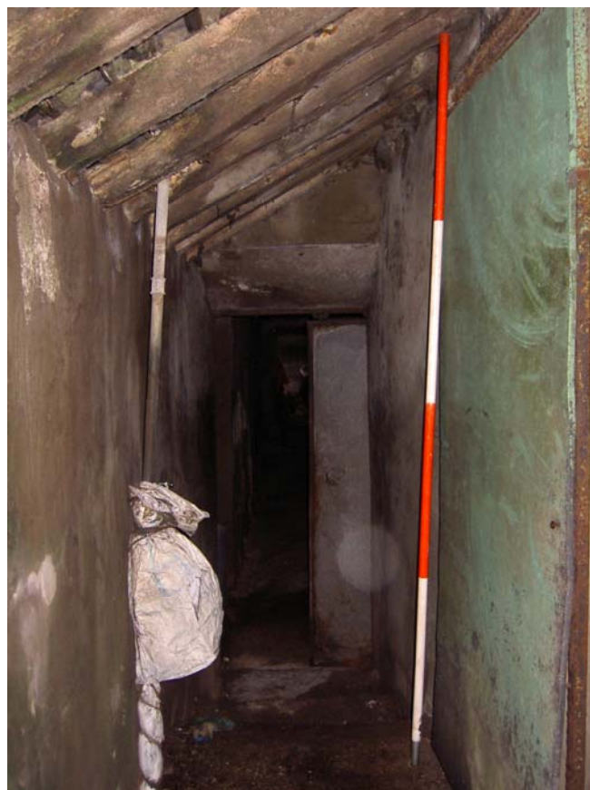
Plate 40: General view of the north end of the west side of Room 5 of the dairy
