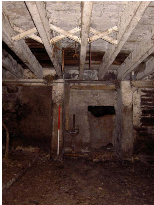
Plate 48: West side of the ground floor of the north-east outshut attached to the barn showing the cross-braced ceiling
