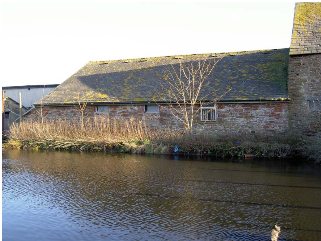
Plate 20: The west external elevation of the shippon
