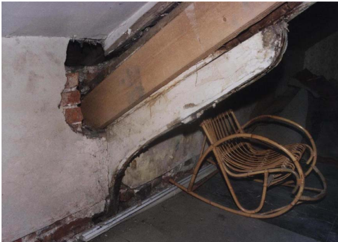
Plate 56: Angled brace bolted to a truss at 16 Queen Street, Ulverston
