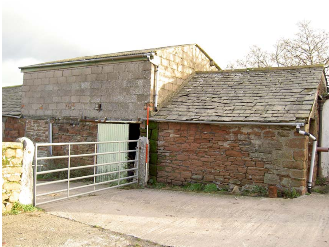
Plate 14: The south end of the west external elevation of the dairy
