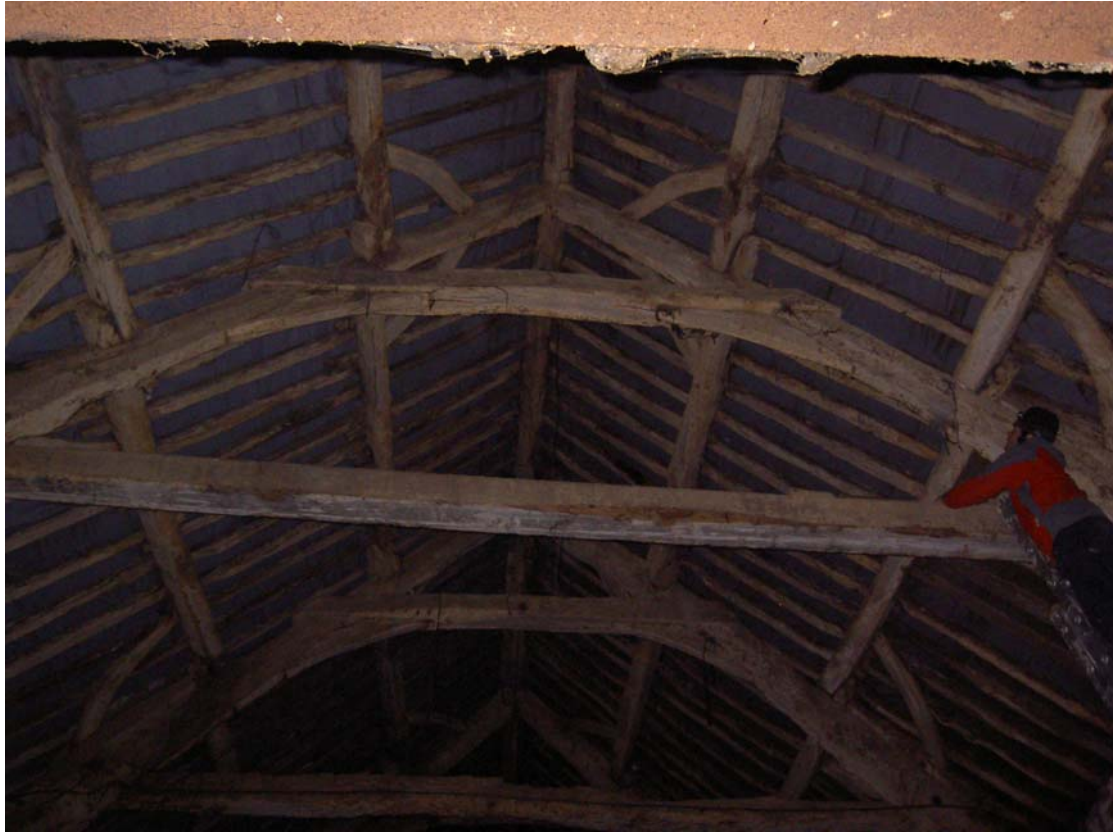
Plate 45: North faces of Trusses 1 and 2 within the barn
