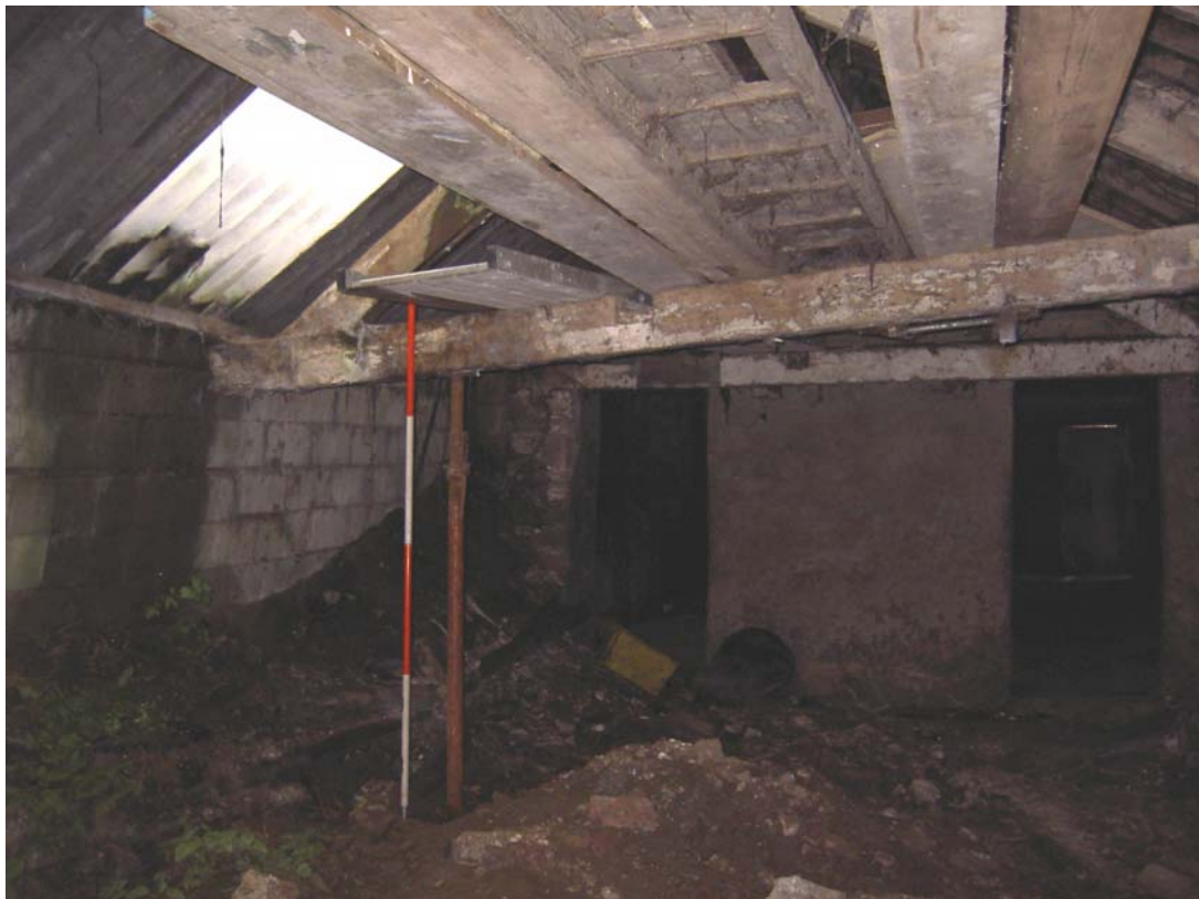
Plate 36: General view of the south end of Room 3 of the dairy showing the collapsed wall and trusses
