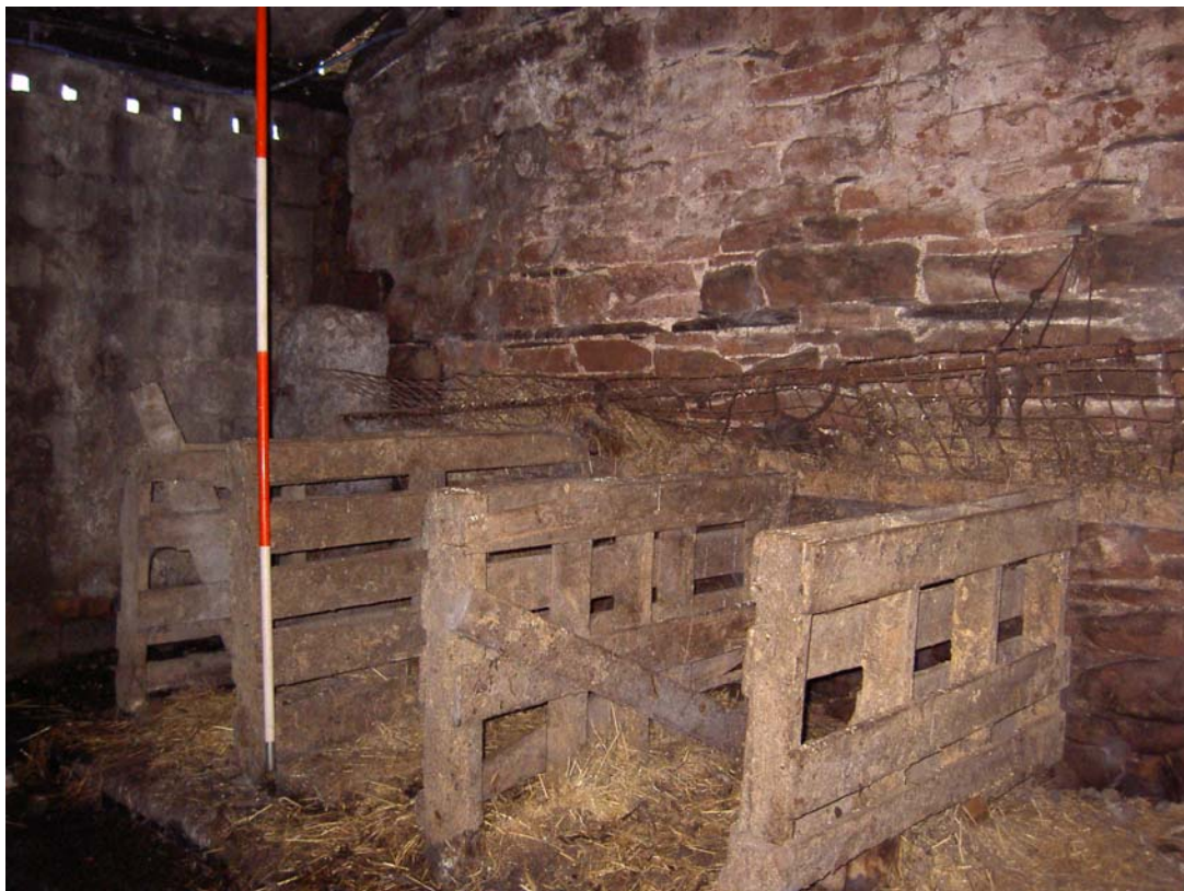
Plate 34: Stalls constructed from re-used pallets on the south side of Room 1 of the dairy
