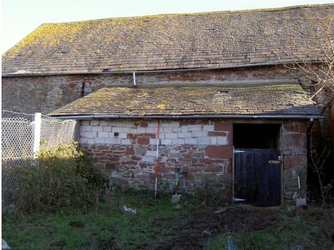
Plate 33: North-west outshut attached to the west external elevation of the barn
