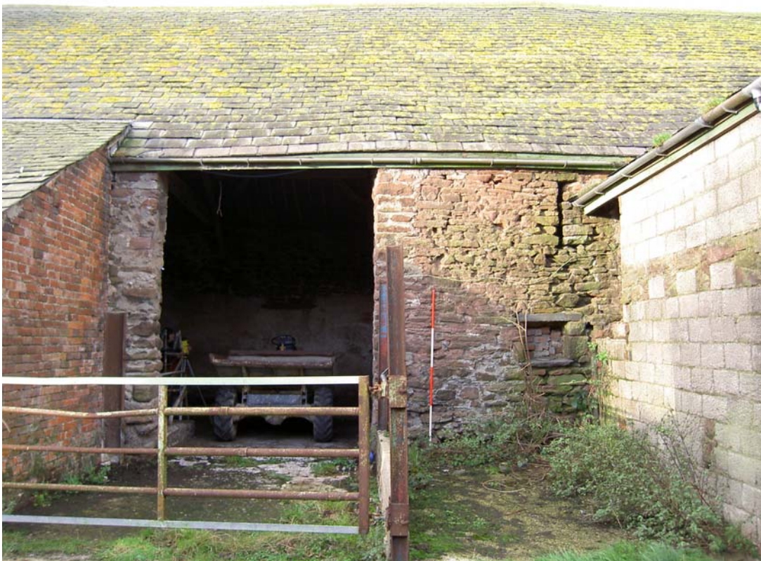
Plate 22: The wagon doorway in the centre of the east external elevation of the barn
