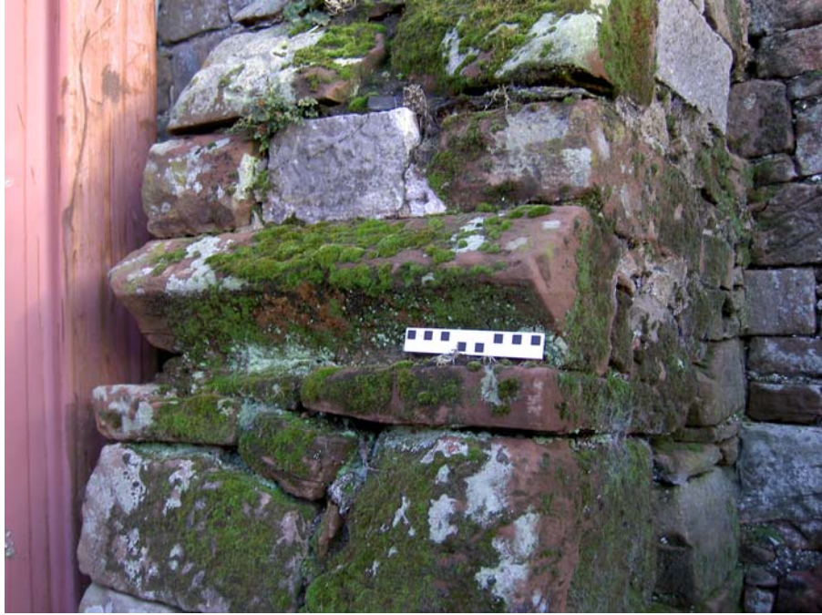
Plate 31: Re-used chamfered stone incorporated into the central buttress against the west external elevation of the barn
