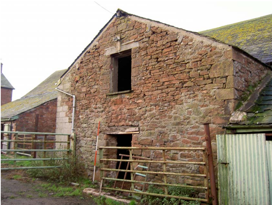
Plate 21: The two storey outshut at the north end of the east external elevation of the barn
