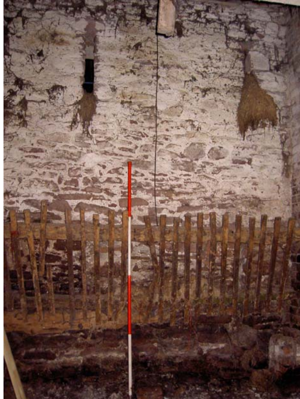
Plate 51: Ventilation slots and manger in the west elevation of the northern room of the south-east outshut attached to the barn
