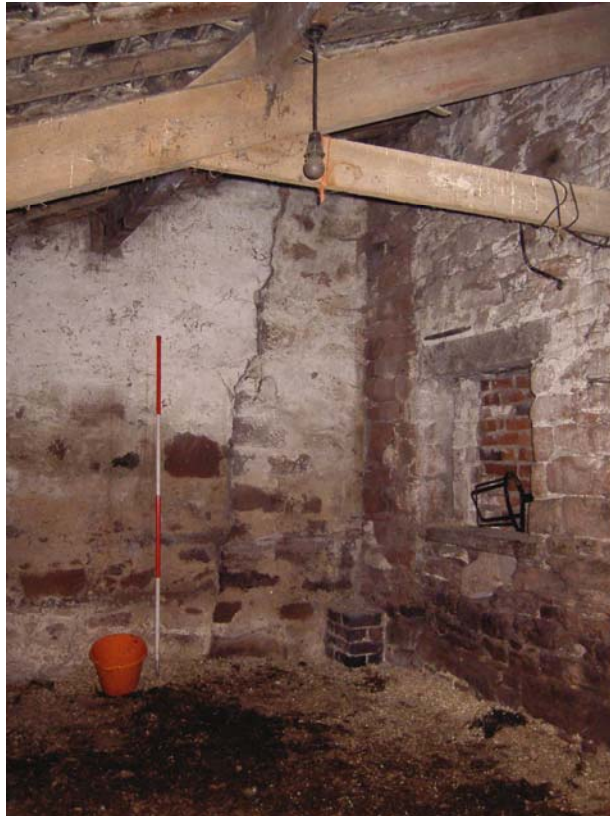
Plate 53: Buttress incorporated into the north elevation of the north-west outshut attached to the barn
