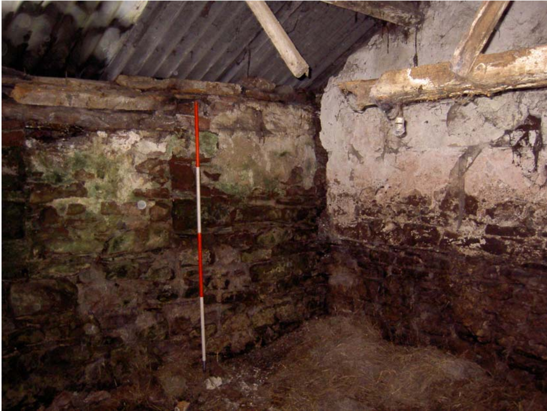
Plate 35: General view of the south-east corner of Room 2 of the dairy showing the blocked window, the butt joint between the south and east walls, and the truss
