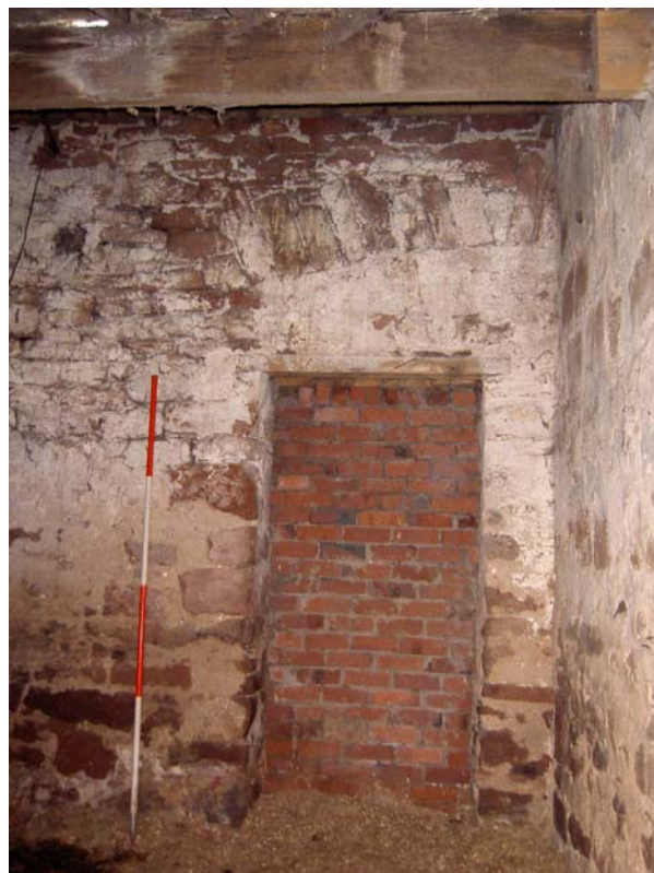
Plate 54: North side of the blocked wagon doorway in the east elevation within the north-west outshut attached to the barn
