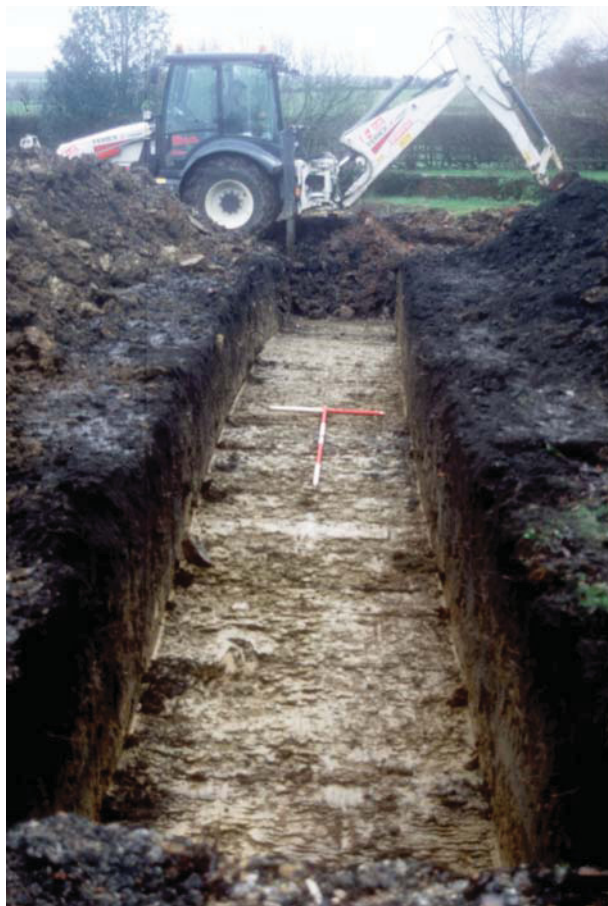
Plate 2: Trench 2, looking south.
