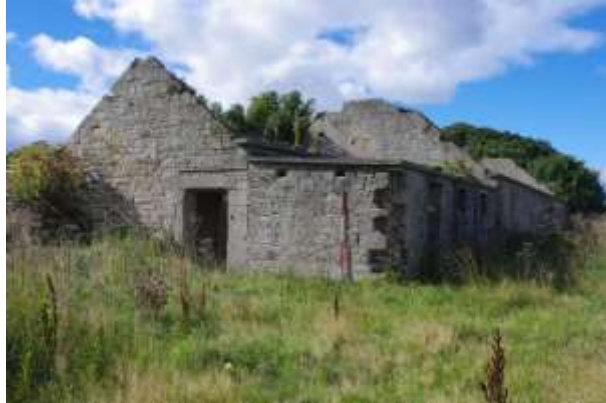
The Detached Byre Range from the north-east
