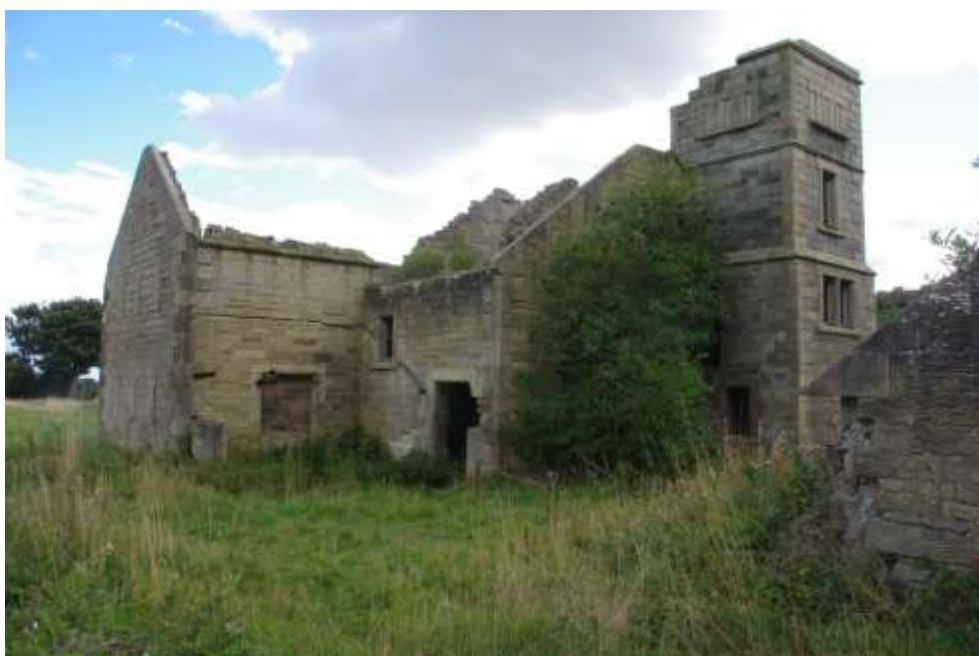
The Dovecote/Chimney and Engine House (with Barn beyond) from the north-west
