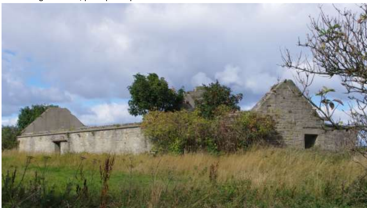
The Detached Byre range from the south-east
