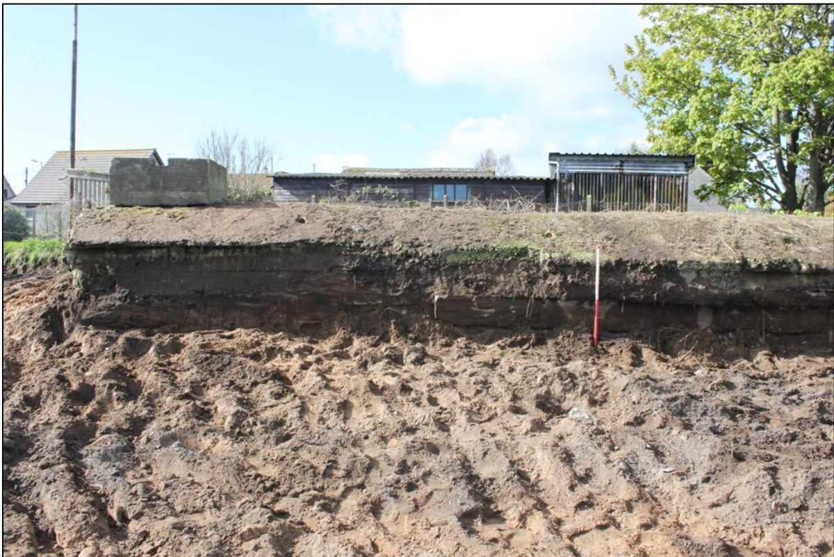
Figure 6b: Structure (001) demonstrating the sequential pouring with the roof capping the body of the Air0raid shelter.
