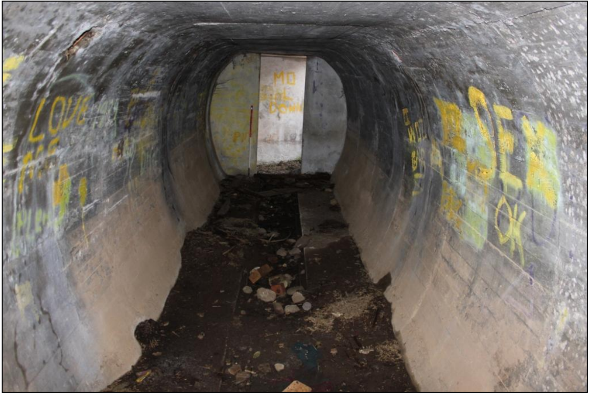
Figure 9a: Room B looking west demonstrating the internal form, graffiti , ceramic air vent in the top left of the image and access from Room A
