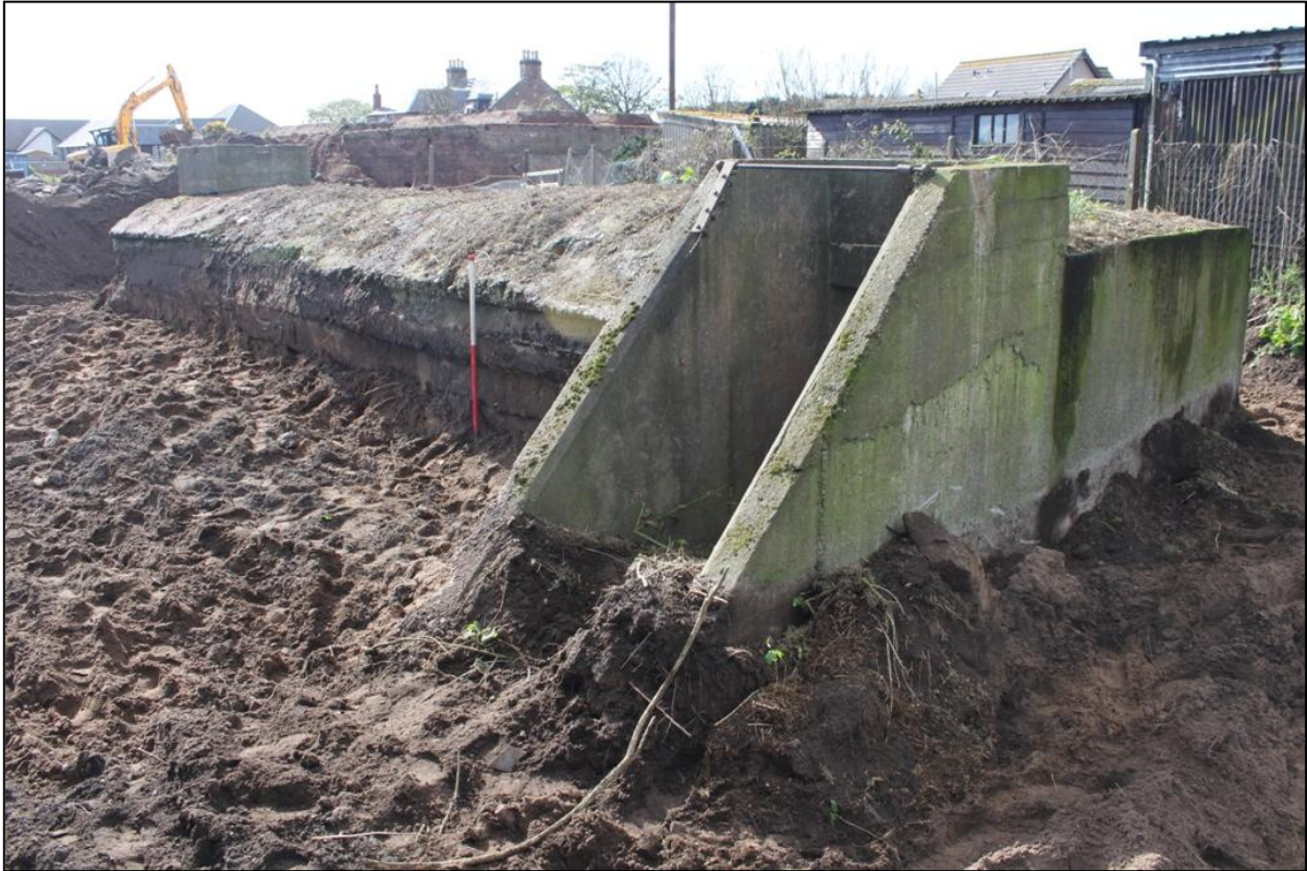
Figure 6a: Structure (001) showing the north facing elevation with main access located at the western end and the access hatch protective surrounding at the eastern end
