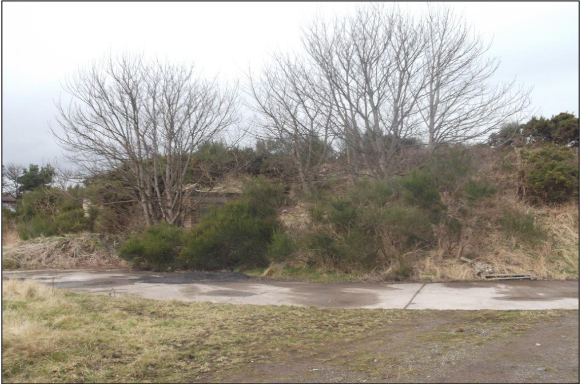
Figure 5a: Structure 003 (Fuel Bunker) demonstrating the thick vegetation and covering mound with the surrounding sectional poured concrete roadway in the foreground
