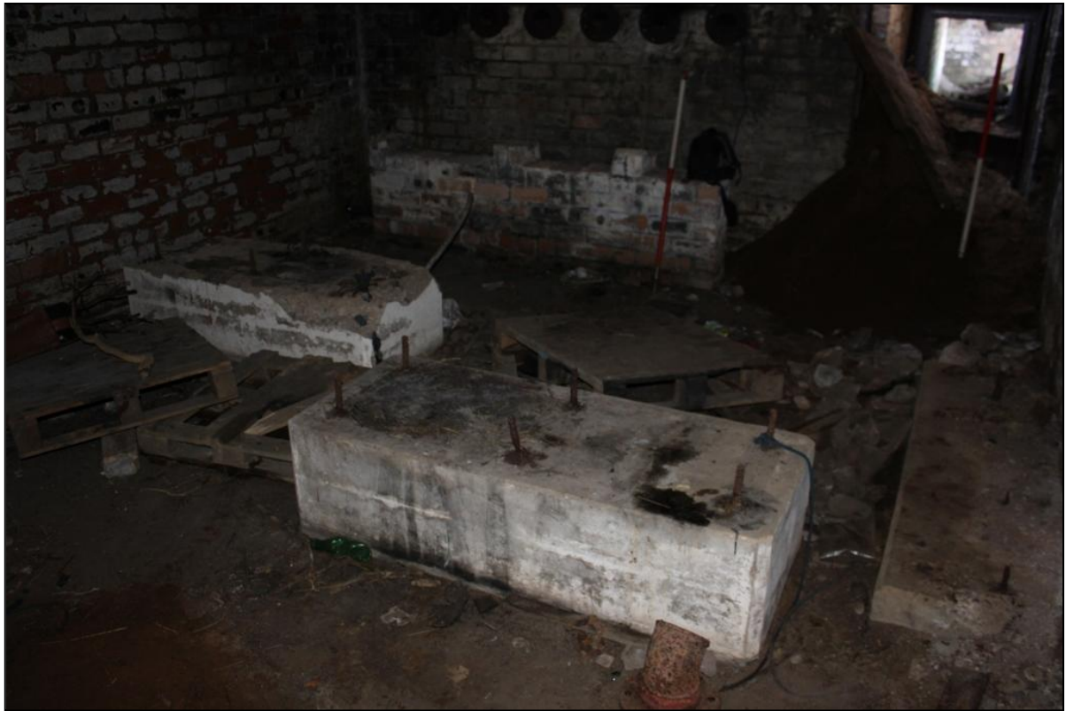
Figure 11a: Concrete plinths (details ii & iii) also demonstrating the metal fixings
