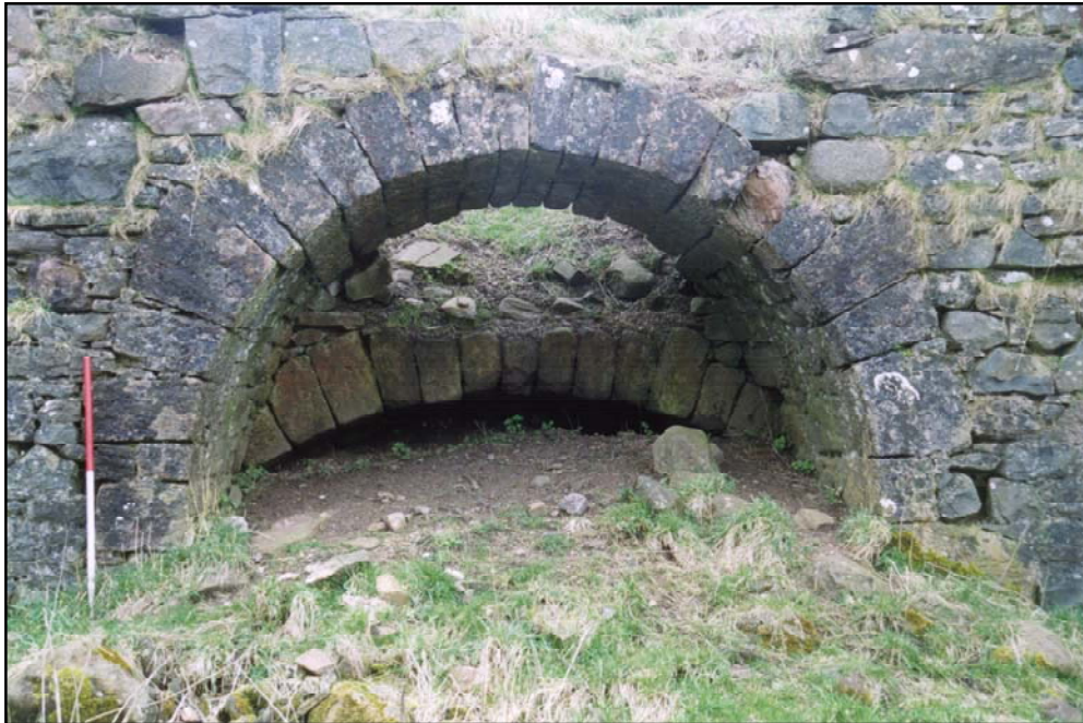
Figure 3b: Double relieving arch of Lime Kiln
