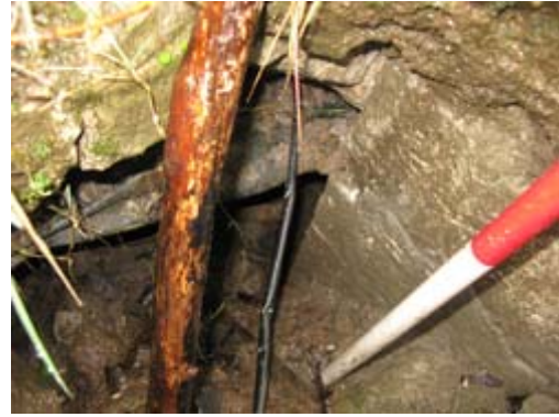
Fig.5.2: Inside the Vault
