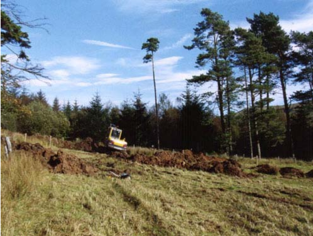
Figure 2a: Site seen from the west
