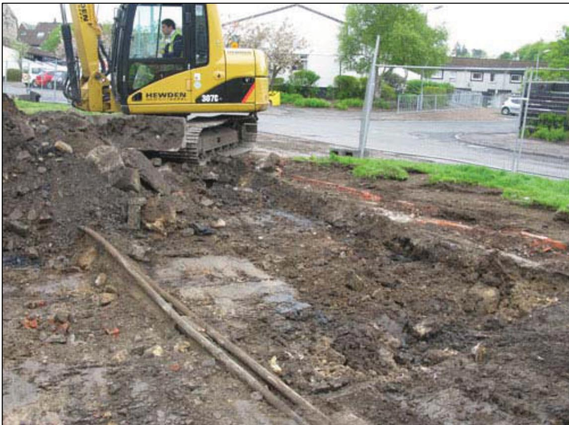
Figure 4b: Gas services exposed at south end
