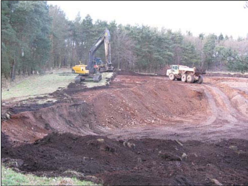
Figure 4a: Work in Progress
