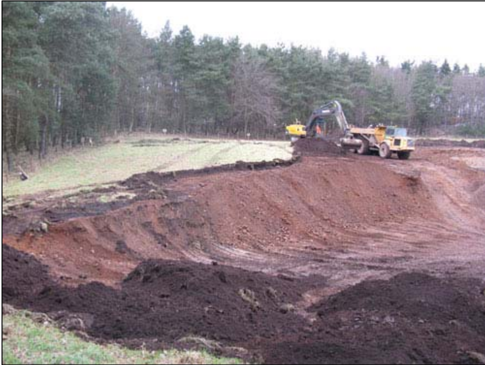
Figure 3a: Work in Progress
