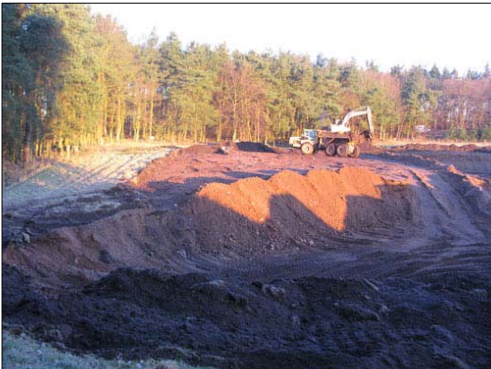
Figure 4b: Work in Progress
