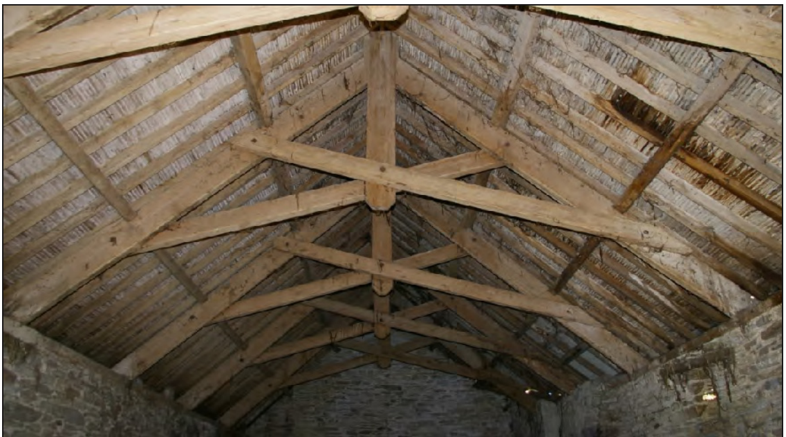
Figure 34: Roof structure of the Shippon, viewed from the west.
