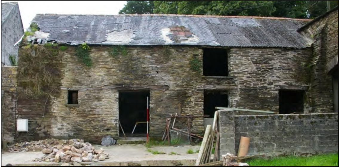
Figure 27: North elevation of the Stables, viewed from the north (scale 2m).
