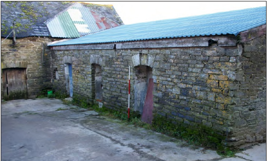
Figure 31: West elevation of Milking Parlour, viewed from the south-west (scale 2m).
