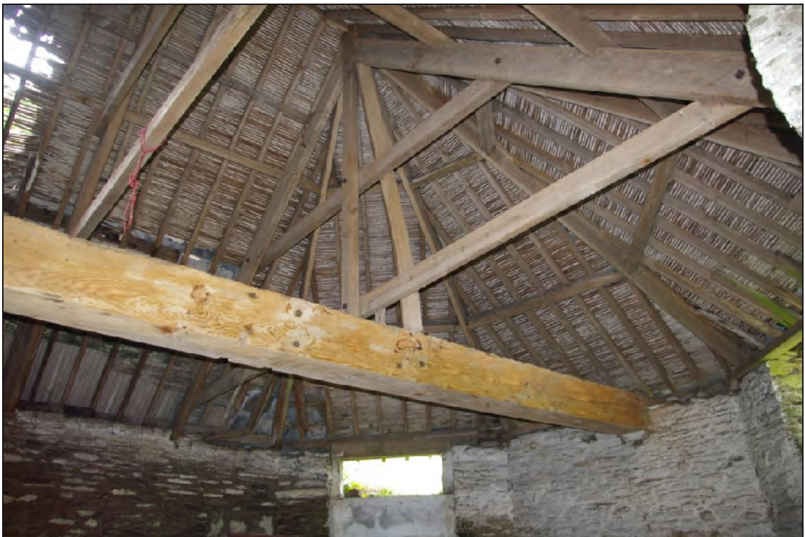
Figure 30: The interior of the Horse Engine House, viewed from the north-east.
