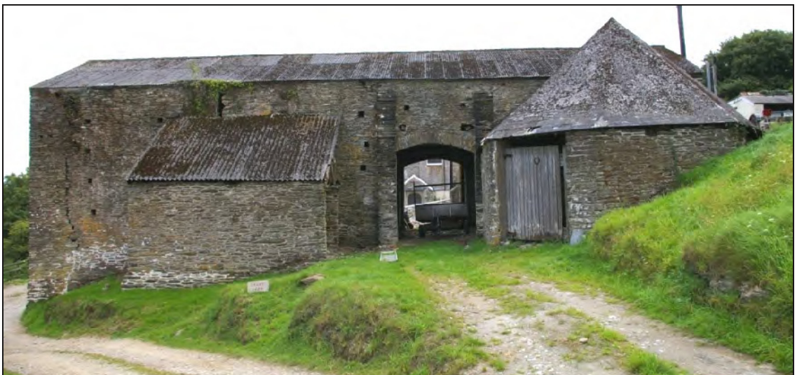
Figure 18: West elevation of the Great Barn, viewed from the west.
