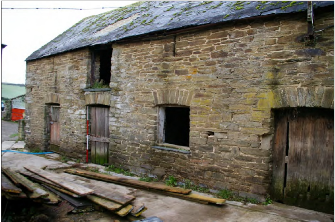
Figure 32: South elevation of the Shippon, viewed from the south-east (scale 2m).
