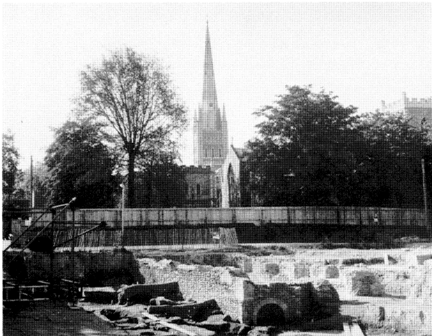
A. ST MARTIN-AT-PALACE PLAIN, NORWICH, NORFOLK 12th-century building from NE
