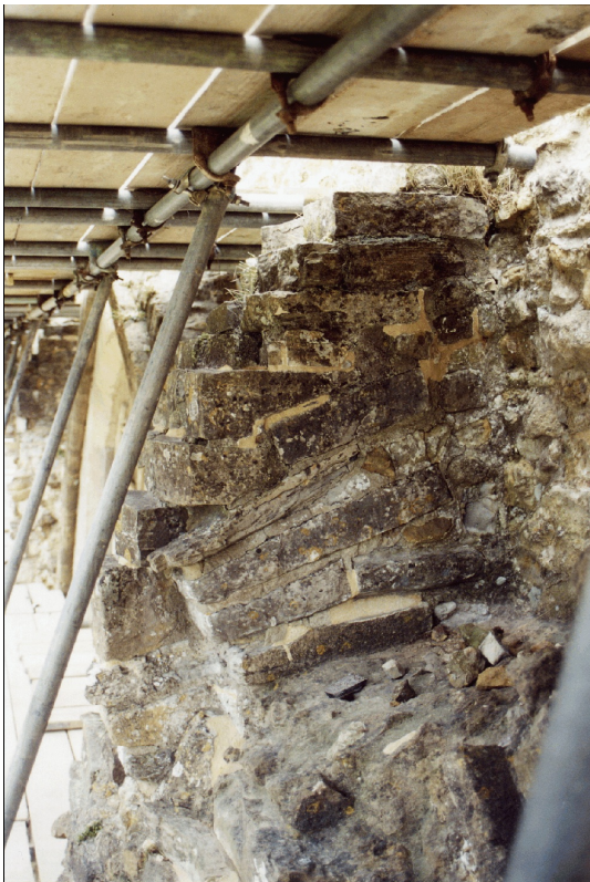
Above left: the late twelfth or early thirteenth century vaulting springer of Bay 4/5 looking South-East, showing the apparently vertical rise of the transverse rib.
