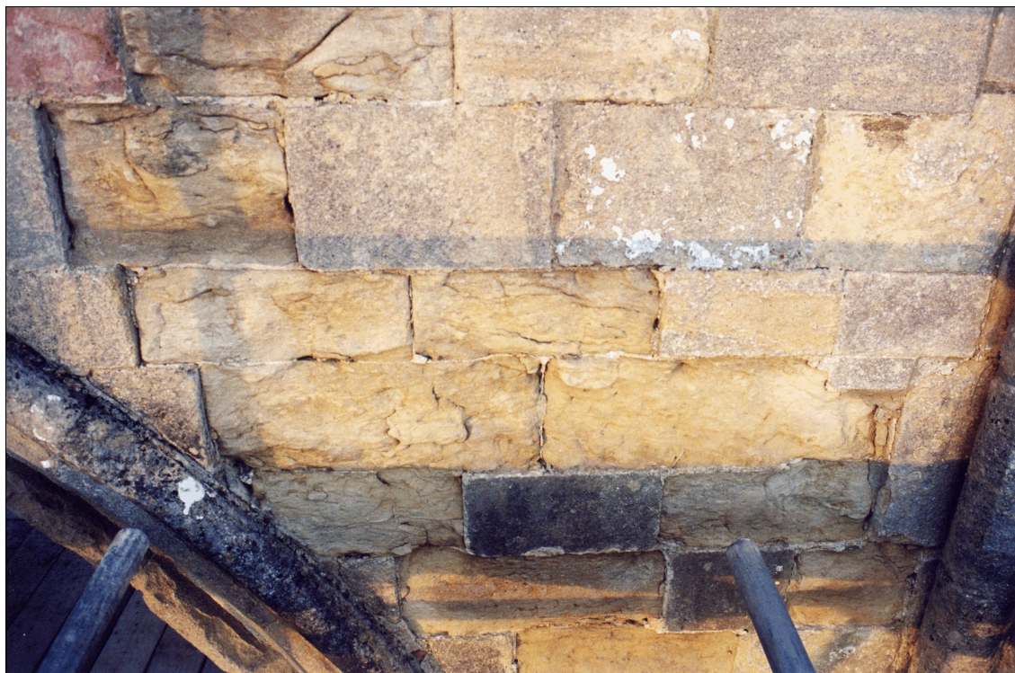
Above: Upper lias ashlars in the eastern spandrel of Bay 6. Much of the Douling stone at the top of the wall is repair dating from 1912. Note the burnt block at upper left.
