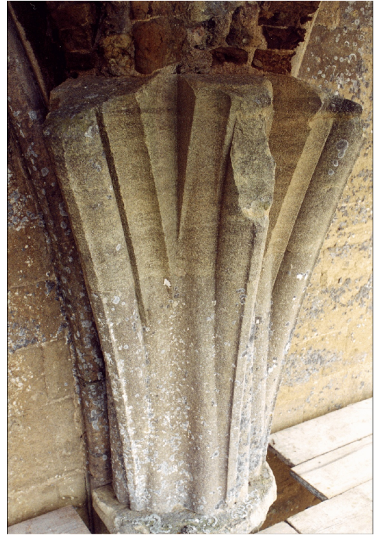
Above left: the late twelfth or early thirteenth century vaulting springer of Bay 4/5 looking South-East, showing the apparently vertical rise of the transverse rib.
