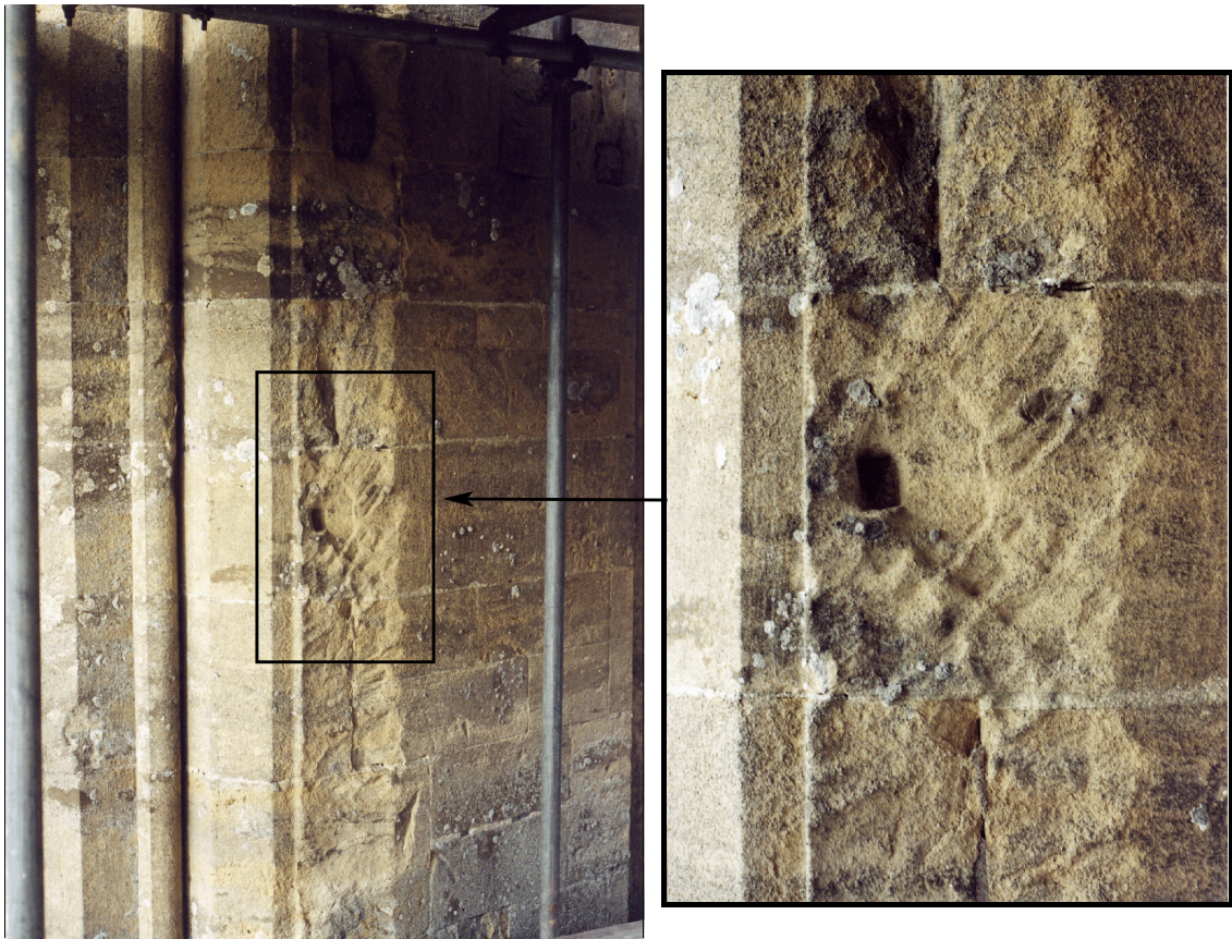
The chamfered face of the C12/13 window jamb cut away to accommodate the inserted tracery of the C14/15 windows, the inset showing both the roughly tooled surface and one of the sockets for the saddle-bars. Below: vertical tooling on the upper part of the wall.
