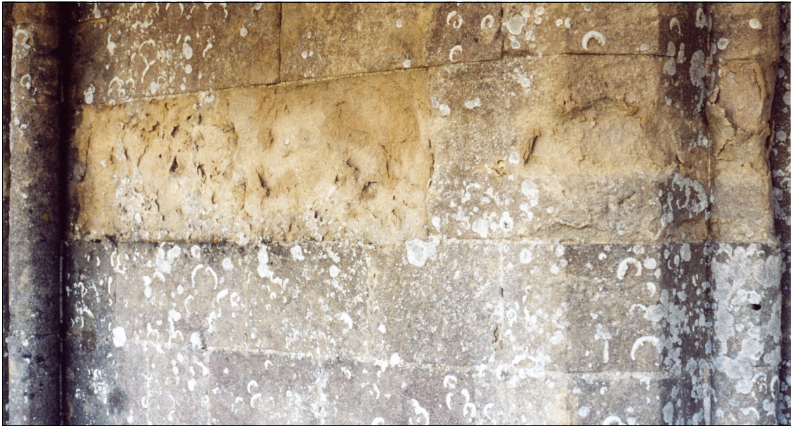
Above: decay along the interface between the Phase 1 and Phase 2 fabric - possibly the result of the extreme carbonation of the lime mortar core of the head of the Phase 1 wall
