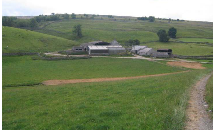
Figure 14: Beecroft Hall, an unoccupied farmhouse that is the closest property in Horton to the quarry, just 175m from the quarry perimeter. Although the property is listed, it has fallen into disrepair due to the covenant placed on it that prohibits inhabitation. On initial inspection of the property and the surrounding land deposits of dust were observed.
