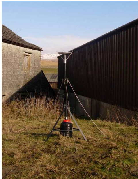
Figure 33: Frisbee Gauge deployed at Beecroft Hall, Horton in Ribblesdale, winter 2006.
