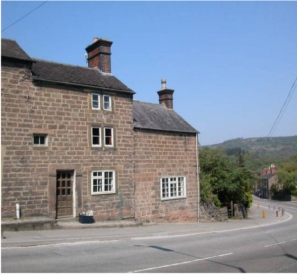
Figure 11: 54 Cromford Hill. Located on the west side half way down Cromford Hill. This is the nearest property to Dene Quarry (350m from the quarry perimeter), with the rear of the property facing the quarry.
