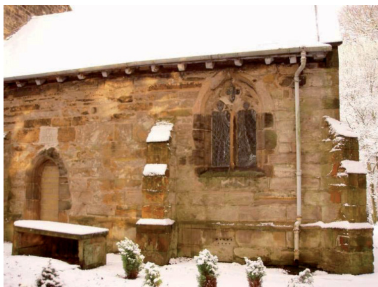
Plate 6: The southern side of the chancel
