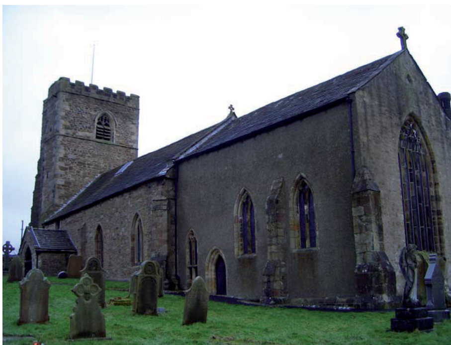
Plate 34: Southern side of All Hallows Church at Mitton, demonstrating the use of nave walls that sit lower than those of the chancel
