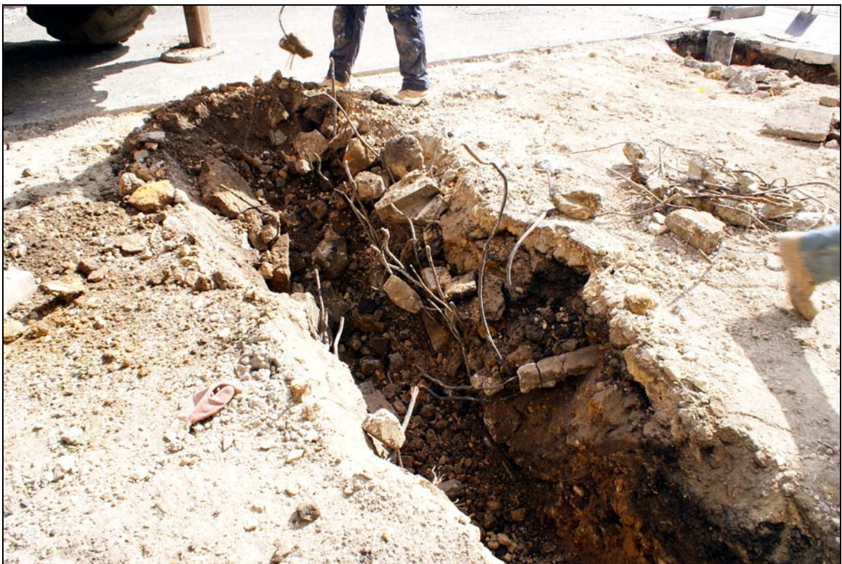
Plate 4: General view of air-raid shelter remains [253] - looking south
