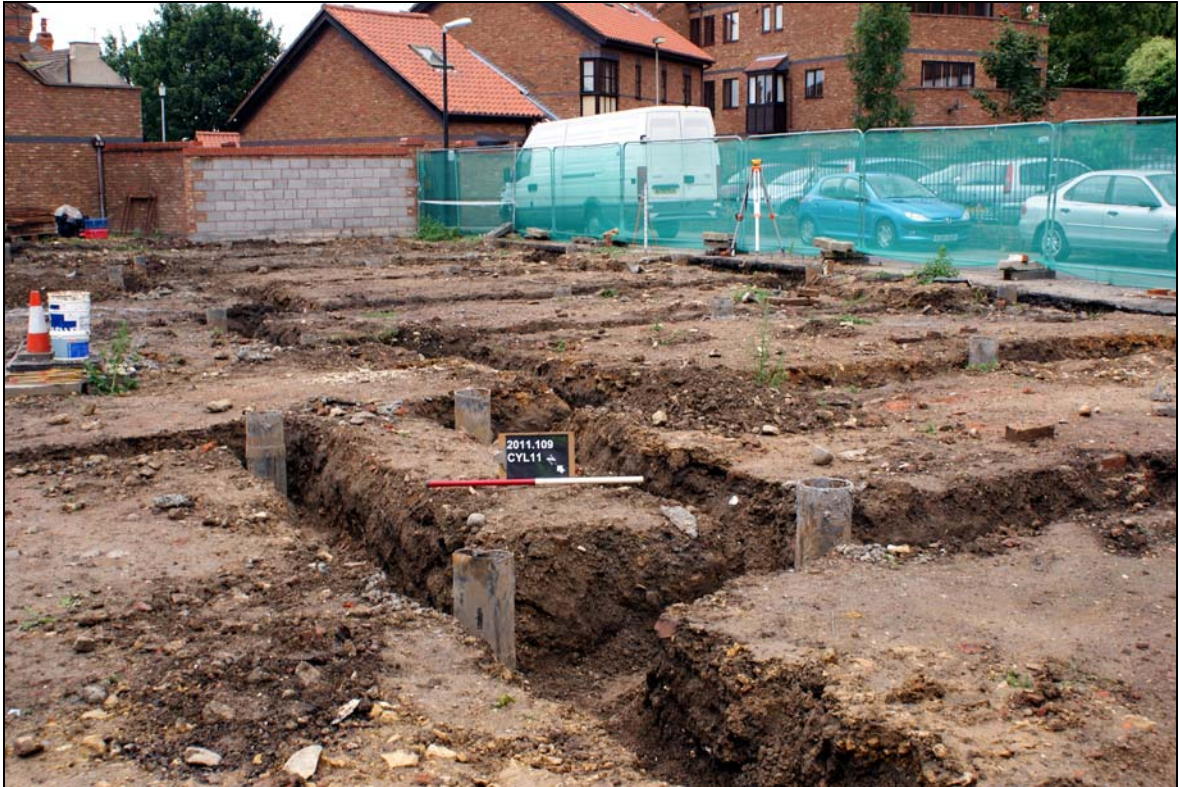
Plate 3: General view of completed foundation trenching for Plots 5-11 - looking north-east
