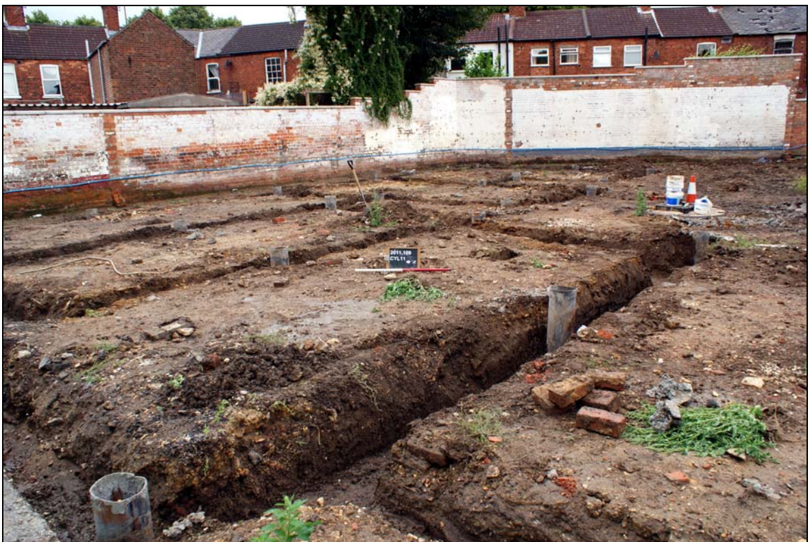
Plate 2: General view of completed foundation trenching for Plots 10-14 - looking south-west
