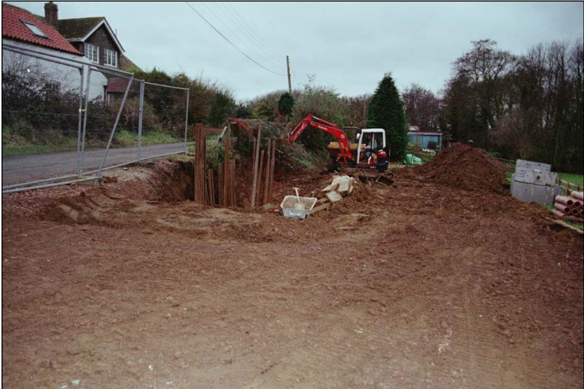
Plate 3: General view showing trenching for main sewer diversion in progress - looking west
