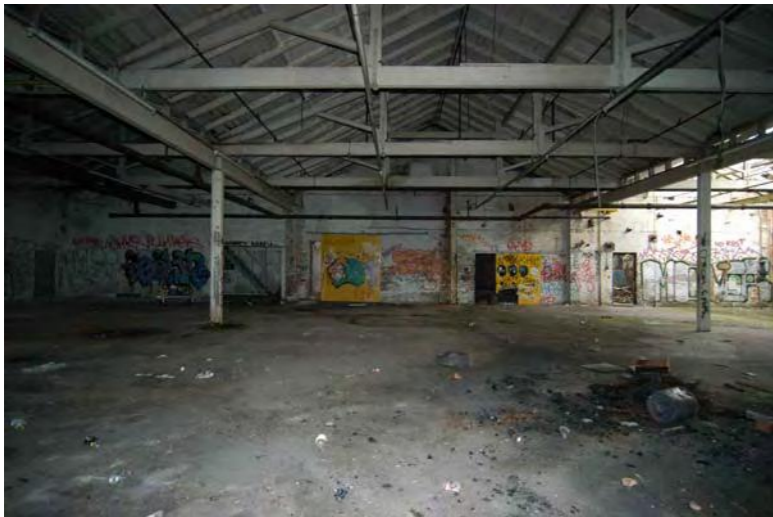
Plate 4 Unit 33 No.2 Shop, interior view. Central bay with queen post roof
