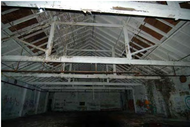
Plate 1 No.5 Shop, interior view. Central bay with queen post roof
