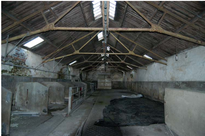
Plate 45: Interior shot of the calving shed (Building 4) showing composite iron roof joists
