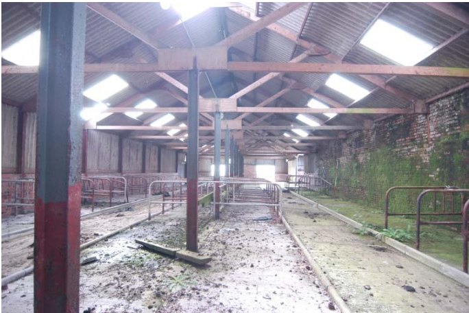
Plate 10: Interior of Building 4 showing its steel and timber framed construction
