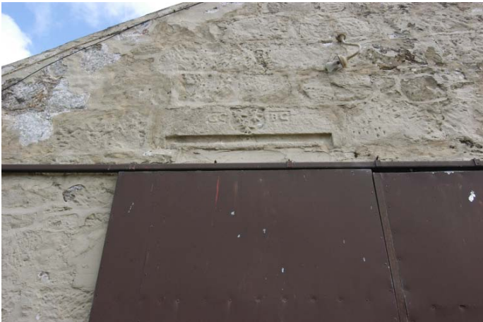
Plate 40: Fabric detail and re-used lintel with carved initials and heraldic plaque on the north-west facing gable (Building 4)
