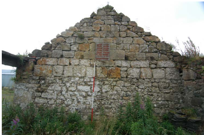
Plate 25: Interior north-facing partition wall between Units 2 and 3 in Building 8 showing droved surrounds around the blocked window and evidence of gable heightening
