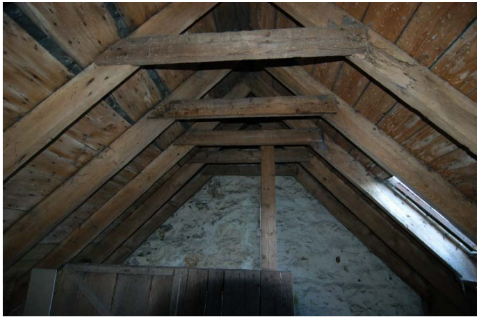
Plate 44: A-frame trusses within the loft above the former cart shed (Building 4)
