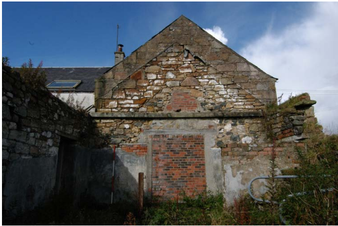
Plate 7: Interior of the byre (Building 3) with two phases of roofline on the farmhouse gable
