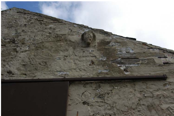
Plate 41: Fabric detail and evidence of wall heightening with a carved face and five carved lintels or sills on the north-west facing gable of Building 4
