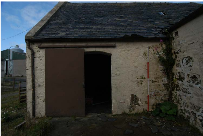
Plate 42: Exterior of south-east facing return wall of Building 4 showing part blocked cart shed openings
