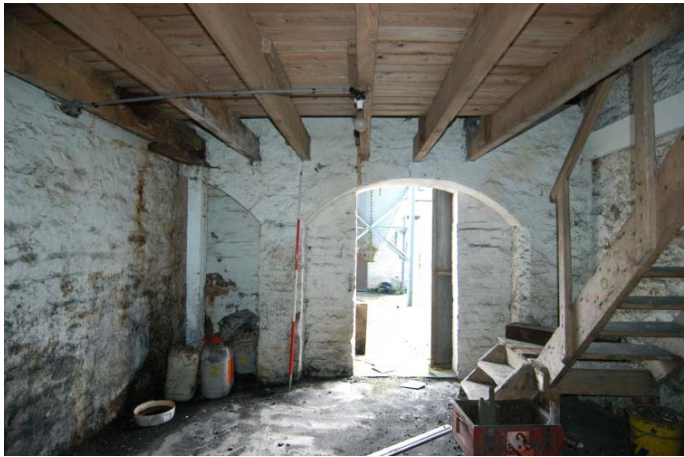
Plate 43: Interior north-west facing elevation showing the arched openings of the former cart shed (Building 4)
