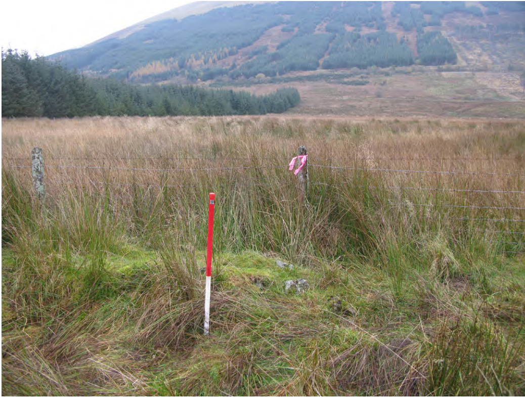
Fig. 6 Drystone wall where it will be crossed by the footpath
