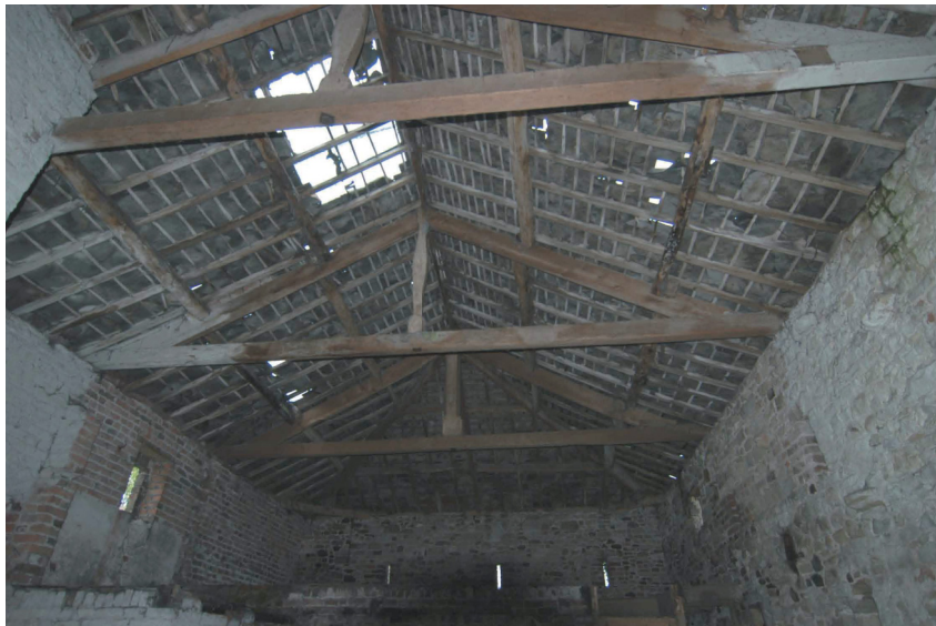
Plate 11 - General view of the A-frame roof structure
