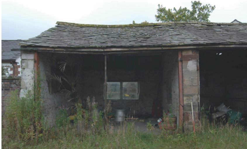
Plate 5 - East range gable and boundary wall
