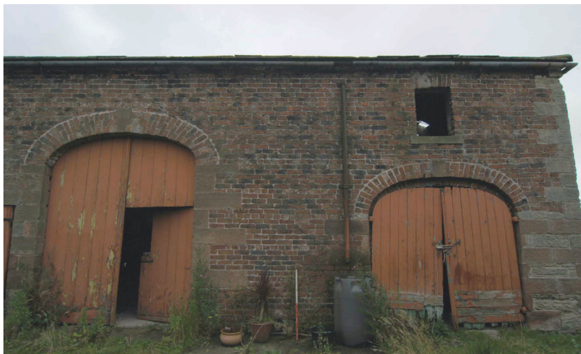
Plate 3 - Close-up of the two arched barn doorways
