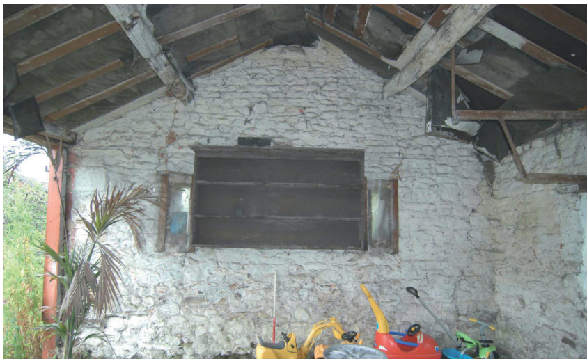
Plate 6 - Interior shot of Unit H
