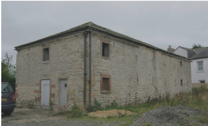
Plate 2 - General view of the west-facing elevation and barn gable
