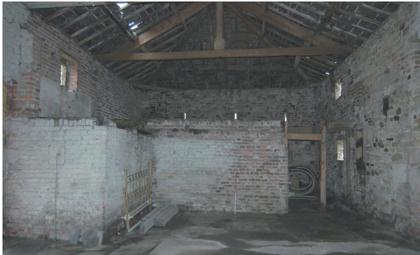
Plate 8 - Interior of the barn looking south
