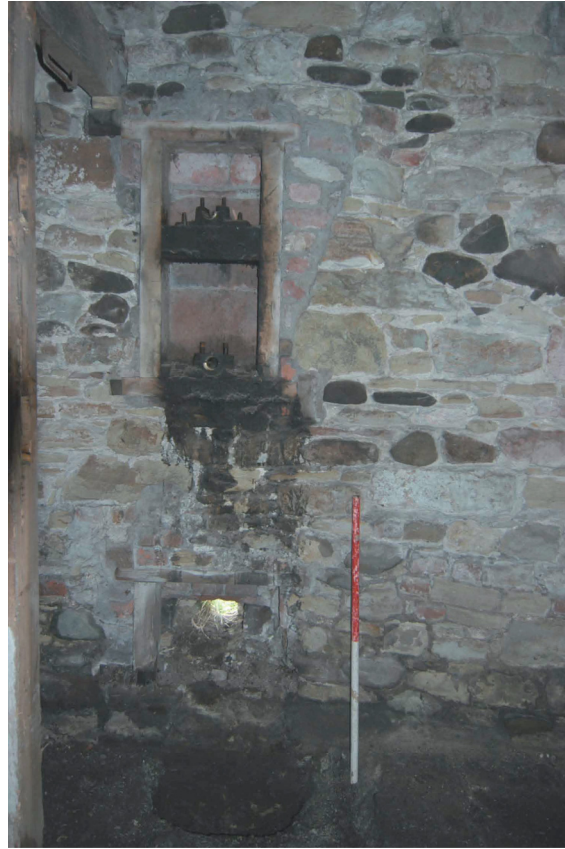
Plate 10 - Oil stained bearing plate inserted in the barn wall
