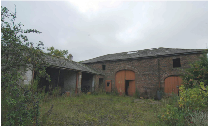
Plate 1 - General view of the east-facing elevation of the barn
