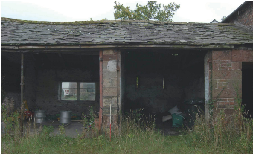
Plate 4 - General view of the garage doorways on the east range
