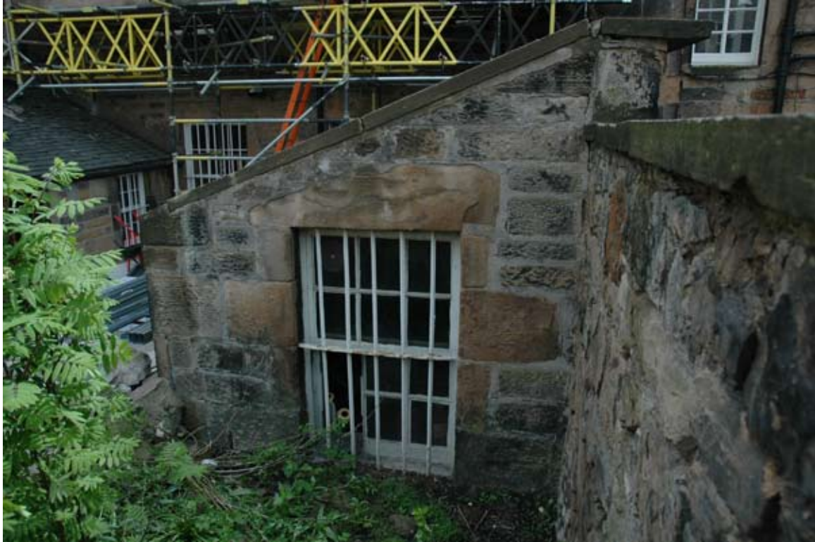
Fig 6. North elevation of lean-to
