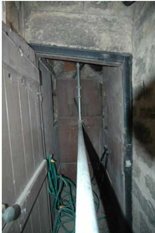
Fig 7 East elevation of shed
