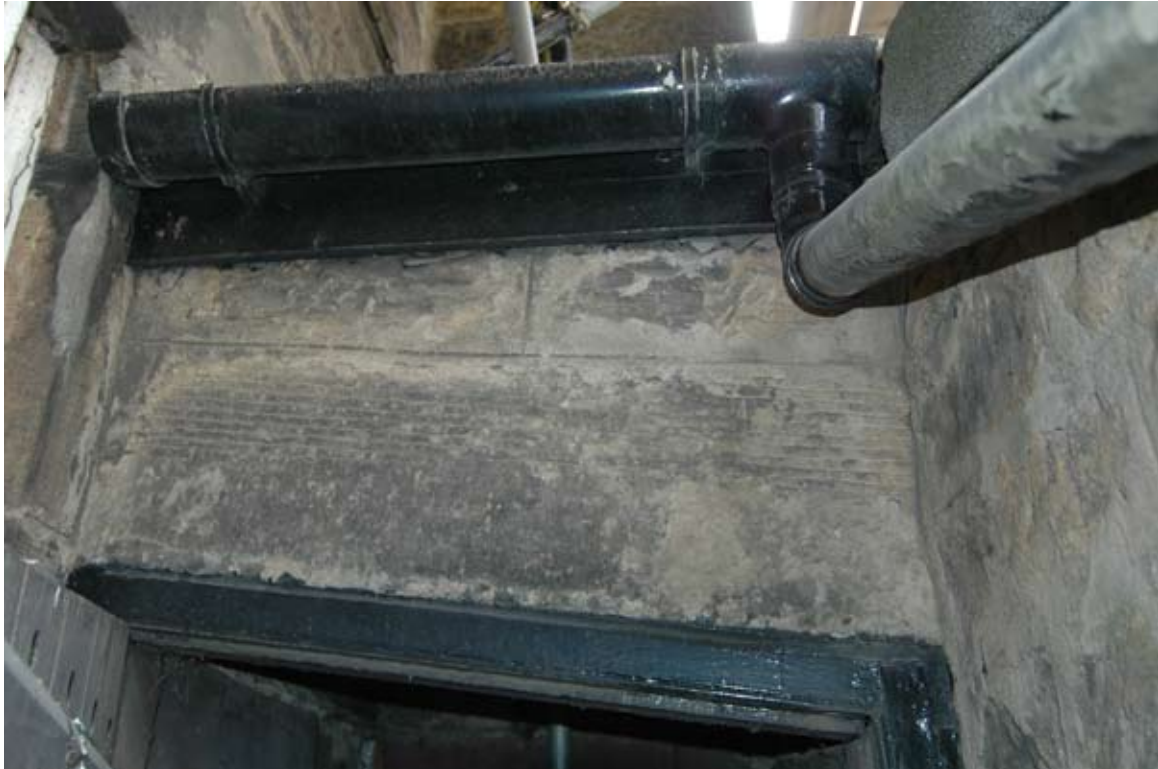
Fig 8. Detail of shed lintel
