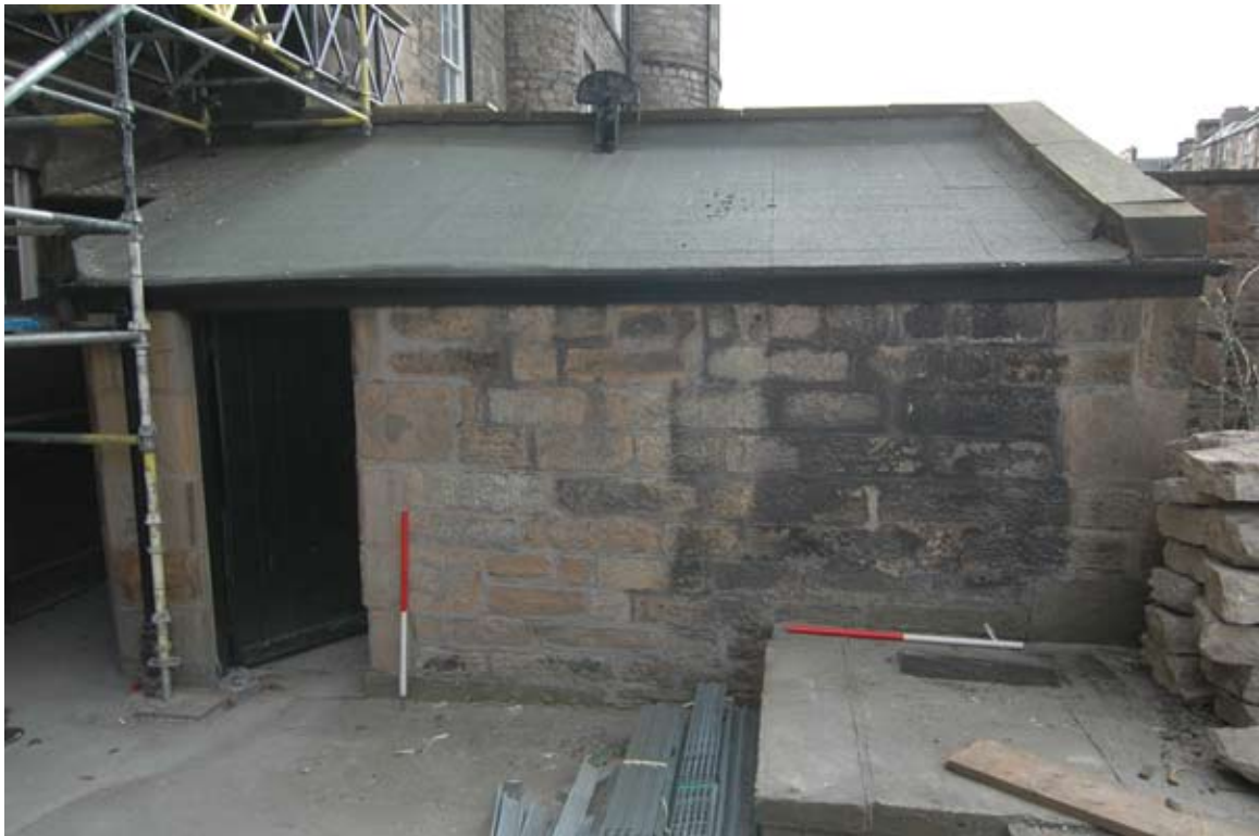
Fig 5. East elevation of lean-to
