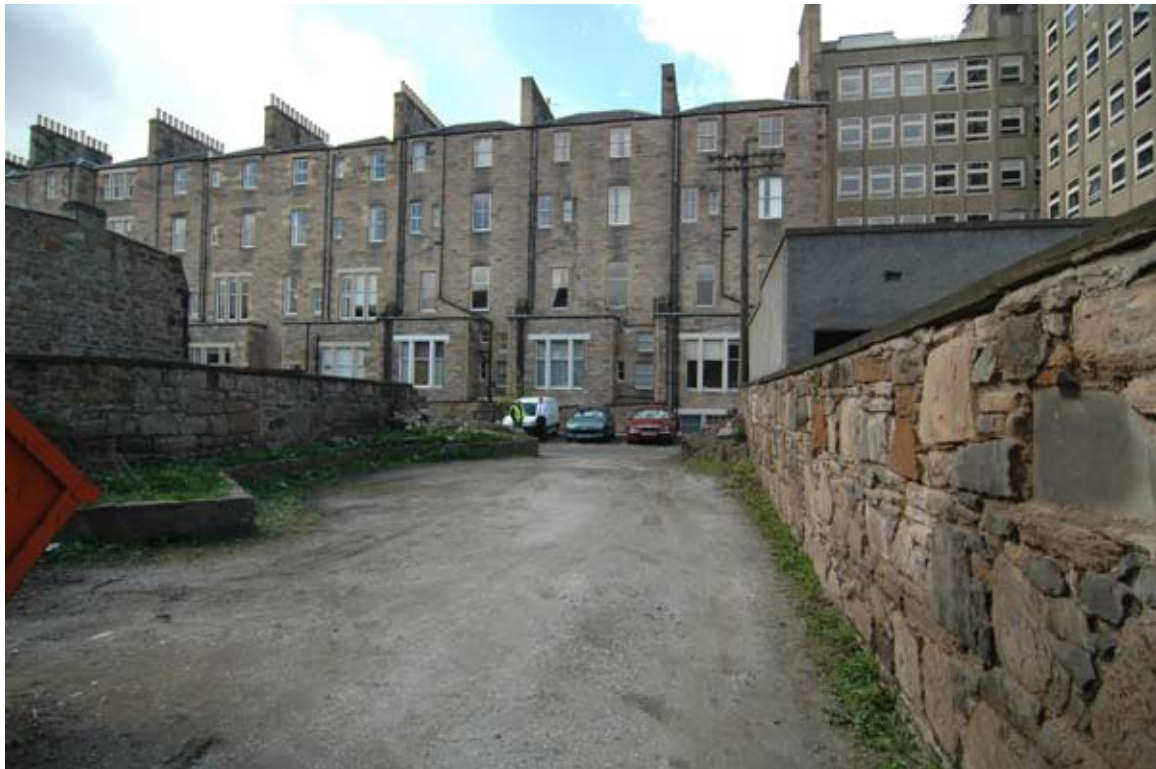
Fig 11. View of plot from rear of building
