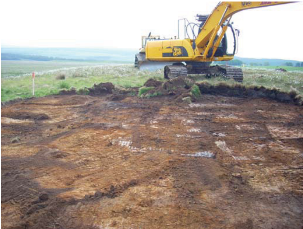
Fig. 3 General view of topsoil stripping for access tracks
