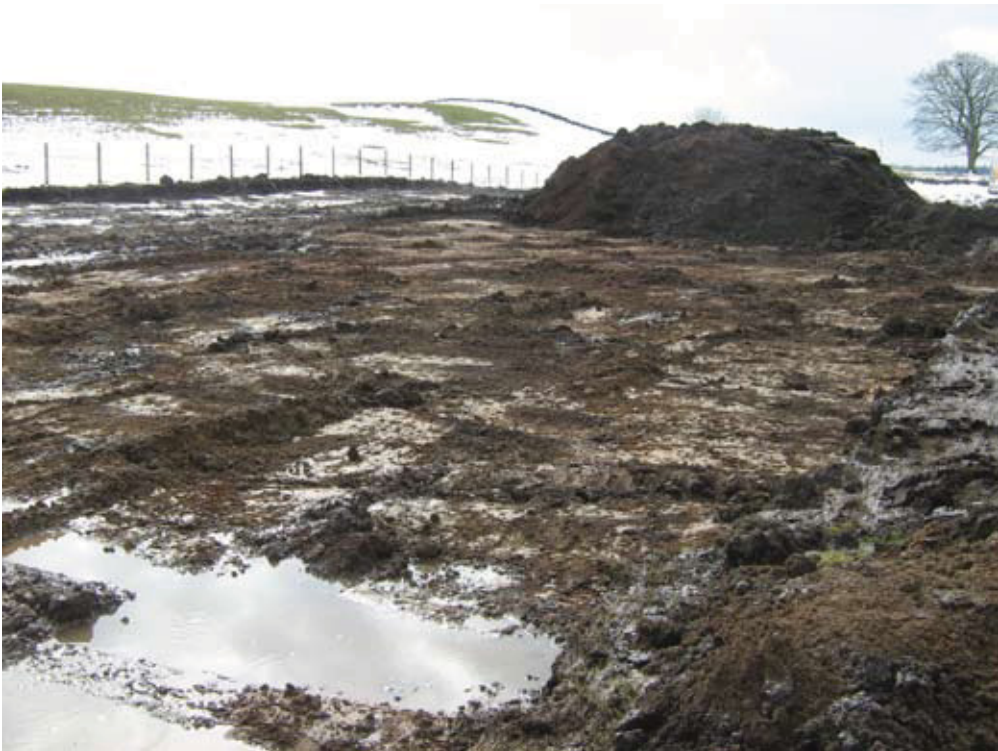
Fig. 2 Stripped area of site compound after topsoil removal
