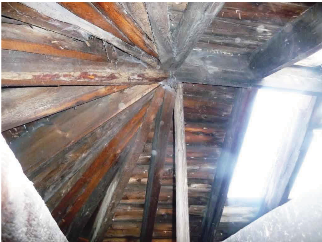
Figure 28: Detail of curved end roof truss (Photo courtesy of Richard Berry, 2009)
