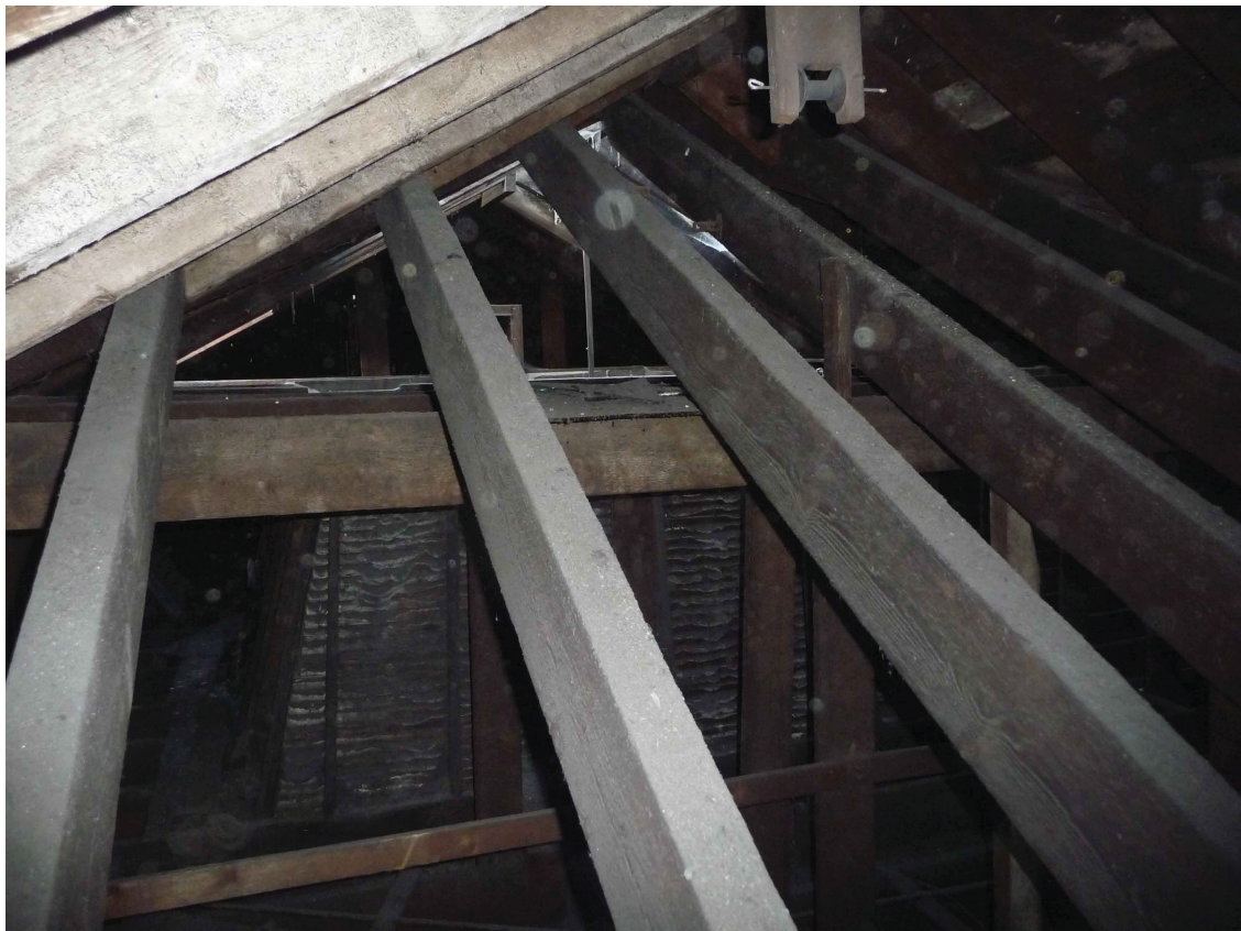
Figure 29: Detail of reinforcing truss (Photo courtesy of Richard Berry, 2009)
