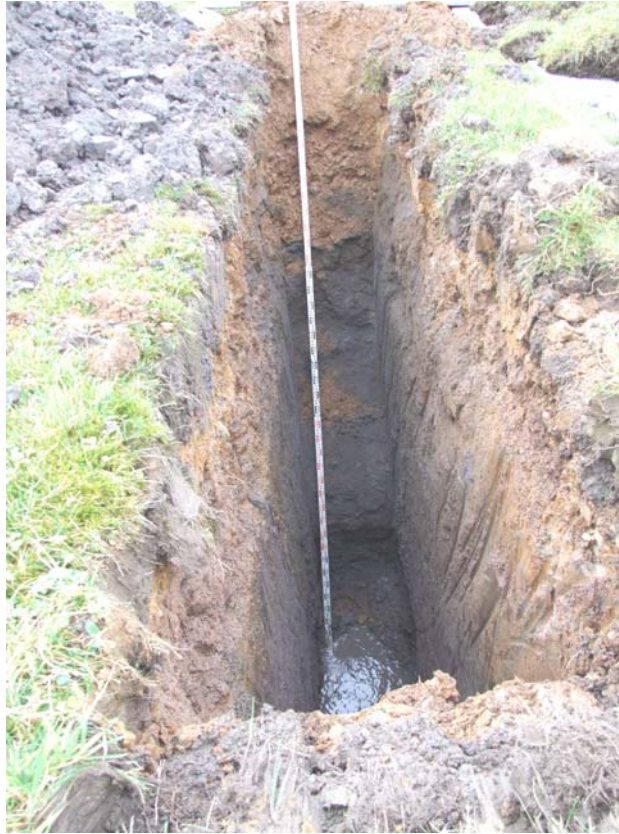
PLATE 3 Test Pit 04, looking north west.
