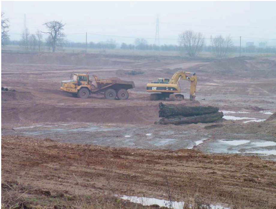
Fig 5.5: Photograph of the tree trunks from Warren Farm Quarry that were dendrochronologically dated.
