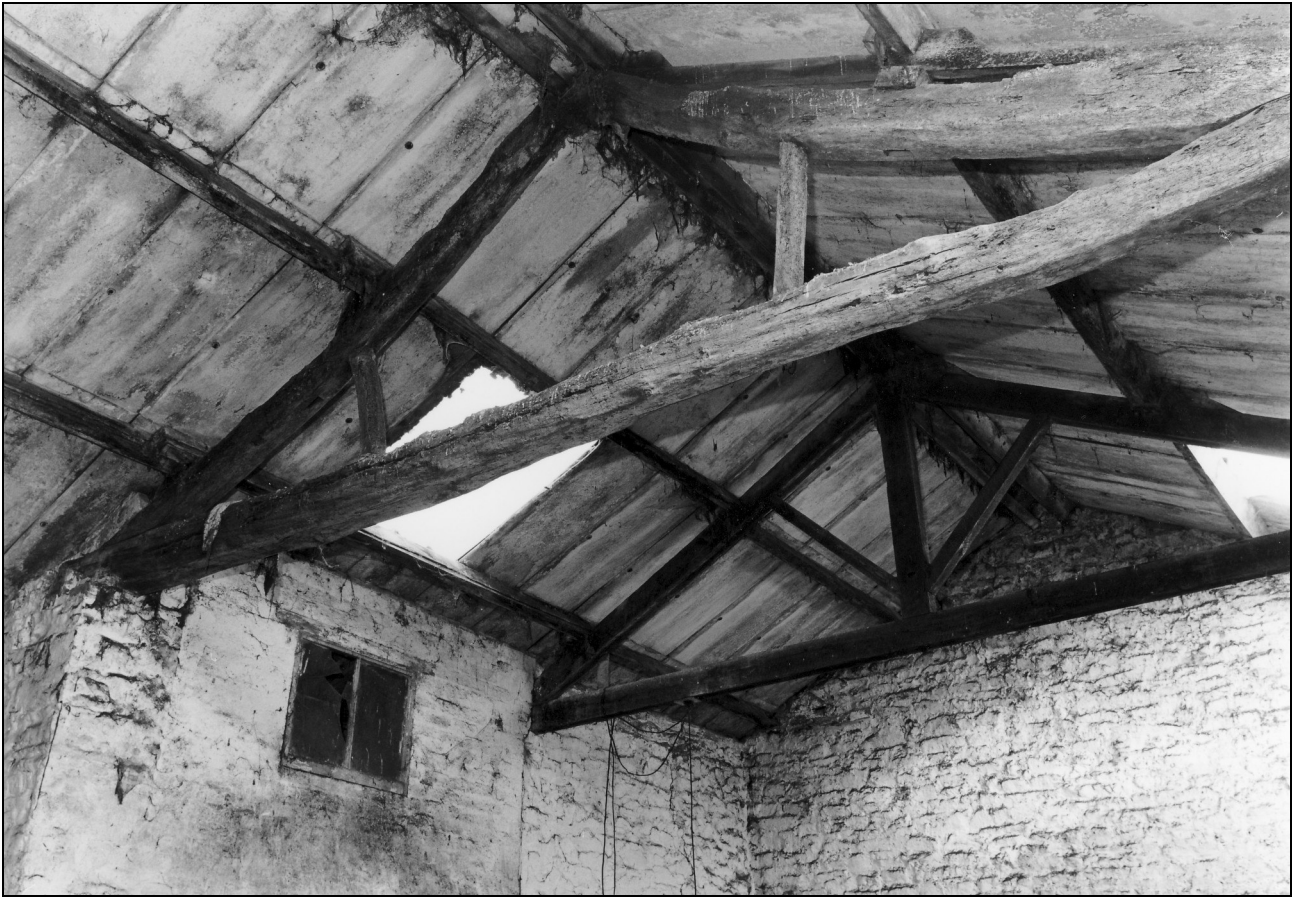
Photo 16: Earliest, central roof truss, from the south
