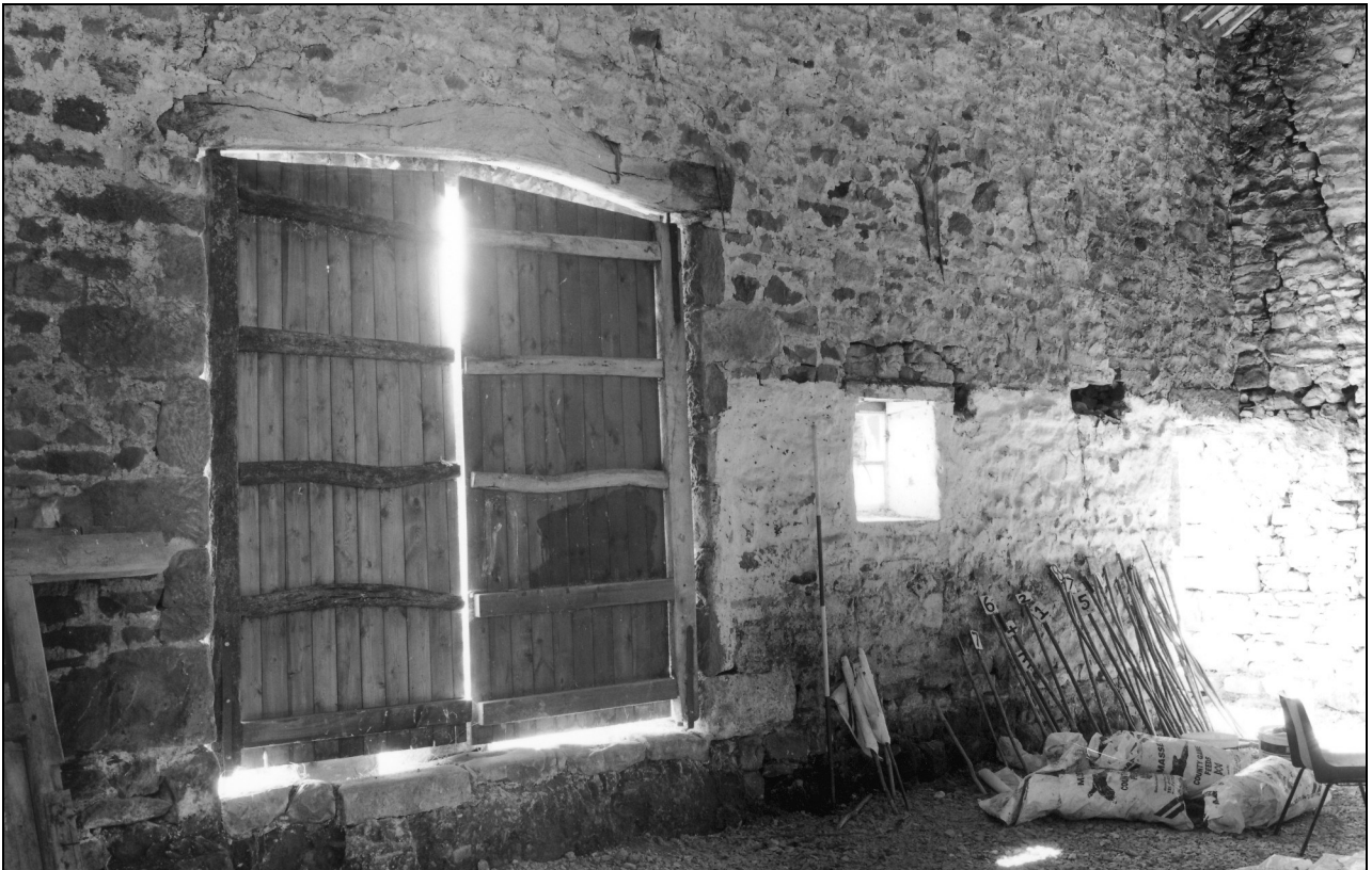
Photo 17: South-west corner of interior and main entrance
