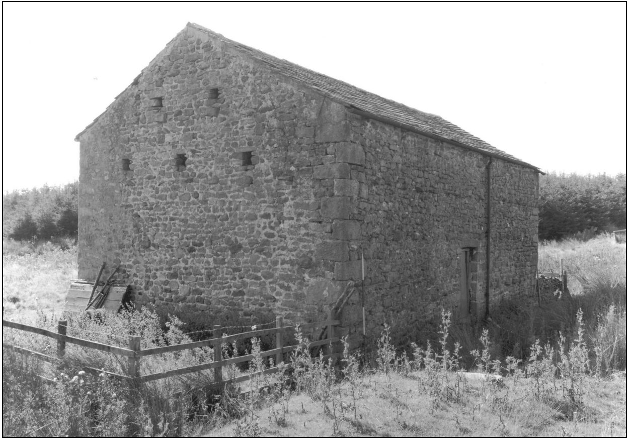
Photo 9: The barn, from the north
