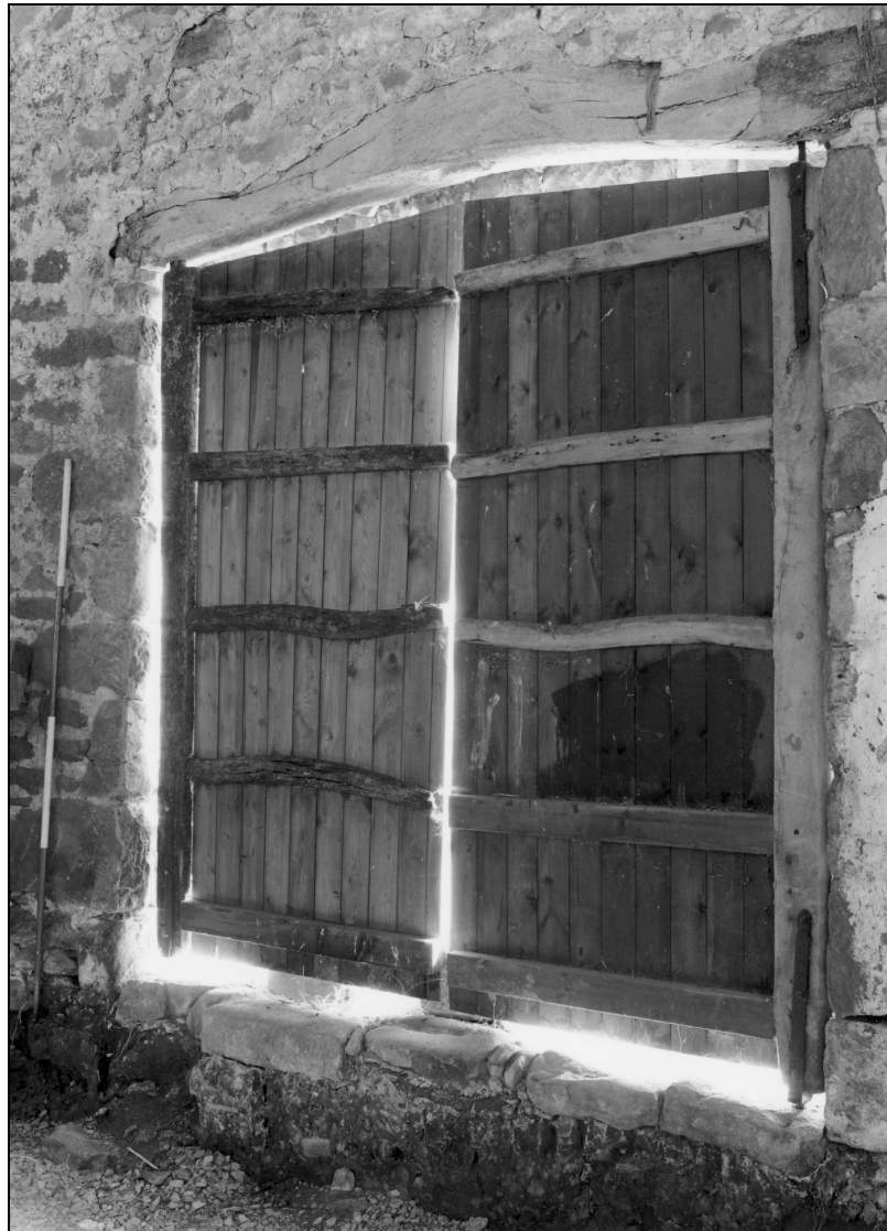
Photo 15: Detail of main doors, interior face, from the west
