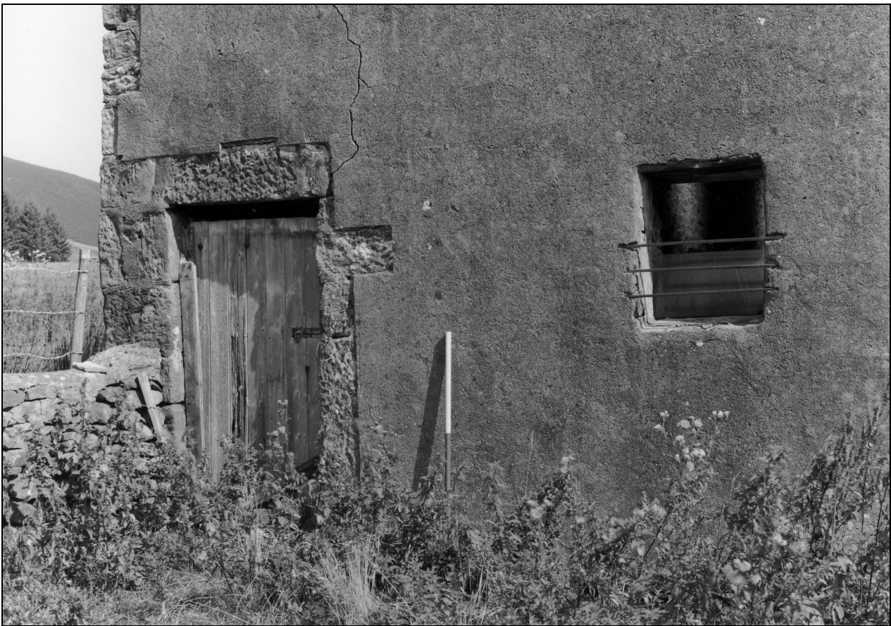
Photo 7: Detail of doorway and window in south-west gable
