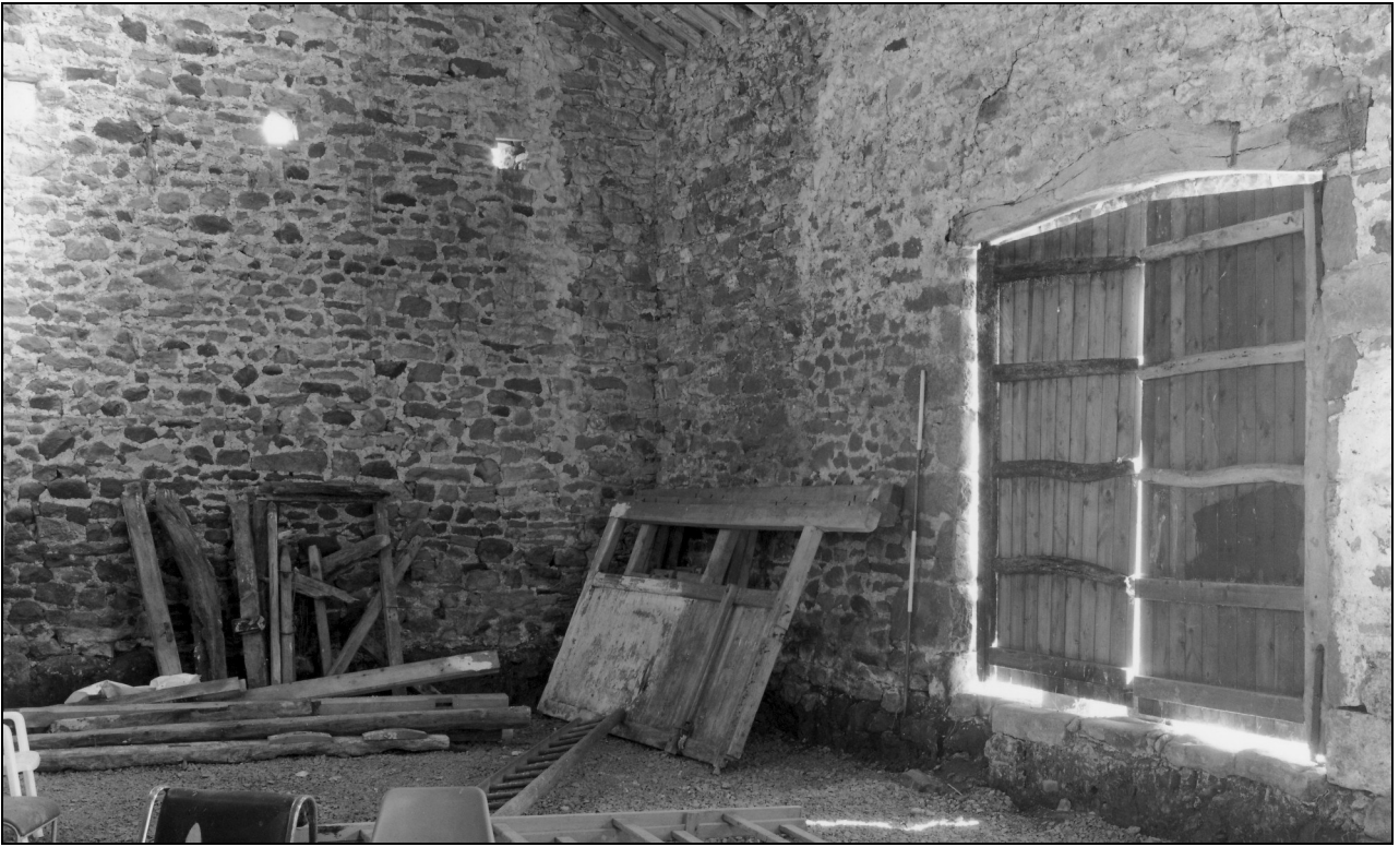
Photo 13: Interior of barn, from the west
