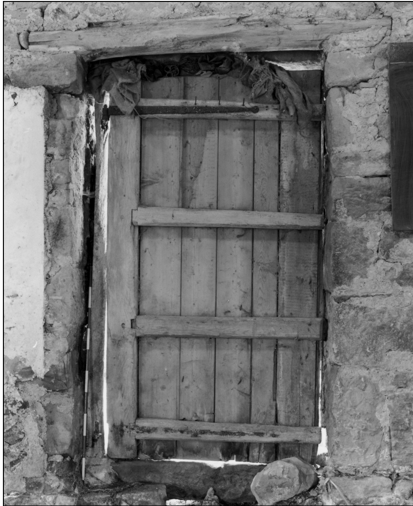
Photo 16: Detail of rear door, interior face
