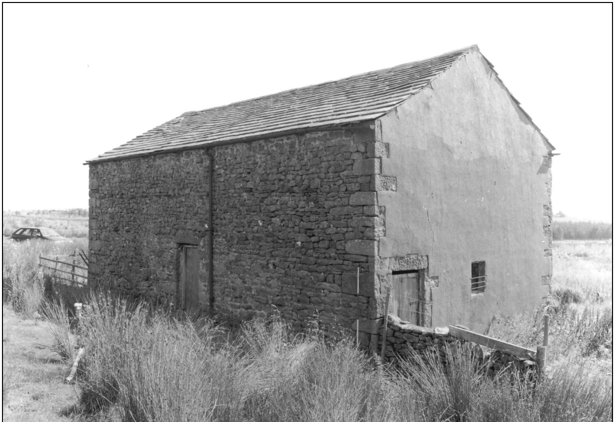
Photo 11: The barn, from the west
