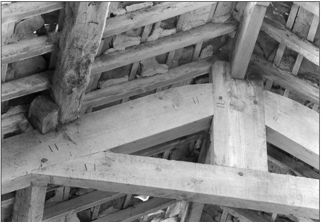
Photo 27: Detail of head of central truss, from the east
