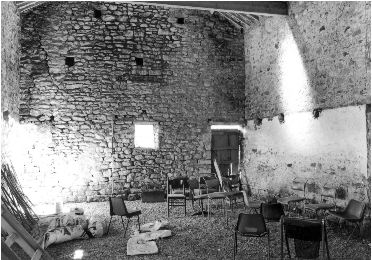
Photo 18: Interior of barn, from the east
