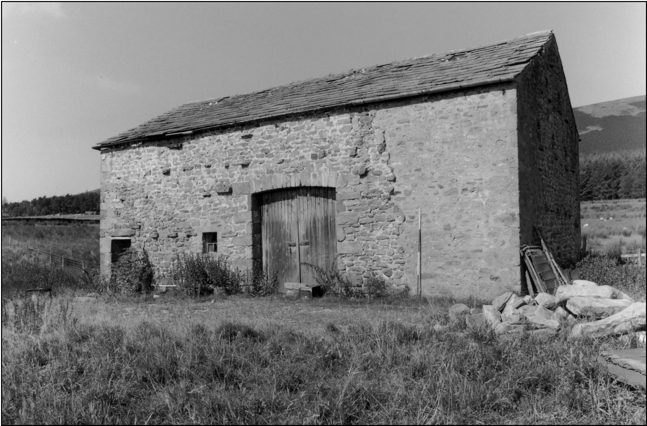
Photo 3: Front elevation, from the south-east
