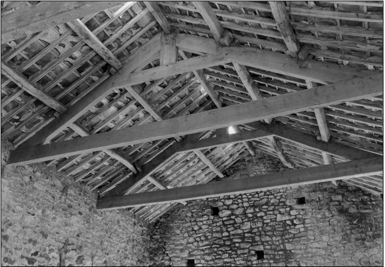
Photo 25: Central roof truss, from the north-east
