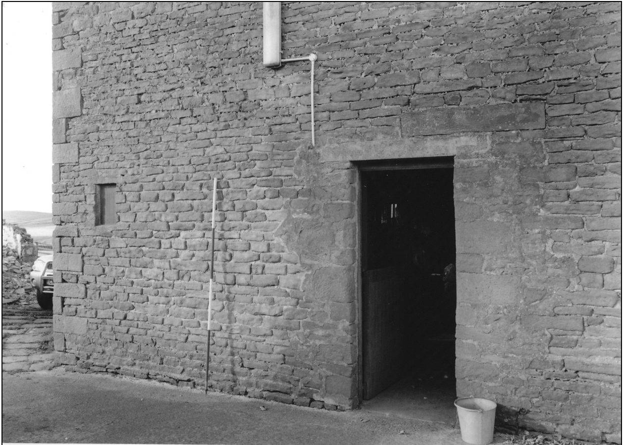
Photo 6: Inserted doorway to shippon in south elevation of barn
