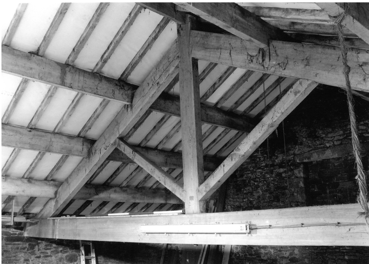
Photo 28: Roof truss in barn, from the north-east
