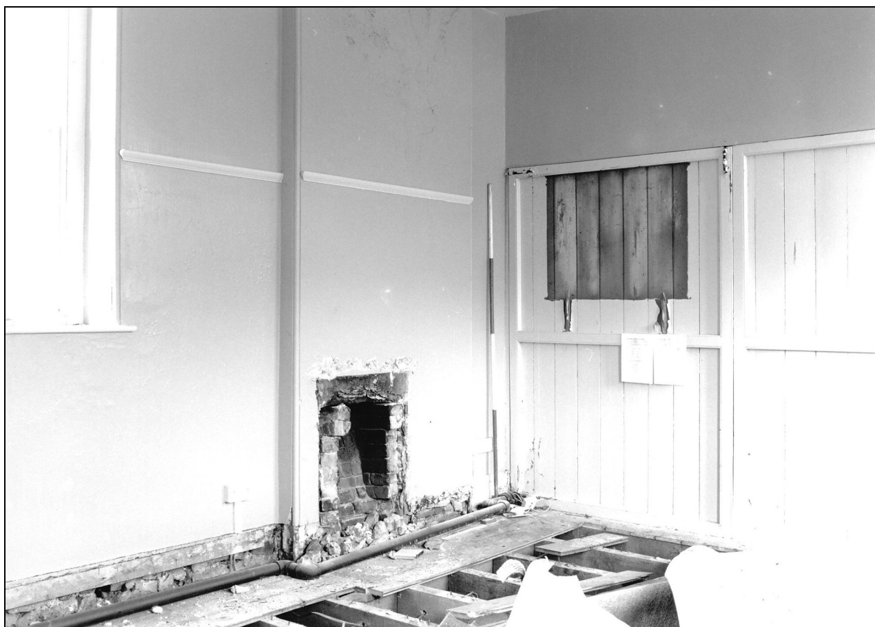
Photo 52: Interior of Sunday school: first floor classroom, from the south, showing remains of fireplace and movable partitions
